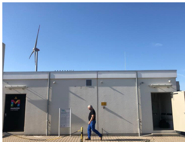
The gas blending building in Mainz, Germany, home to a 6 MW electrolyzer and direct hydrogen blending into the natural gas system
