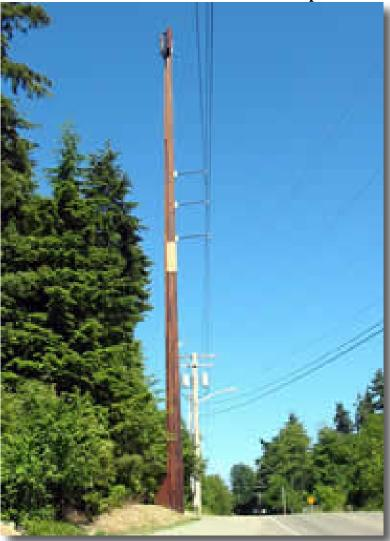
Note how much taller the pole is in the foreground compared to the one in the background to accommodate a wireless antenna.
