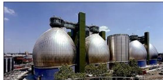
Anaerobic Digester Eggs at Newtown Creek
