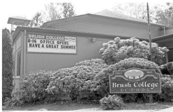
The original Brush College Elementary School was built in 1860. The current spot in West Salem is seen here in August 2017. ANNA REED/STATESMAN JOURNAL
