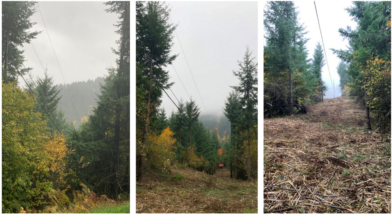
Figure 116: Mowing Mitigation (Heavily Vegetated Powerline Corridor), Pre and Post-Mitigation
