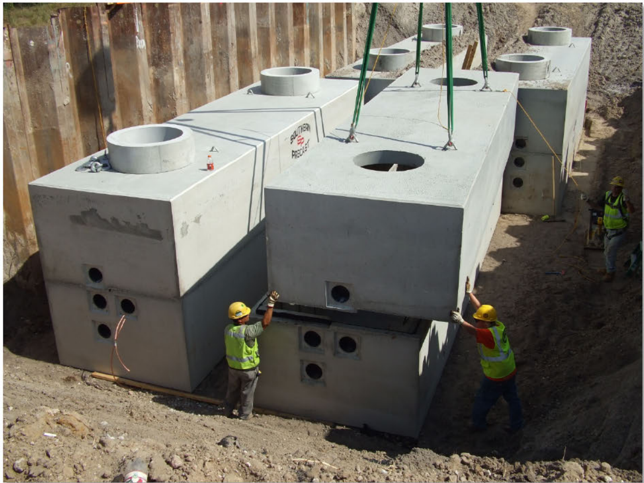
Figure 3: Typical Splicing Vault Installation (lower voltage example)
