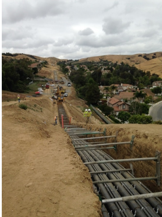
Figure 5: Typical Trench Excavation (Single Trench Only)
