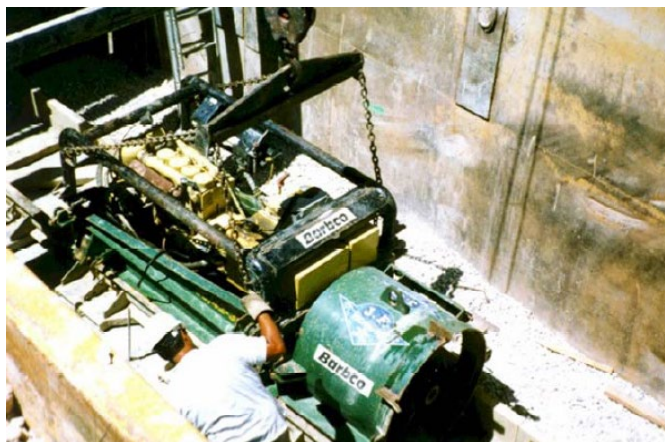
Figure 7: Typical J&B Setup (Lower Voltage Example)
