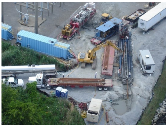
Figure 8: Typical HDD Setup (Lower Voltage Example)
