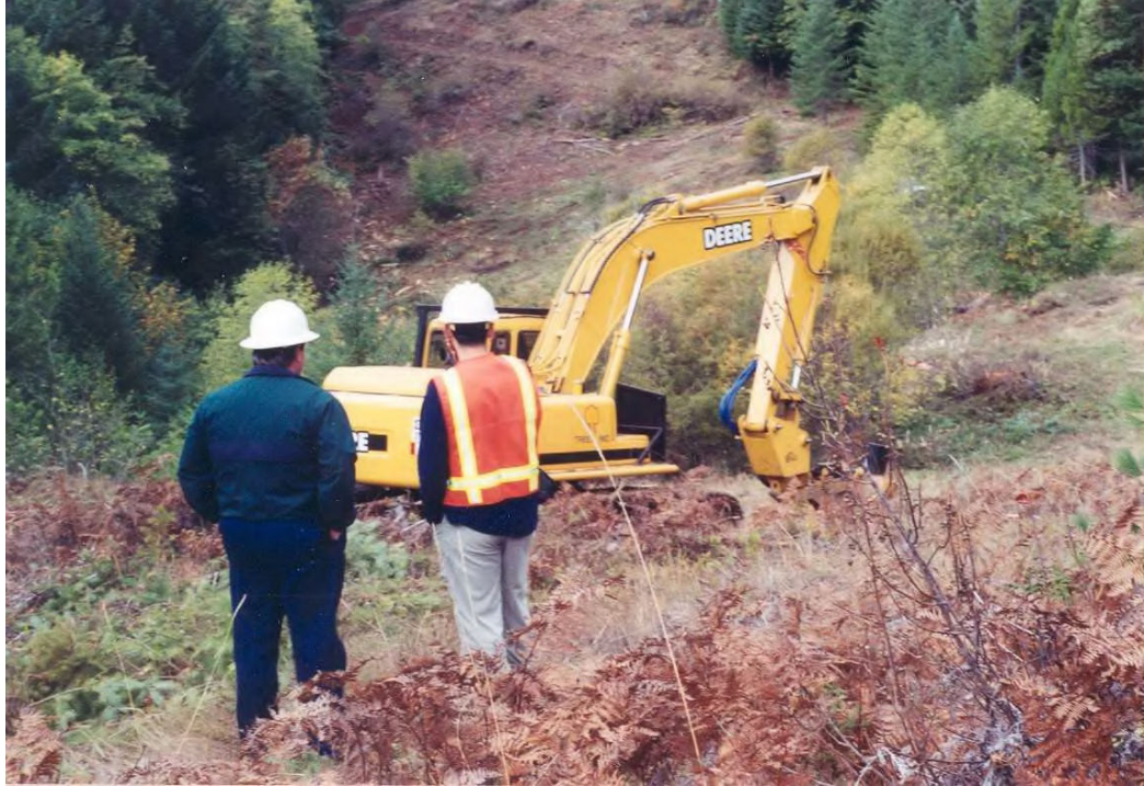
Figure 6.3. Right-of-way reclamation using mechanical control. In this case, a slashbuster.
