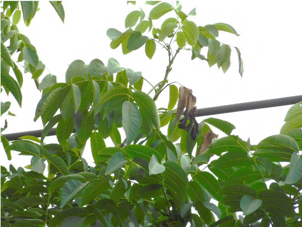
Probable violation B.119: Tree shows evidence of contacting primary conductors at 1180 Rosemont Road, West Linn. (45.3698, -122.6483)
