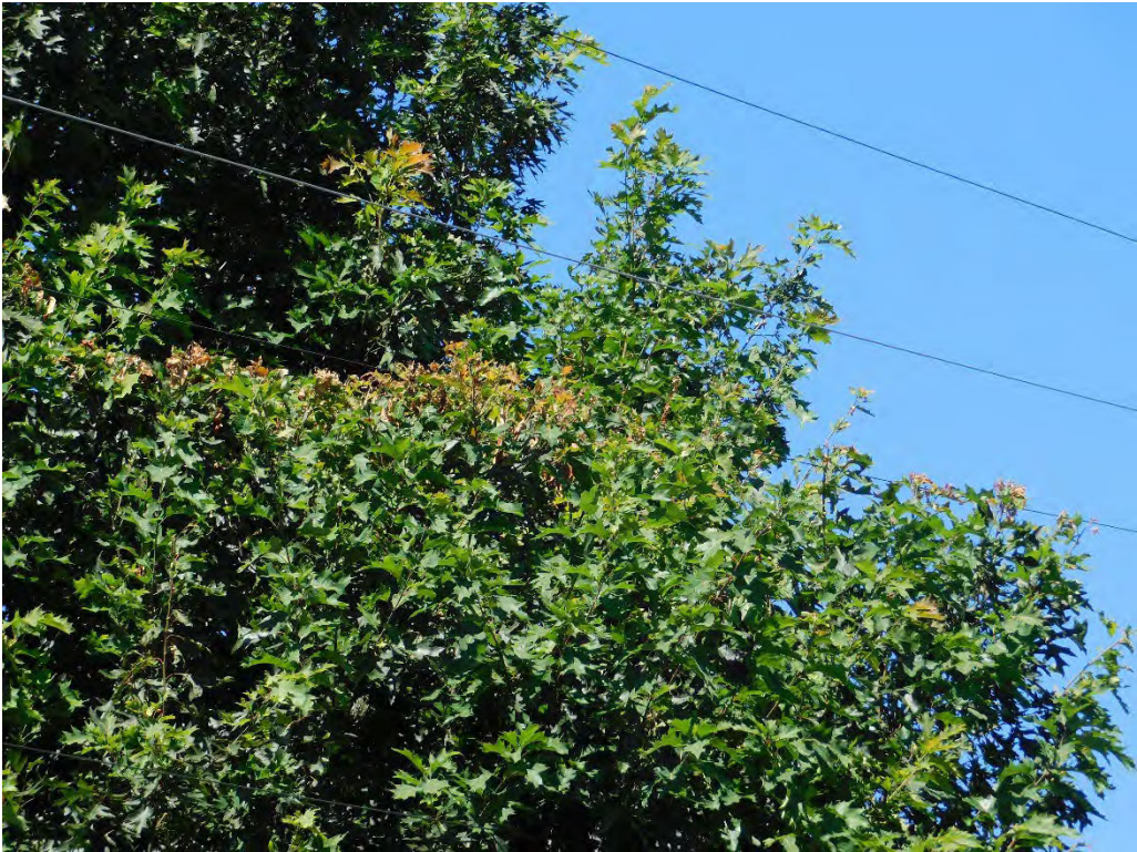
Probable violation B.146: Tree shows evidence of contacting primary conductors at 14325 SE River Road, Portland. (45.4188, -122.6457)
