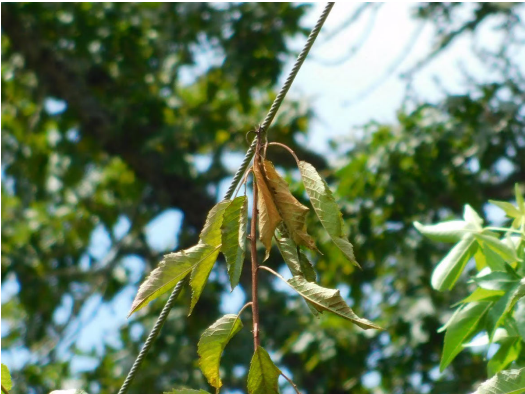
Probable violation B.16: Tree shows evidence of contacting primary conductors on Bruch College Road NW, Salem. (45.0125, -123.1292)
