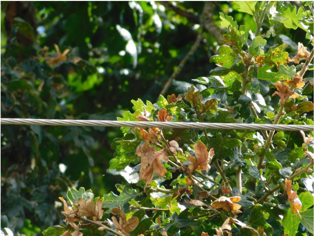
Probable violation B.17: Multiple trees show evidence of contacting the primary conductor on Spring Valley Road NW, Salem. (45.0354, -123.1182)
