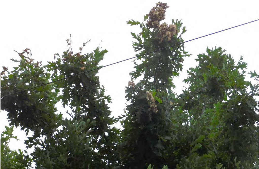
Probable violation B.185: Multiple trees show evidence of contacting the primary conductor at 10852 SE 7th Avenue, Portland. (45.4446, -122.5891)
