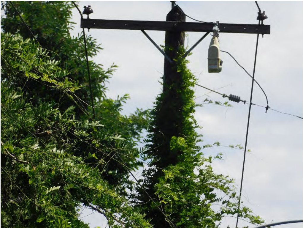
Probable violation C.5: Vines engulfing pole and approaching primary conductor are creating a hazard at the intersection of SE Aldercrest Court and SE Thiessen Road, Portland. (45.4162, -122.5992)
