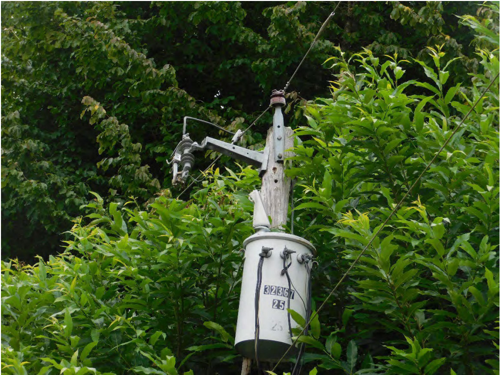
Probable violation B.117: Multiple trees show evidence of contacting the primary conductor at 2175 SW Borland Road, Tualatin. (45.3711, -122.6982)
