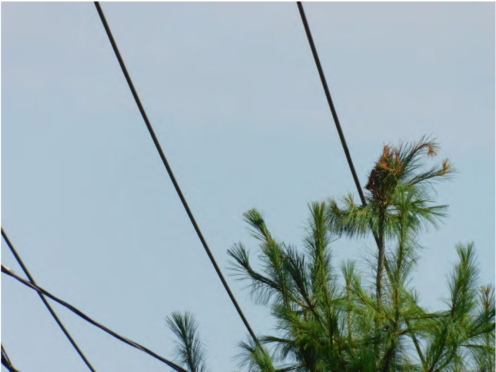
Probable violation B.266: Tree shows evidence of contacting primary conductors at 4128 Cordon Road NE, Salem. (44.9789, -122.9567)
