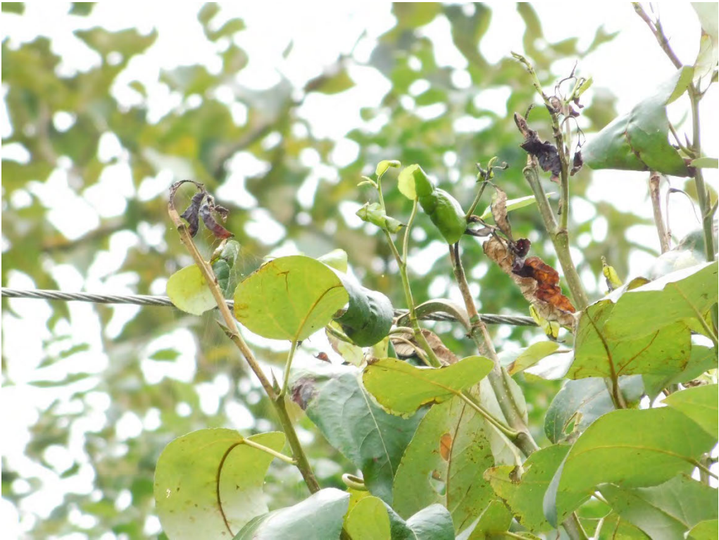
Probable violation B.245: Two trees show evidence of contacting the primary conductor on 4 th Avenue, West Linn. (45.3456, -122.6396)
