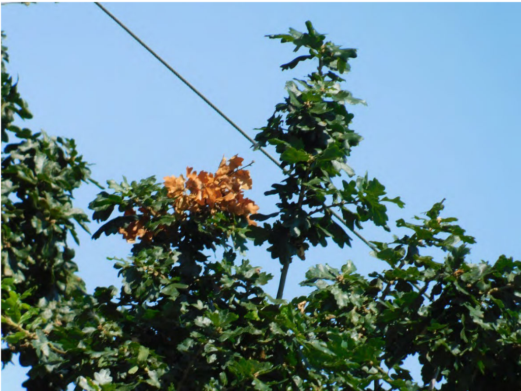
Probable violation B.255: Tree shows evidence of contacting primary conductors at 7472 Mill Creek Road SE, Aumsville. (44.8389, -122.9069)
