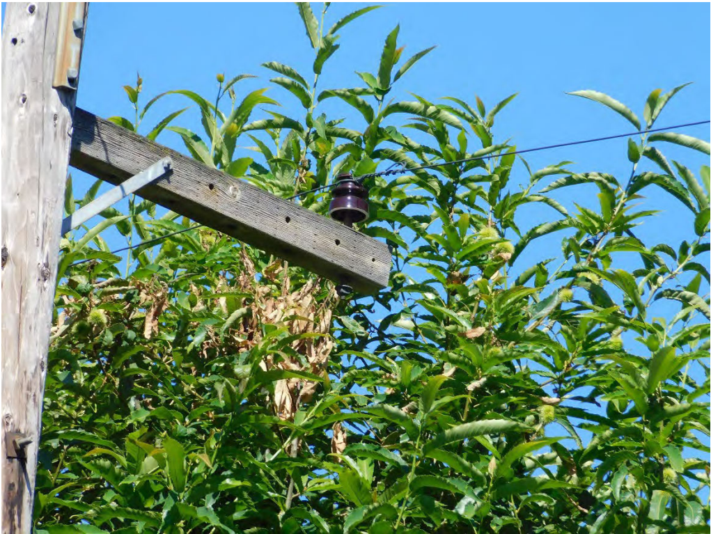
Probable violation B.129: Multiple trees show evidence of contacting the primary conductor at 4531 SE Jennings Avenue, Portland. (45.3905, -122.6158)
