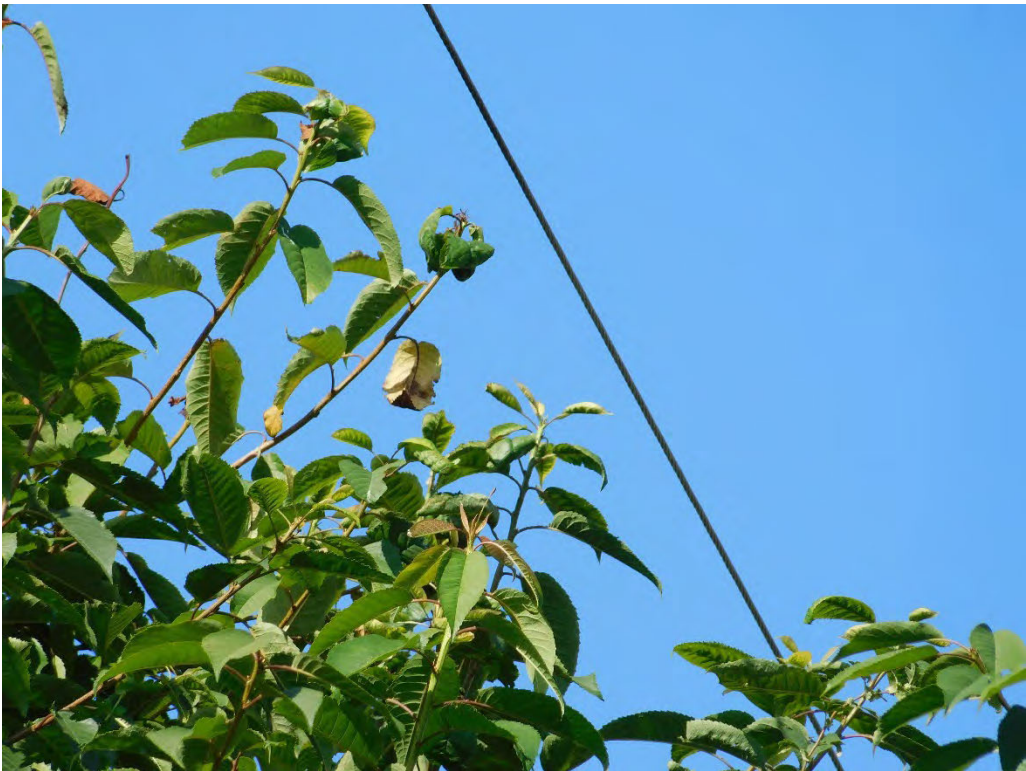
Probable violation B.285: Tree shows evidence of contacting primary conductors at 7256 Lakeside Drive NE, Salem. (45.0236, -122.9573)
