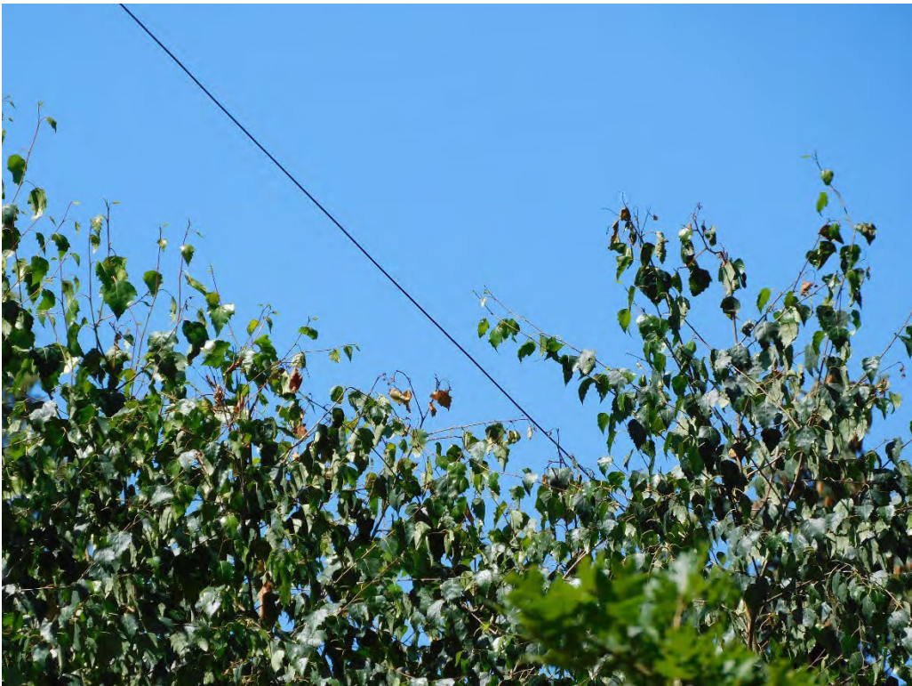
Probable violation B.51: Tree shows evidence of contacting primary conductors at 14510 NW Pioneer Road, Beaverton. (45.5214, -122.8262)
