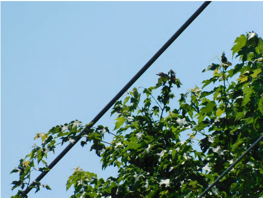
Probable violation A.14: Hazard: Multiple spans of readily climbable trees show evidence of contacting the primary conductor at 3790 Fisher Road NE, Salem. (44.9739, -122.9884)
