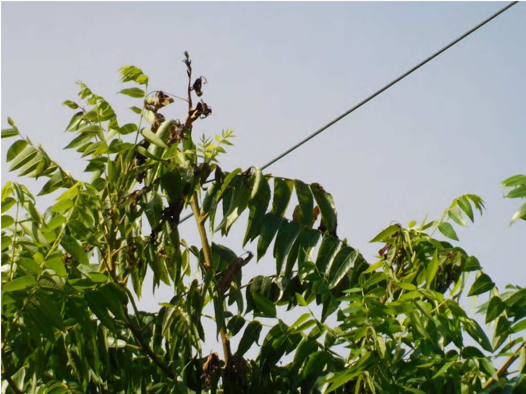
Probable violation B.283: Tree shows evidence of contacting primary conductors at 5995 Lake Labish Road, Salem. (45.0078, -122.9617)
