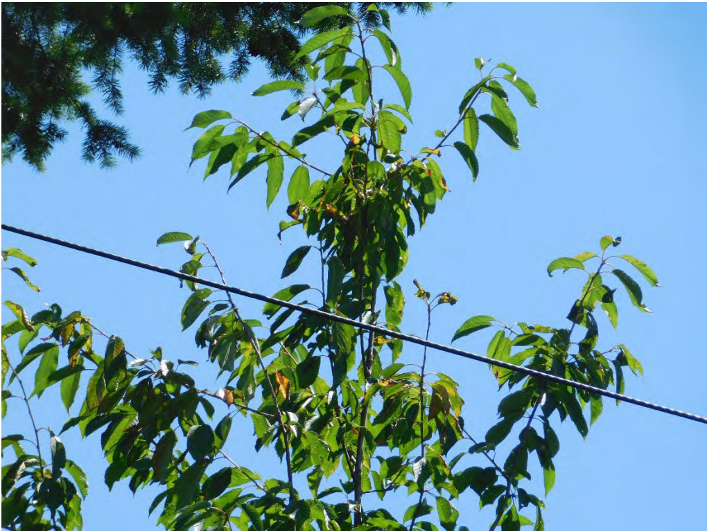
Probable violation B.320: Tree shows evidence of contacting primary conductors across from 28383 South Baurer Road, Colton. (45.1949, -122.4144)
