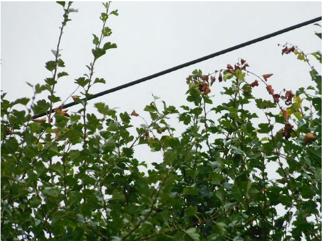
Probable violation B.200: Tree shows evidence of contacting primary conductors at 4180 SE Harvey Court, Portland. (45.4513, -122.6205)
