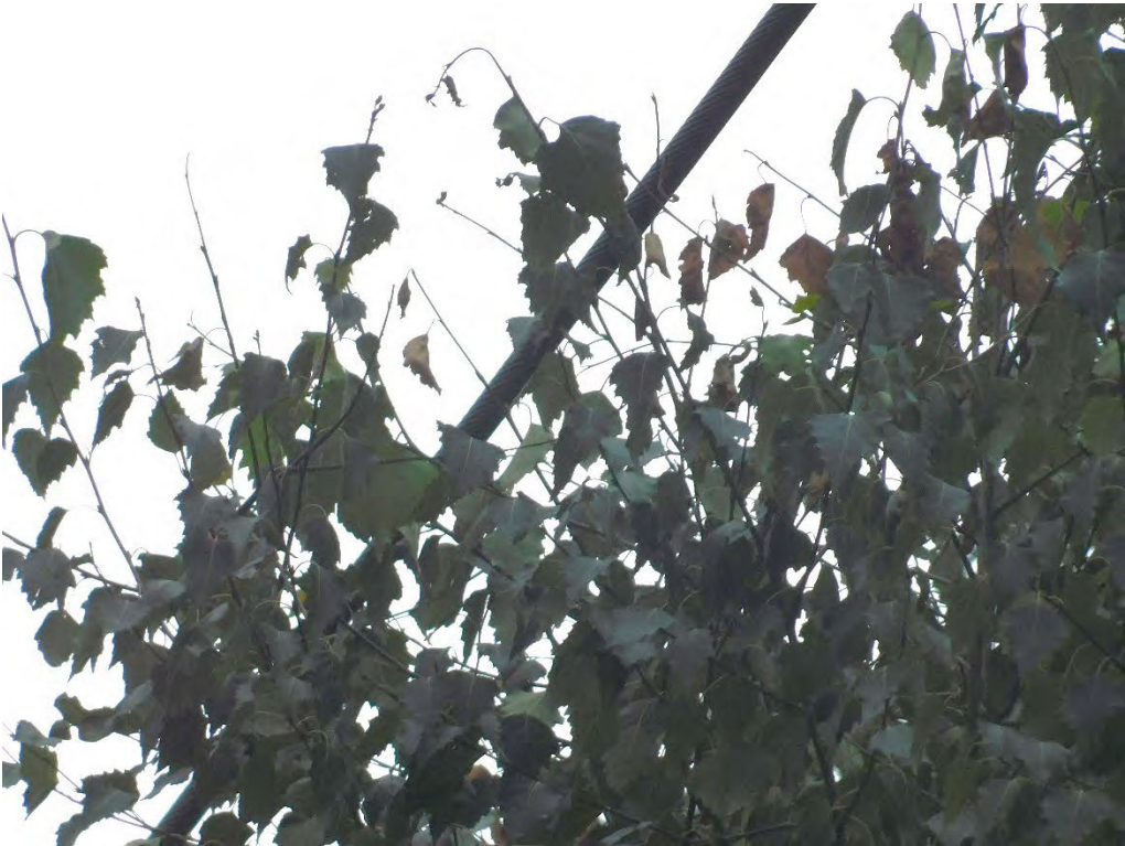
Probable violation B.203: Tree shows evidence of contacting primary conductors at 8607 SE 29 th Avenue, Portland. (45.4573, -122.6328)
