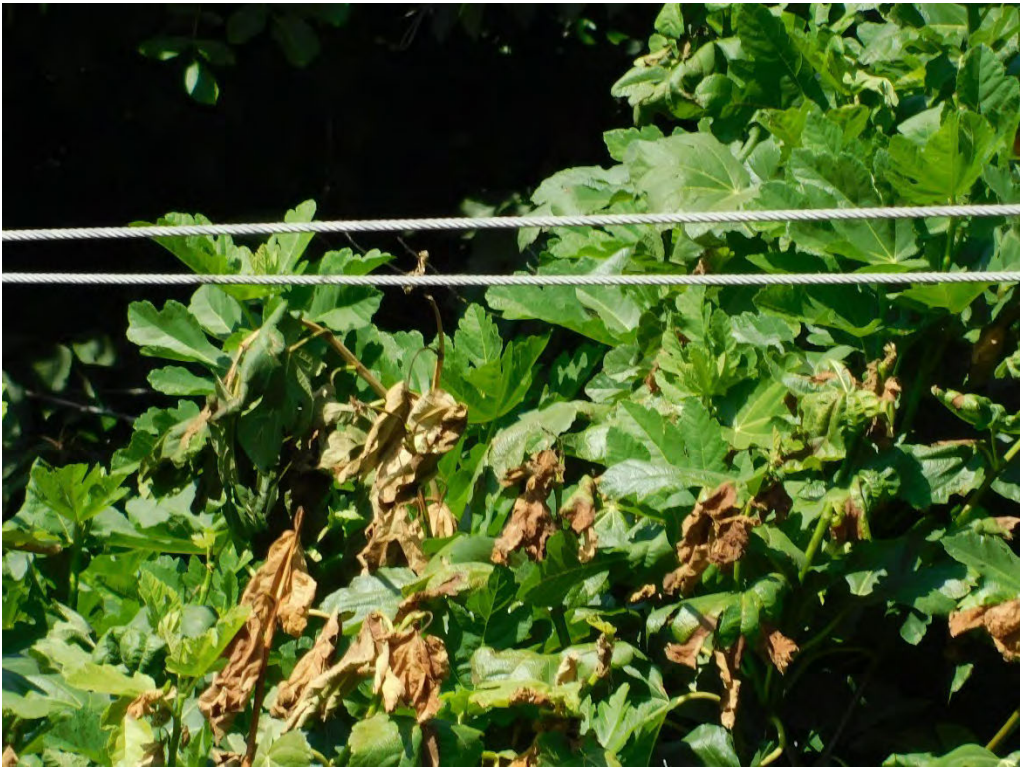
Probable violation B.19: Tree shows evidence of contacting primary conductors at 8275 Wheatland Road North, Keizer. (45.0389, -123.0177)
