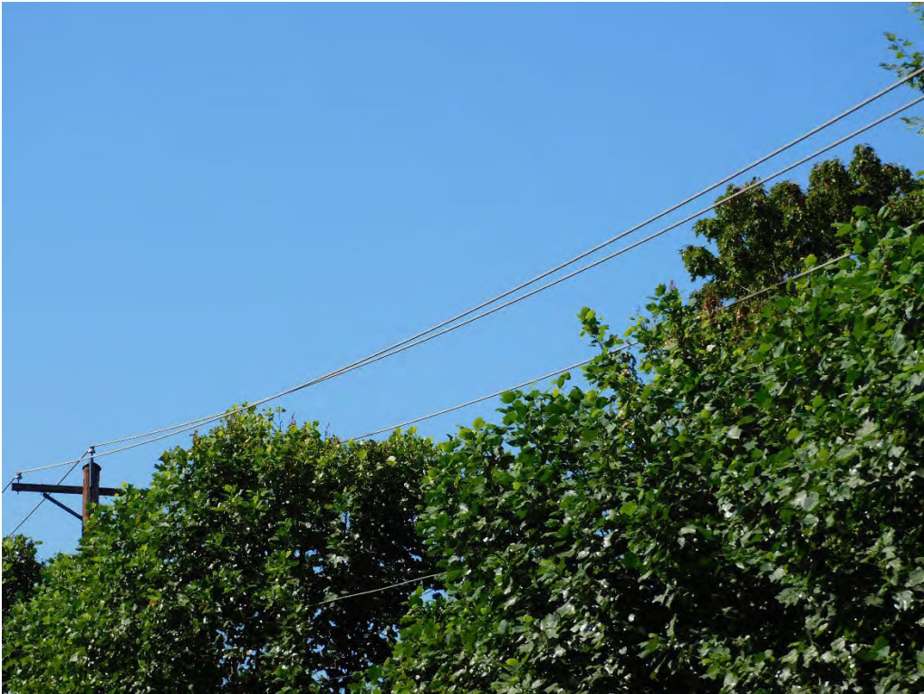
Probable violation B.46: Multiple trees show evidence of contacting the primary conductor on NE 15th Avenue, Hillsboro. (45.5402, -122.9663)
