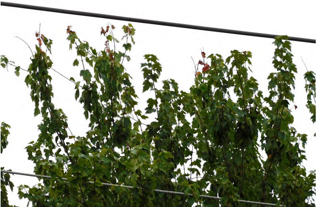
Probable violation B.368: Tree shows evidence of contacting primary conductors at 12155 SE Harold Street, Portland. (45.4833, -122.5383)
