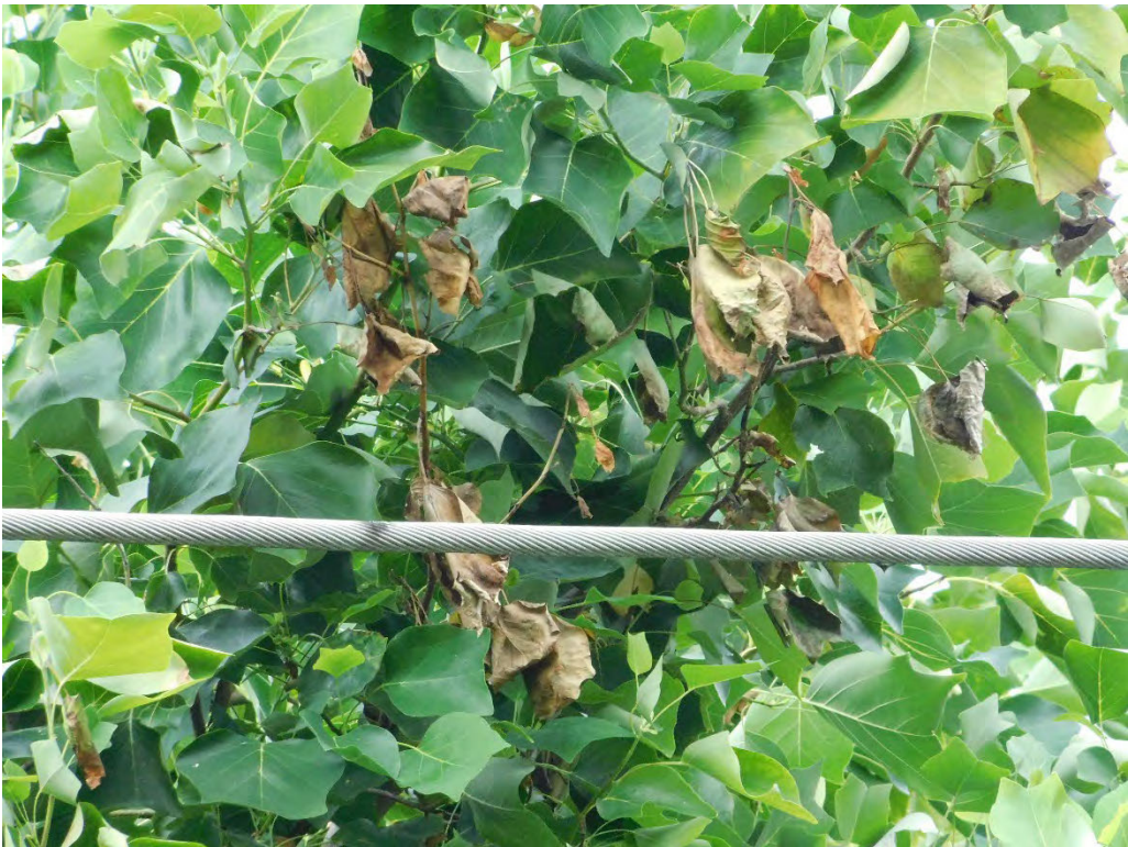
Probable violation B.240: Two trees show evidence of contacting the primary conductor at 1208 SW Willamette Falls Drive, West Linn. (45.3439, -122.6651)
