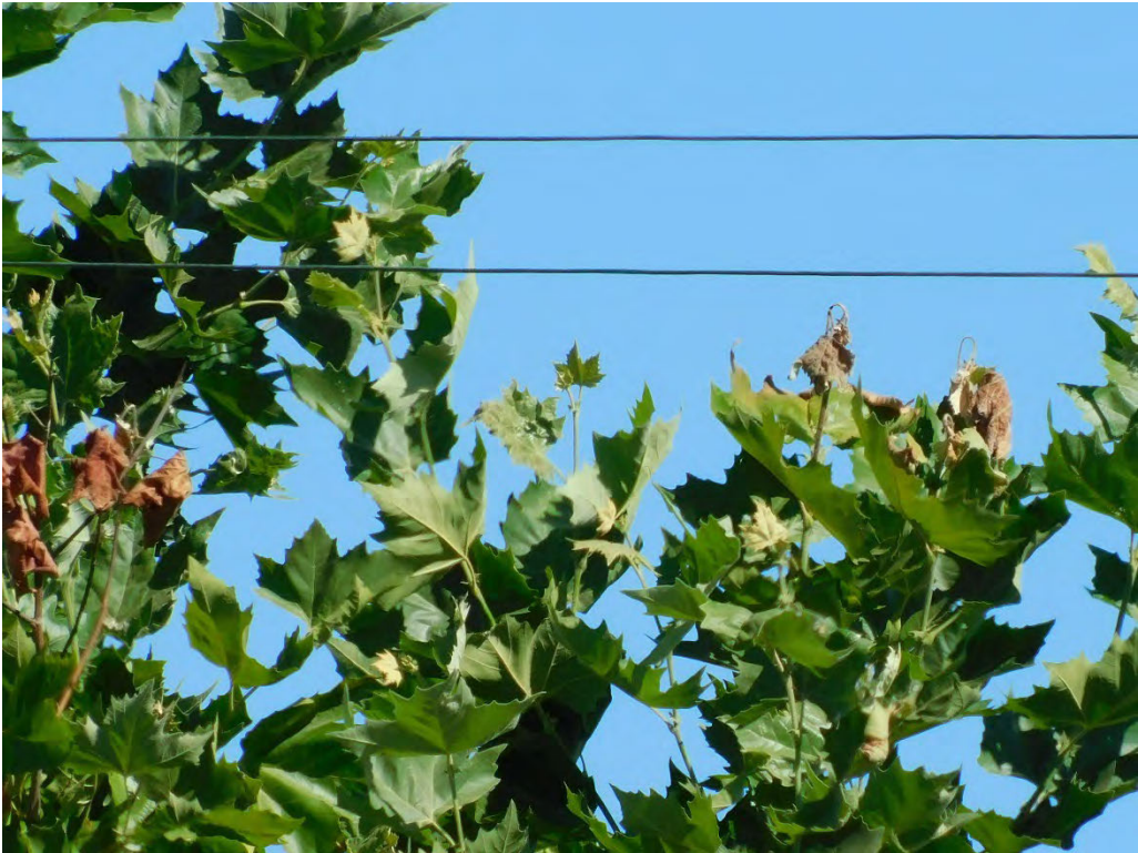
Probable violation B.20: Tree shows evidence of contacting primary conductors on Donald Road NE, Donald. (45.2207, -122.8311)
