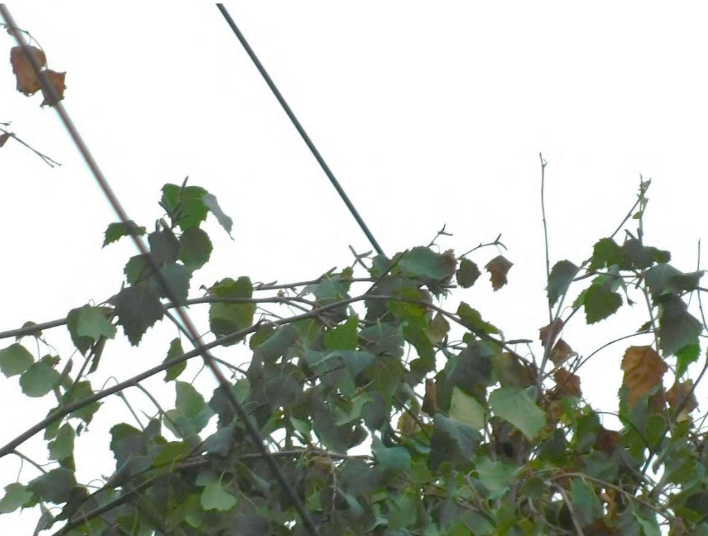
Probable violation B.93: Tree shows evidence of contacting primary conductors at 10112 SW 55 th Avenue, Portland. (45.4524, -122.7333)
