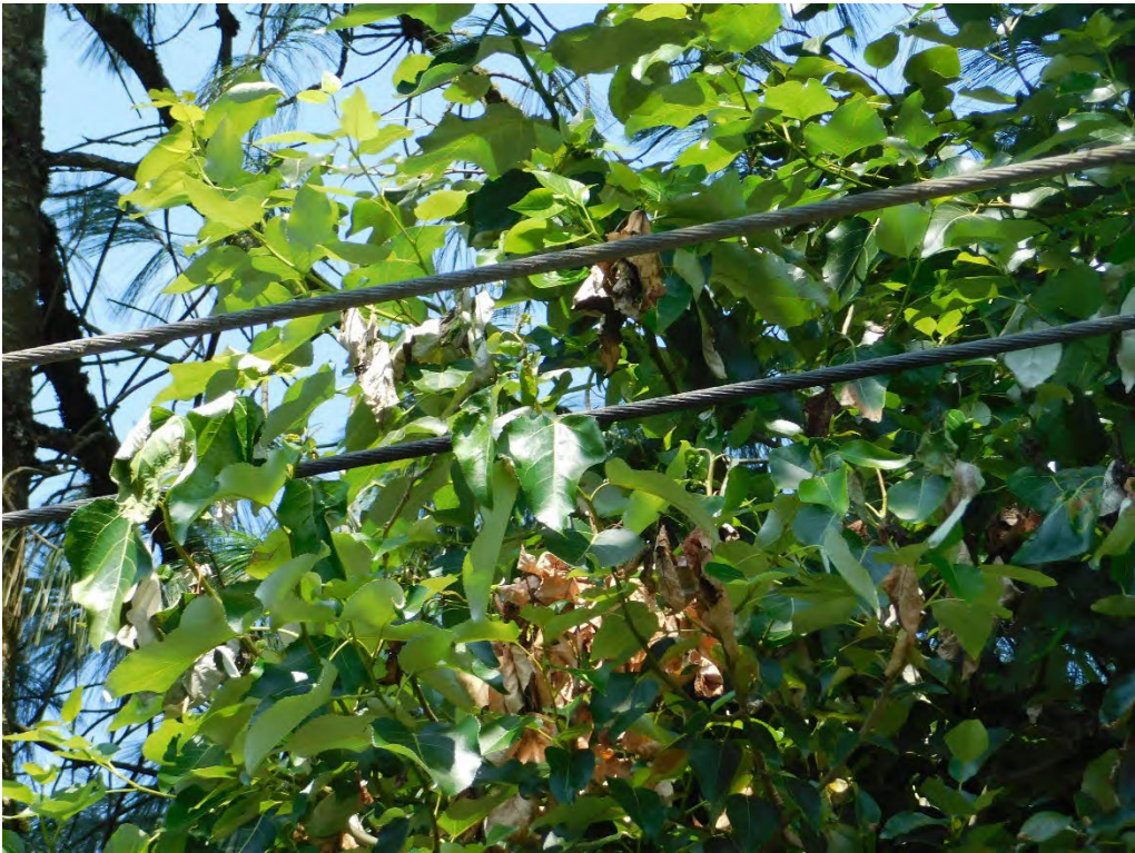
Probable violation B.167: Tree shows evidence of contacting primary conductors at the intersection of SE Aldercrest Road and SE Thiessen Road, Portland. (45.4163, -122.6000)
