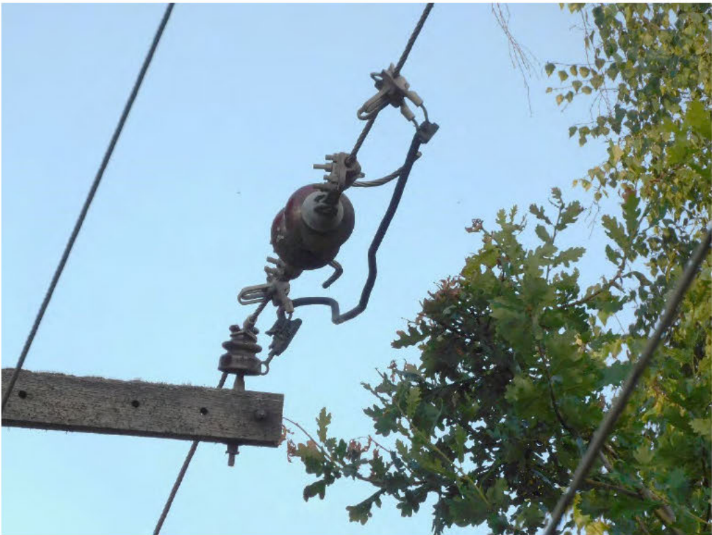
Probable violation B.330: Tree shows evidence of contacting primary conductors at the intersection of South Bremer Road and South Haines Road, Canby. (45.2711, -122.6613)
