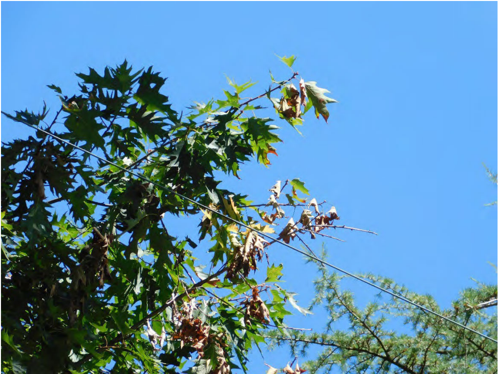
Probable violation B.143 Multiple trees show evidence of contacting the primary conductor at 2611 SE Tarbell Avenue, Portland. (45.4047, -122.6371)
