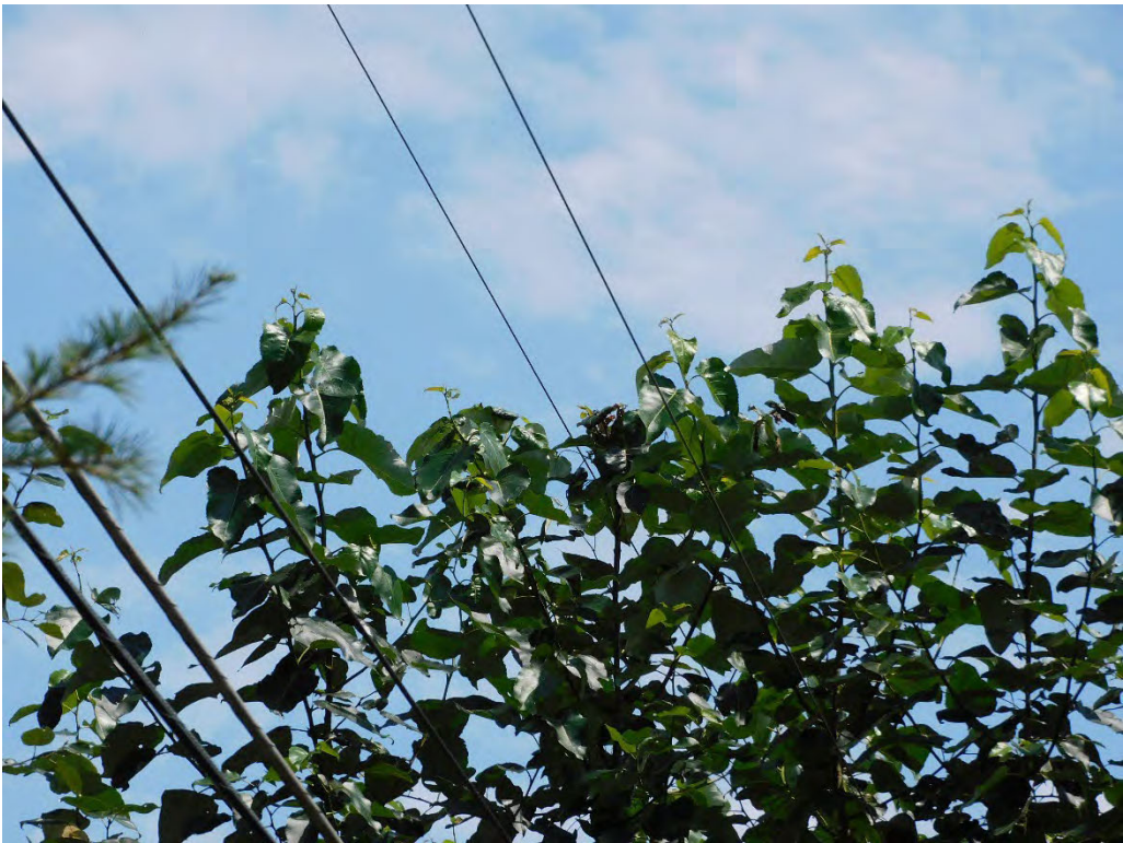
Probable violation B.334: Tree shows evidence of contacting primary conductors at 15199 South Maplelane Road, Oregon City. (45.3378, -122.5545)
