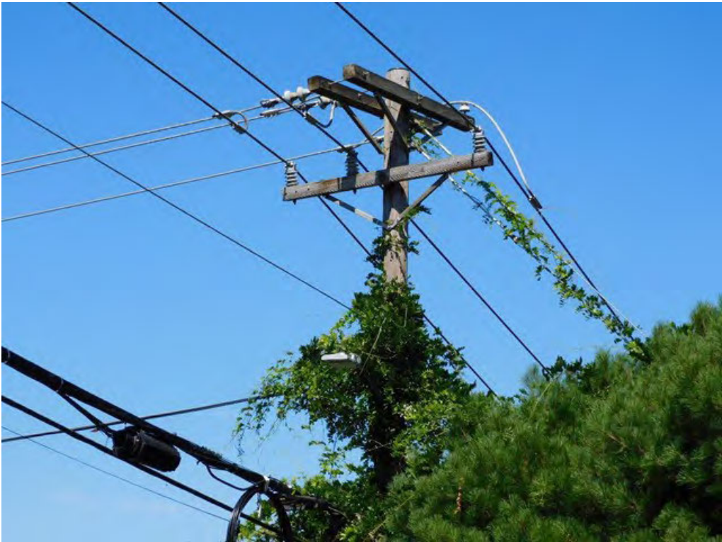
Probable violation C.17: Vines engulfing pole and approaching primary conductor are creating a hazard at 247 SE 4th Street, Troutdale. (45.5387, -122.3864)
