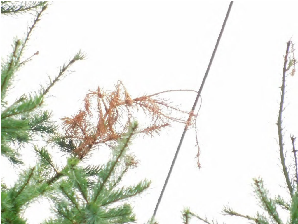
Probable violation B.243: Tree shows evidence of contacting primary conductors at 1315 Dollar Street, West Linn. (45.3460, -122.6630)
