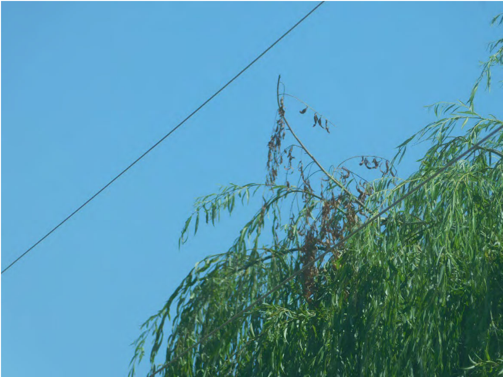
Probable violation B.307: Two trees show evidence of contacting primary conductors at 6098 Topaz Street NE, Salem. (45.0620, -122.9364)
