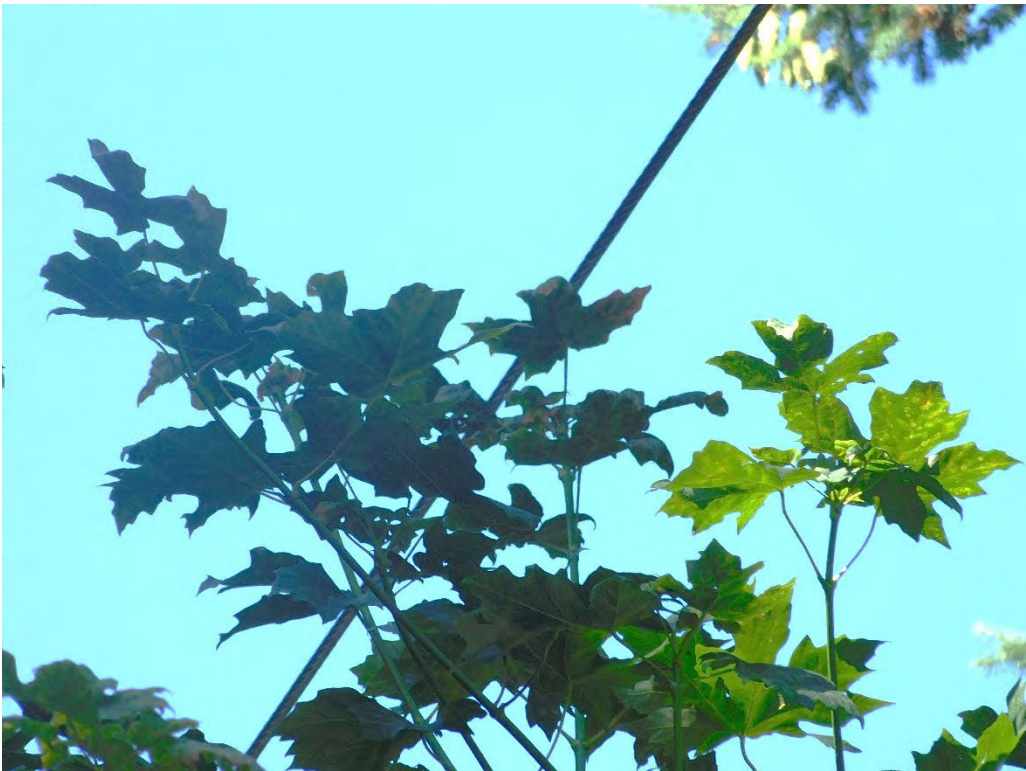
Probable violation B.55: Tree shows evidence of contacting primary conductors at 3149 SE Fairview Blvd., Portland. (45.5194, -122.7146)
