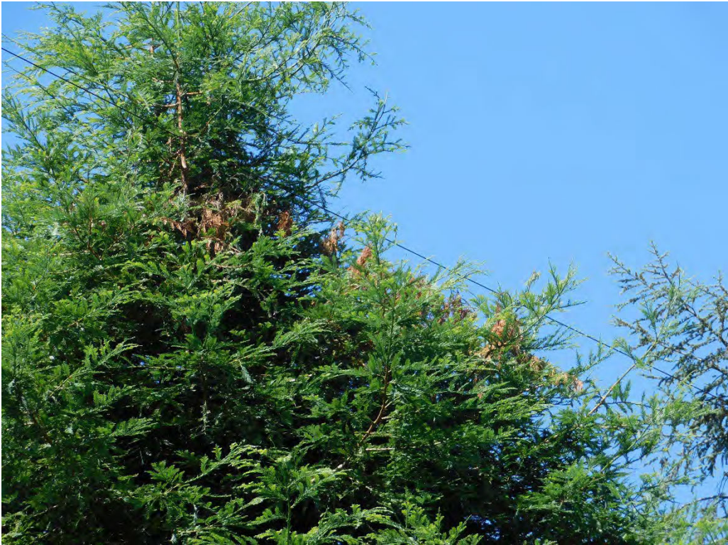
Probable violation B.144: Multiple trees show evidence of contacting the primary conductor at 16205 SE River Road, Portland. (45.4056, -122.6405)
