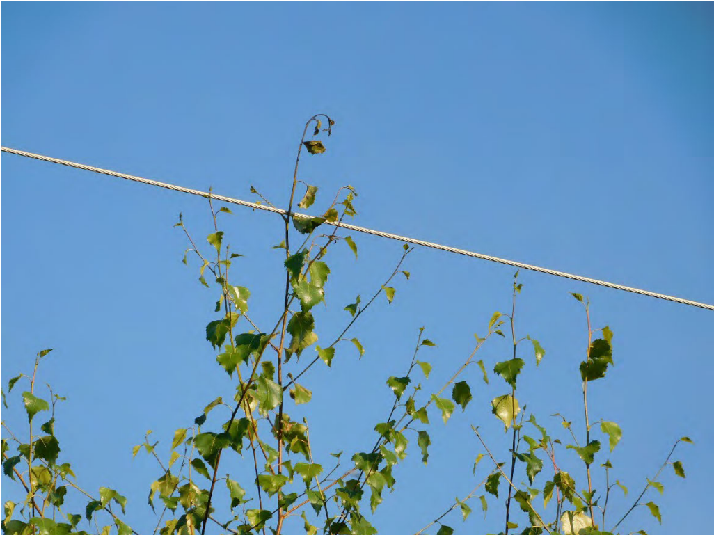
Probable violation B.342: Tree shows evidence of contacting primary conductors at 16268 South Babler Road, Oregon City. (45.3710, -122.4539)
