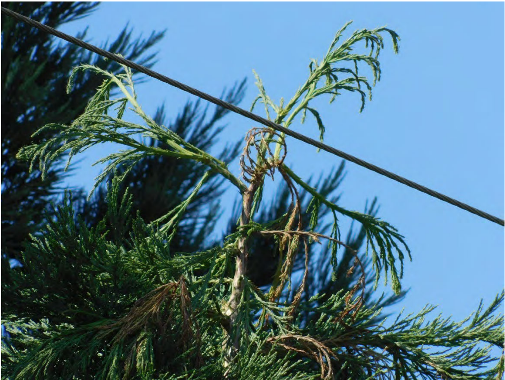
Probable violation B.252: Tree shows evidence of contacting primary conductors at 6724 Mill Creek Road SE, Turner. (44.8387, -122.9233)
