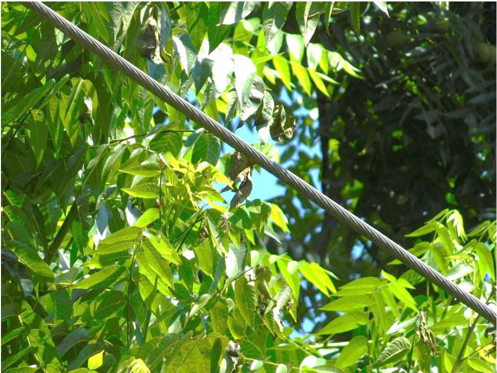
Probable violation B.169: Tree shows evidence of contacting primary conductors at 6593 SE Thiessen Road, Portland. (45.4162, -122.5962)
