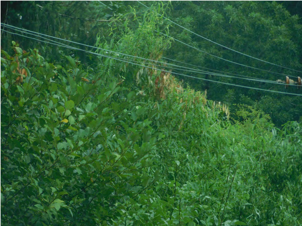
Probable violation B.97: Multiple trees show evidence of contacting the primary conductor at the intersection of SW 62nd Drive and SW Huddleson Street, Portland. (45.4491, -122.7385)
