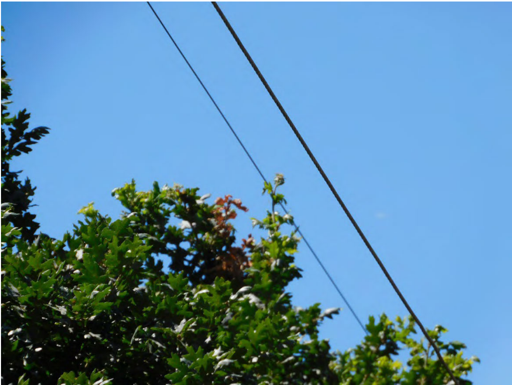
Probable violation B.34: Tree shows evidence of contacting primary conductors on SW Laurelwood Road, Gaston. (45.4248, -123.0896)
