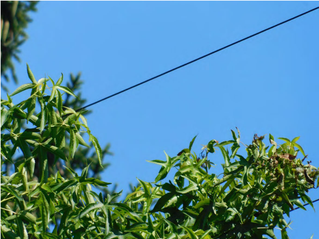
Probable violation B.220: Tree shows evidence of contacting primary conductors at 6136 SE 46 th Avenue, Portland. (45.4778, -122.6153)
