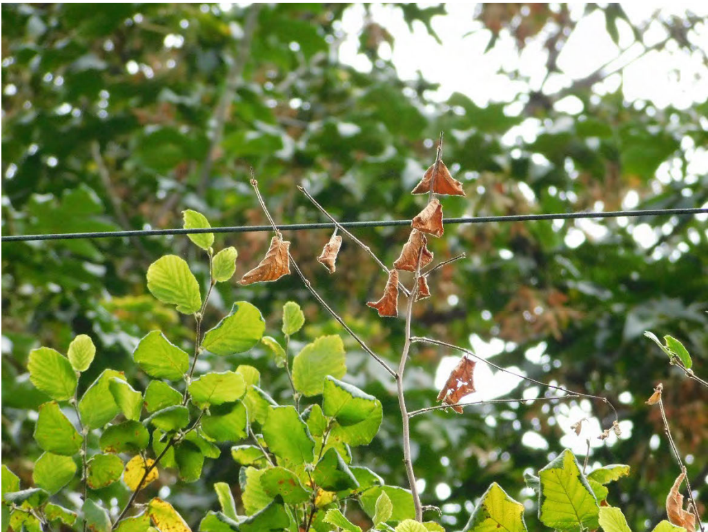
Probable violation B.238: Two trees show evidence of contacting the primary conductor on SW Turner Road, West Linn. (45.3586, -122.6936)
