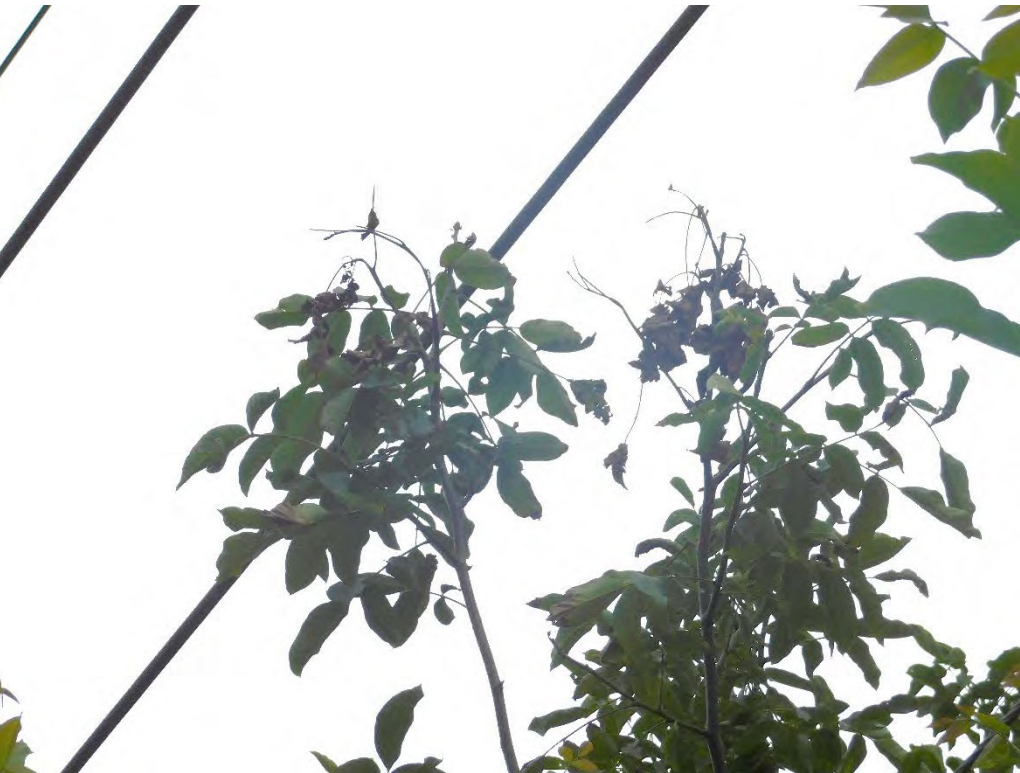
Probable violation B.204: Multiple trees show evidence of contacting the primary conductor at 9029 SE 29 th Avenue, Portland. (45.4552, -122.6327)
