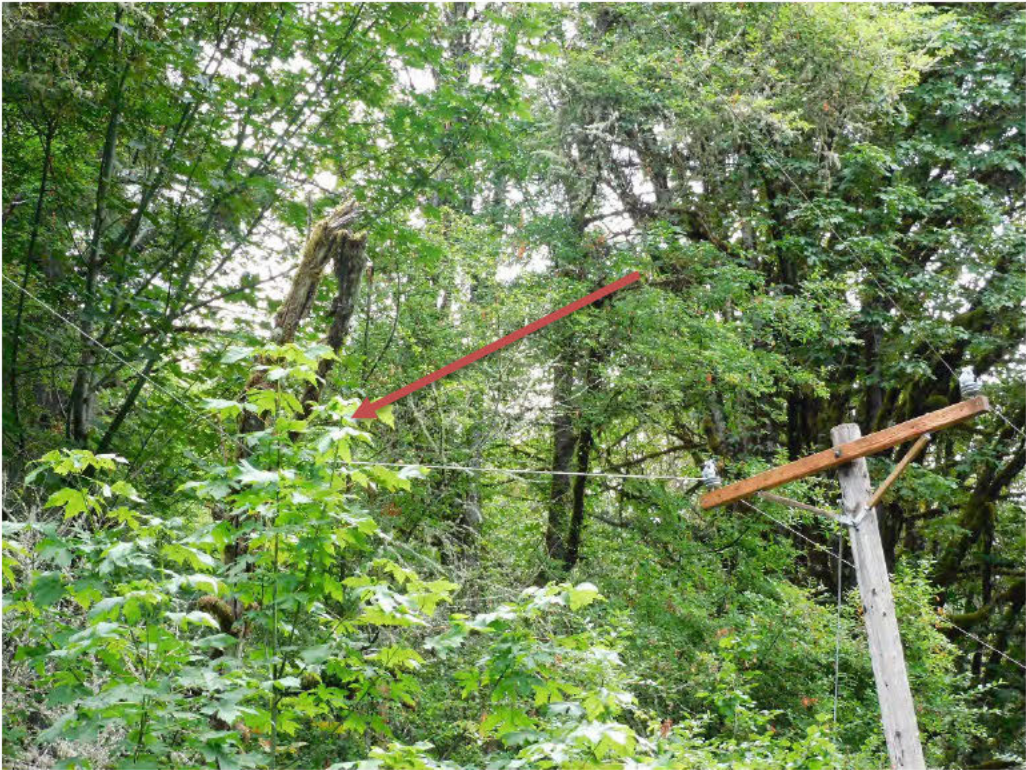
Probable violation D.1: Conductor energized below 600 volts is under strain or abrasion from vegetation on NW Davidson Road, Banks. (45.6326, -123.0755)
