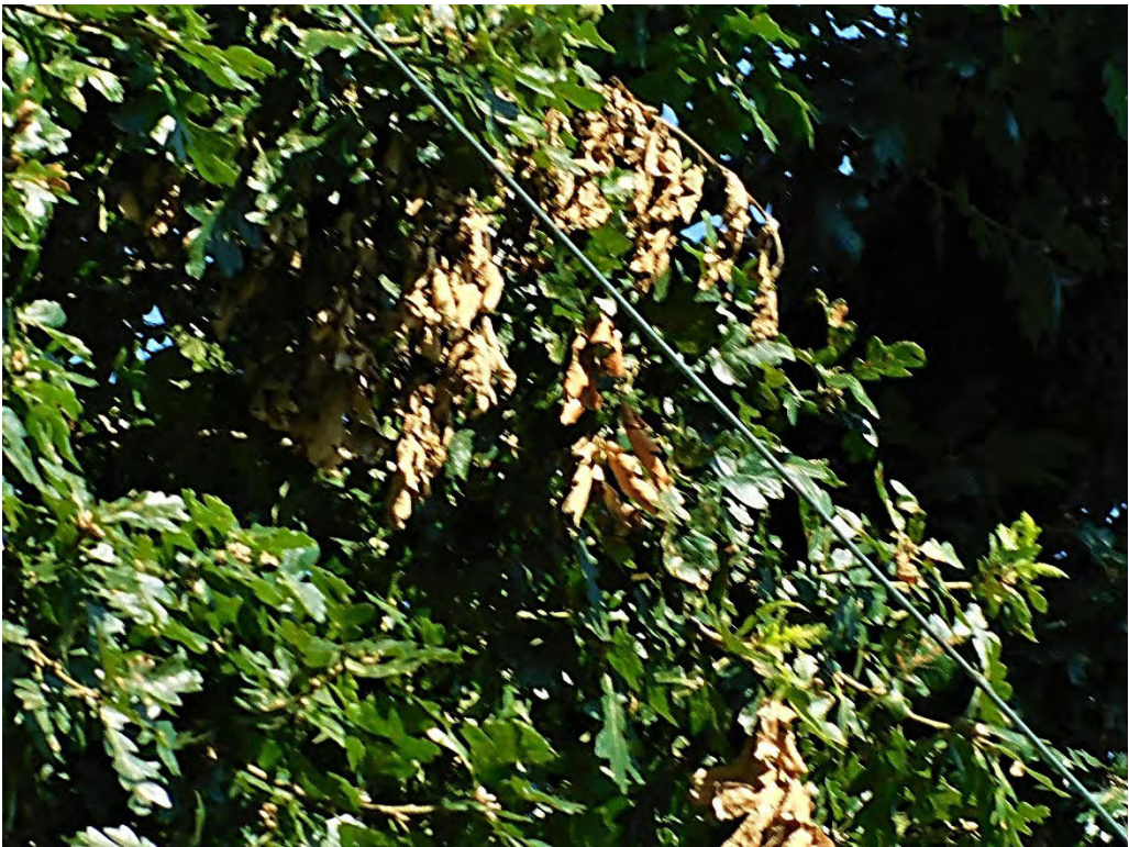
Probable violation B.251: Tree shows evidence of contacting primary conductors at 5255 Boise Street SE, Turner. (44.8436, -122.9522)
