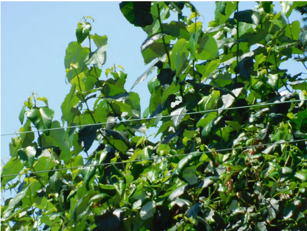
Probable violation B.303: Tree shows evidence of contacting primary conductors at 25393 Pacific Highway East, Aurora. (45.2392, -122.7370)
