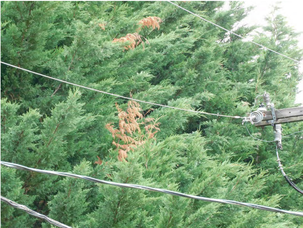
Probable violation B.379: Tree shows evidence of contacting primary conductors at 8690 SE 140 th Place, Happy Valley. (45.4600, -122.5197)
