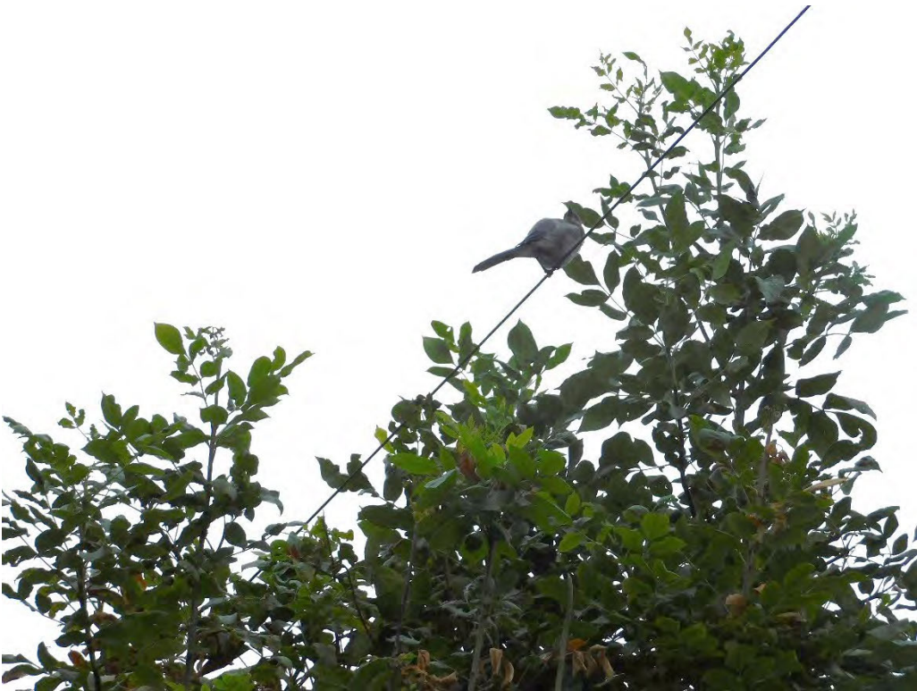
Probable violation B.180: Tree shows evidence of contacting primary conductors at 8010 SE McBride Street, Portland. (45.4358, -122.5814)
