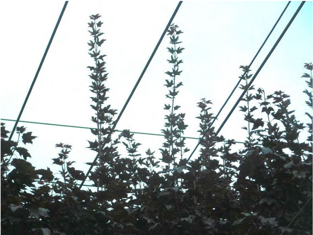
Probable violation B.199: Two trees show evidence of contacting the primary conductor at 9922 SE 37 th Avenue, Portland. (45.4511, -122.6247)
