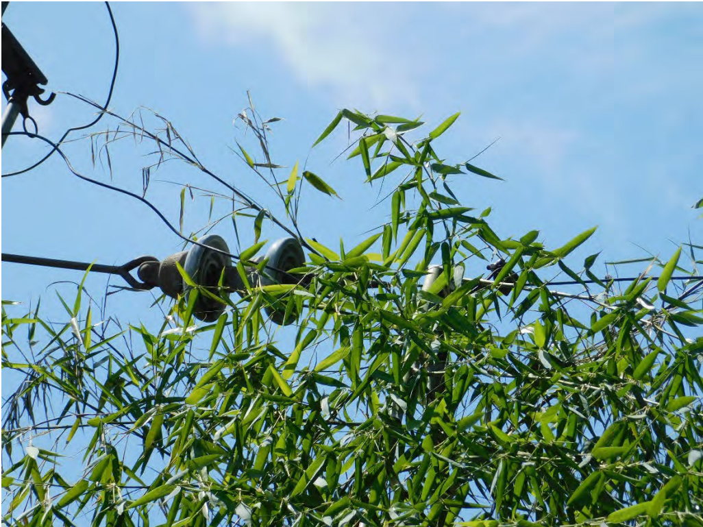
Probable violation B.170: Multiple trees show evidence of contacting the primary conductor at 16060 SE Brenda Avenue, Portland. (45.4066, -122.5849)
