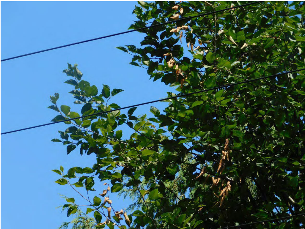
Probable violation B.85: Tree shows evidence of contacting primary conductors at 13941 Northwest Glendoveer Drive, Portland. (45.5960, -122.8217)
