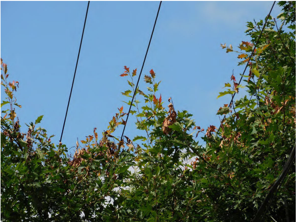
Probable violation B.335: Two trees show evidence of contacting primary conductors on South Maplelane Road, Oregon City. (45.3371, -122.5619)
