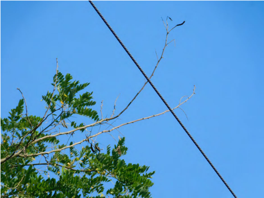
Probable violation B.249: Tree shows evidence of contacting primary conductors at 7715 5 th Street SE, Turner. (44.8434, -122.9560)
