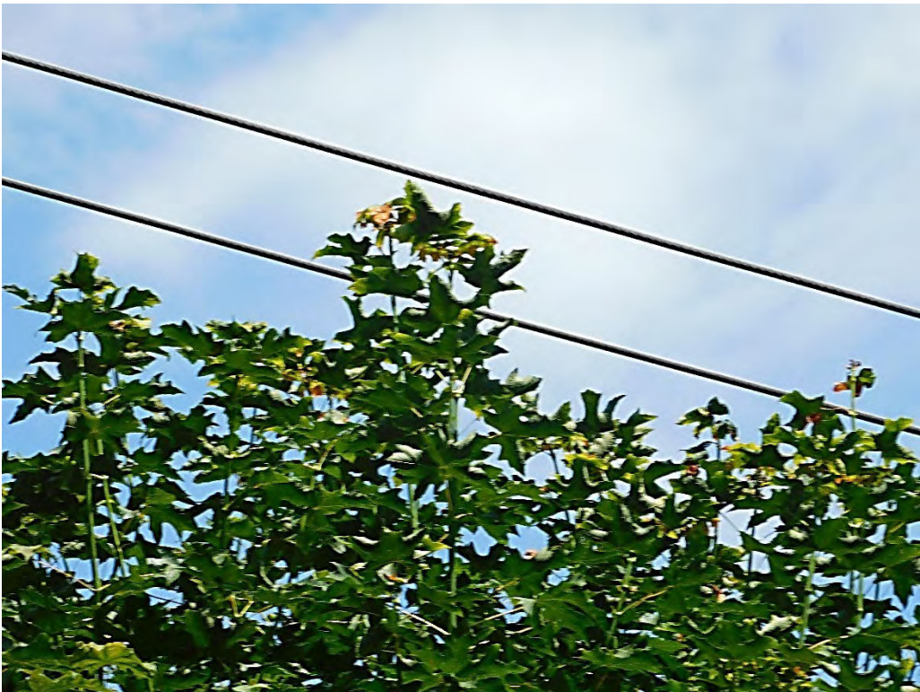
Probable violation B.166: Multiple trees show evidence of contacting the primary conductor across from 5904 SE Thiessen Road, Portland. (45.4162, -122.6022)
