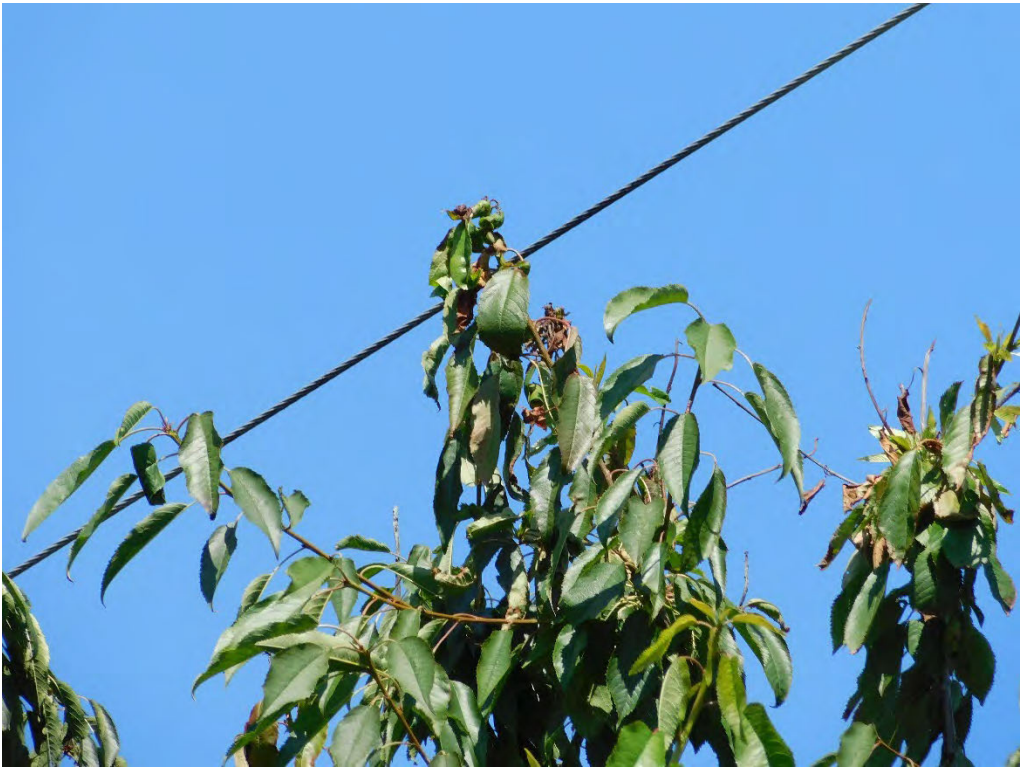
Probable violation A.13: Hazard: Readily climbable tree shows evidence of contacting the primary conductor at 7708 Sunnybrook Lane SE, Salem. (44.8437, -122.9042)
