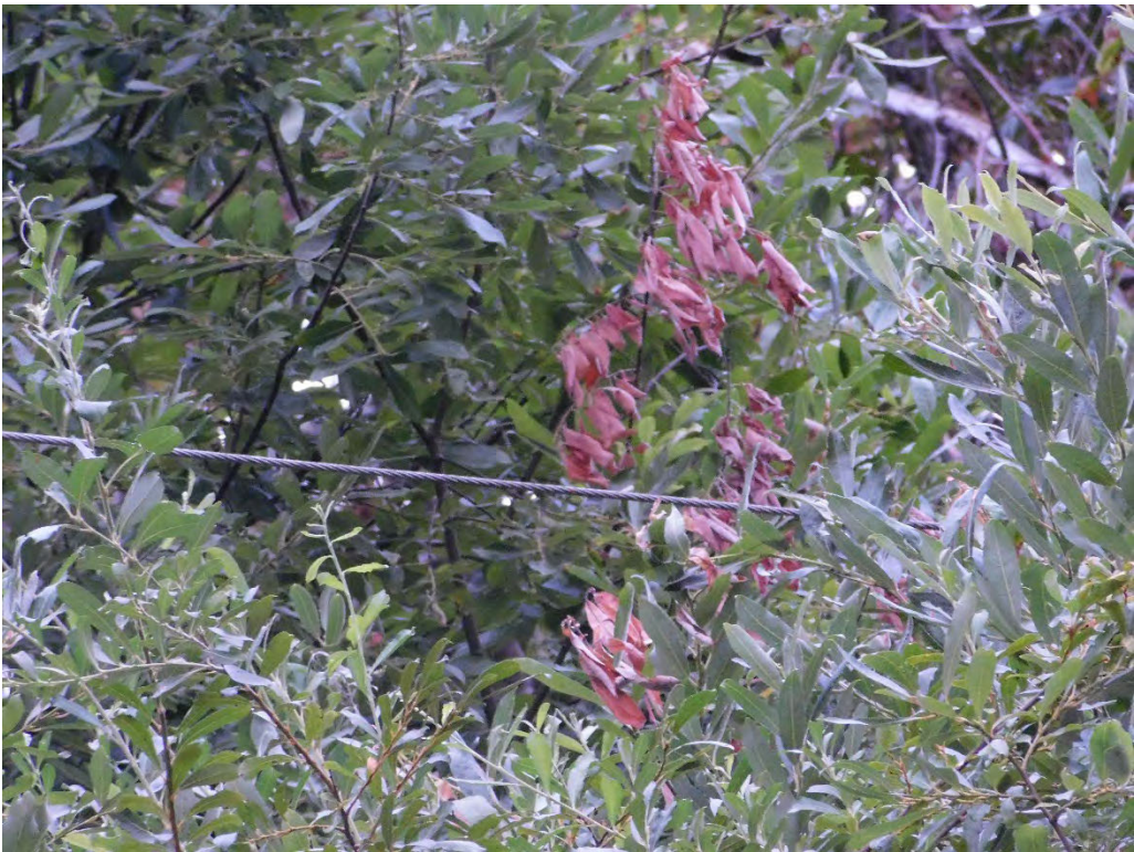
Probable violation B.24: Tree shows evidence of contacting primary conductors at 29560 NW Olson Road, Gaston. (45.4301, -123.1529)
