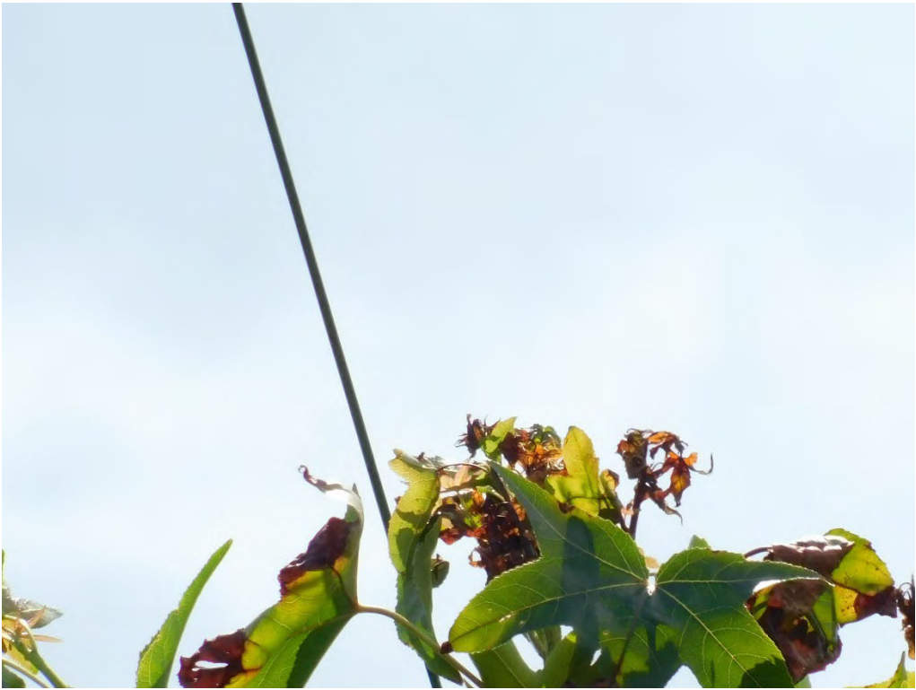
Probable violation B.11: Tree shows evidence of contacting primary conductors at 695 15 th Street NE, Salem. (44.9426, -123.0196)
