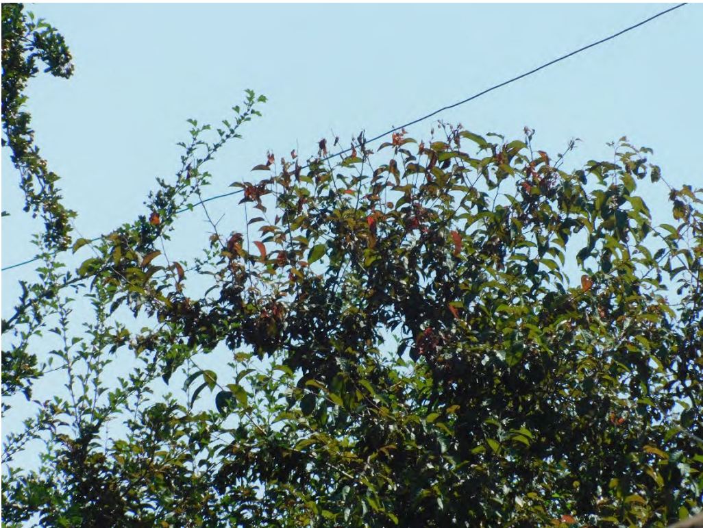
Probable violation B.218: Multiple trees show evidence of contacting the primary conductor behind 5218 SE Tolman Street, Portland. (45.4770, -122.6078)
