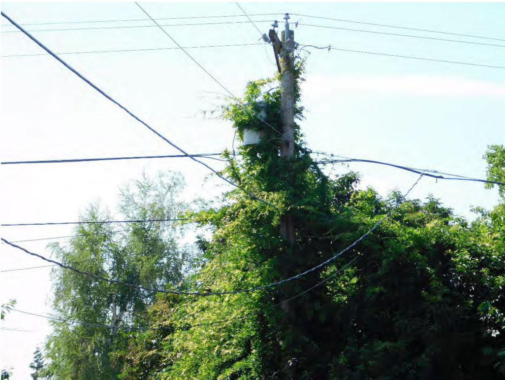
Probable violation C.8: Vines engulfing pole and approaching primary conductor are creating a hazard at 1356 Meadowlark Drive, Keizer. (45.0122, -123.0149)
