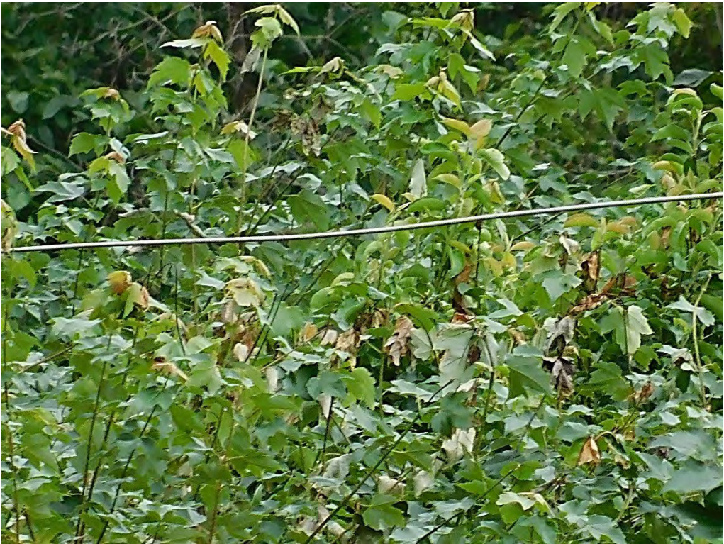
Probable violation B.15: Multiple trees show evidence of contacting the primary conductor on Gibson Road NW, Salem. (44.9813, -123.1039)
