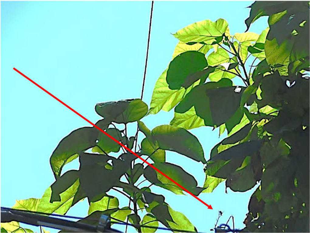
Probable violation B.141: Multiple trees show evidence of contacting the primary conductor at the intersection of SE River Road and SE Vineyard Way, Portland. (45.4011, -122.6334)
