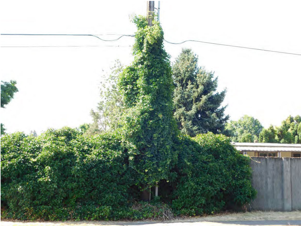
Probable violation C.7: Vines engulfing pole are creating a climbing hazard on Lockhaven Drive North, Keizer. (45.0044, -123.0278)
