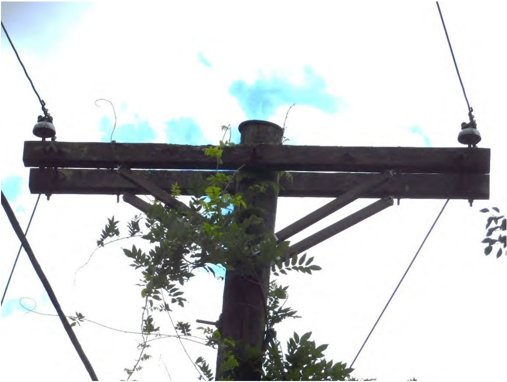
Probable violation C.3: Vines engulfing pole are creating a climbing hazard at 2796 Glen Haven Road, Lake Oswego. (45.4031, -122.7064)
