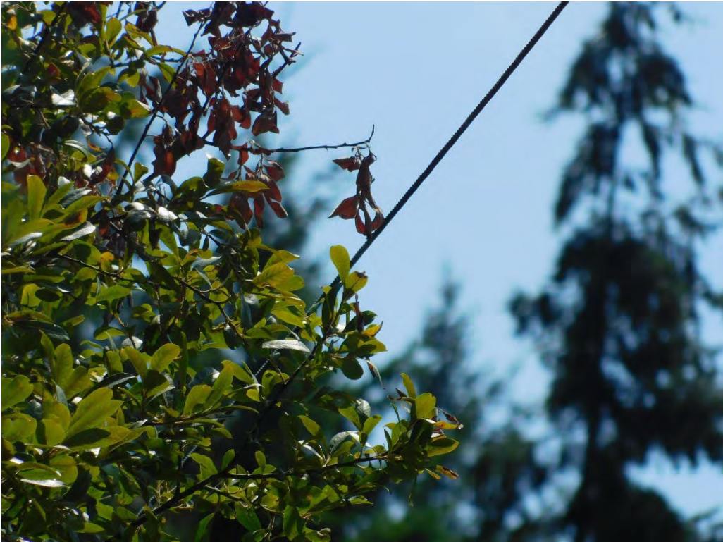
Probable violation B.87: Tree shows evidence of contacting primary conductors across from 12615 NW Skyline Blvd., Portland. (45.6145, -122.8667) HFRZ
