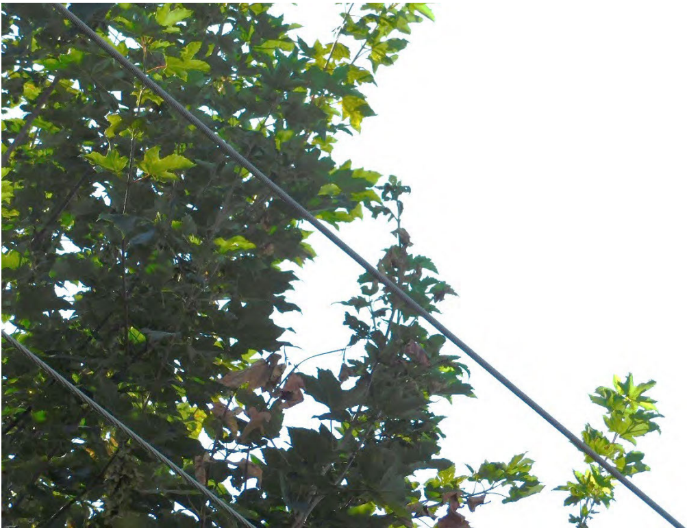
Probable violation B.263: Tree shows evidence of contacting primary conductors at 4507 Blackberry Lane NE, Salem. (44.9733, -122.9731)
