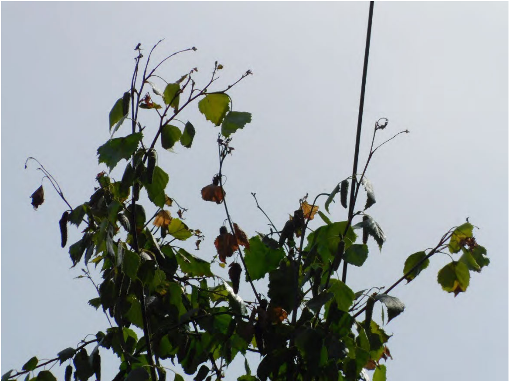
Probable violation B.160: Tree shows evidence of contacting primary conductors at 4912 SE Hill Road, Portland. (45.4189, -122.6124)
