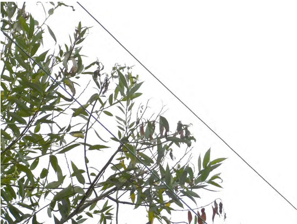
Probable violation B.152: Tree shows evidence of contacting primary conductors at 2340 SE Swain Avenue, Portland. (45.4073, -122.6402)
