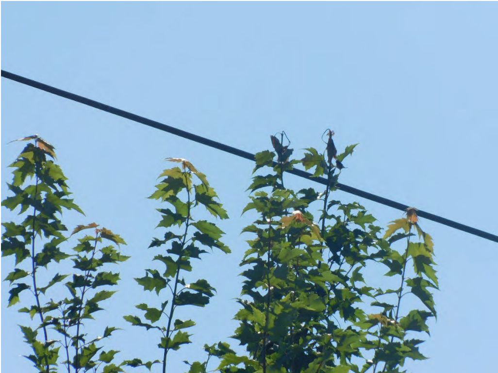
Probable violation B.210: Tree shows evidence of contacting primary conductors across from 4035 SE 82 nd Avenue, Portland. (45.4933, -122.5787)
