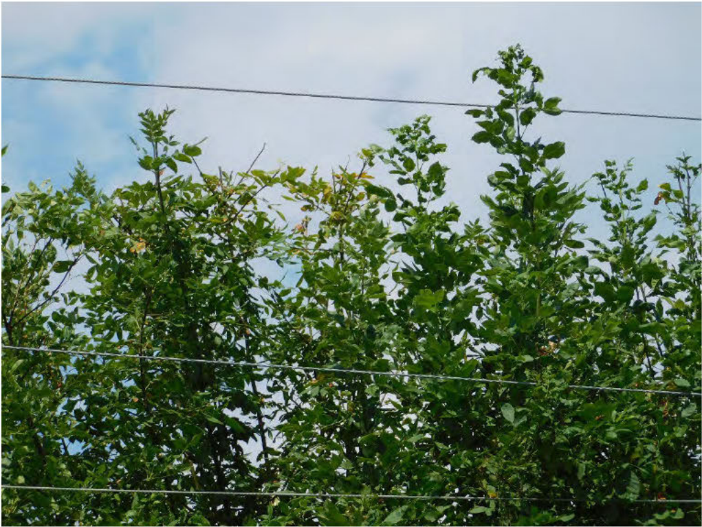
Probable violation B.270: Tree shows evidence of contacting primary conductors at 1291 62 nd Avenue SE, Salem. (44.9137, -122.9339)
