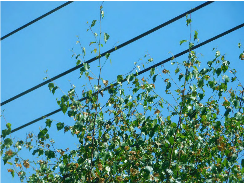
Probable violation B.301: Tree shows evidence of contacting primary conductors at 19598 Pacific Highway East, Aurora. (45.2028, -122.7791)
