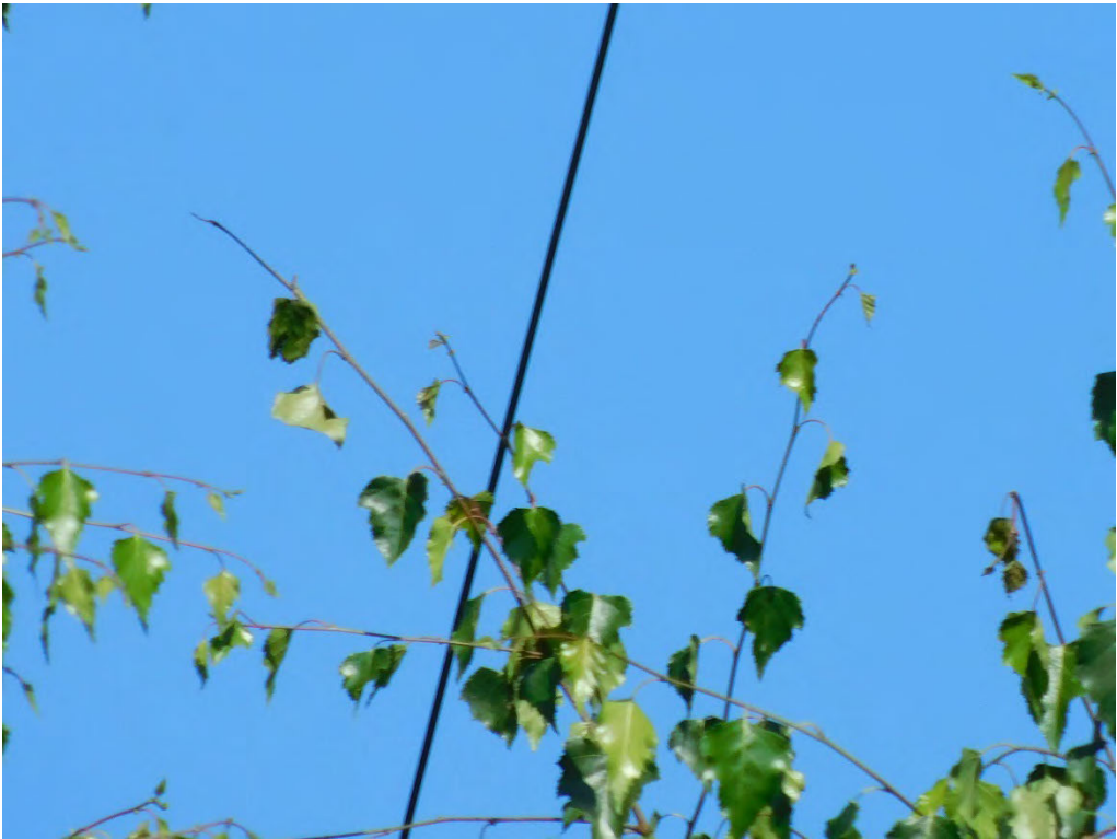
Probable violation B.292: Tree shows evidence of contacting primary conductors at 6601 Brooklake Road NE, Salem. (45.0387, -122.9256)
