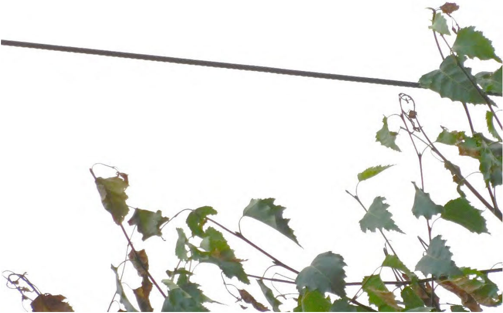
Probable violation B.25: Tree shows evidence of contacting primary conductors on NW Goodin Creek Road, Gaston. (45.4108, -123.1452) HRZ
