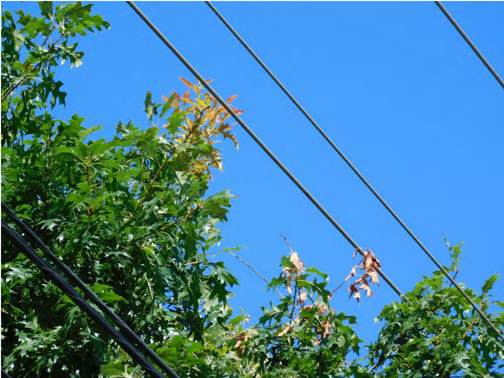
Probable violation B.45: Multiple trees show evidence of contacting the primary conductor on NE 25th Avenue, Hillsboro. (45.5438, -122.9575)
