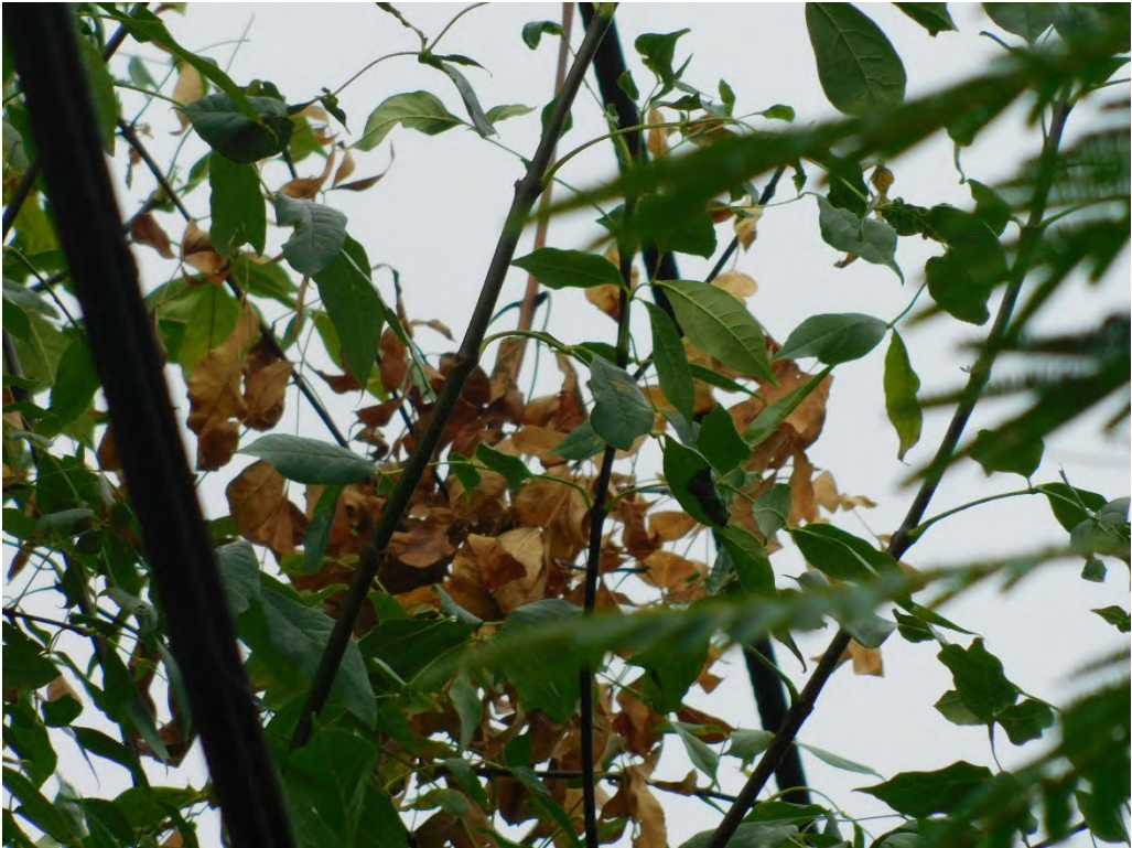
Probable violation B.101: Tree shows evidence of contacting primary conductors at 5301 SW Taylors Ferry Road, Portland. (45.4549, -122.7315)
