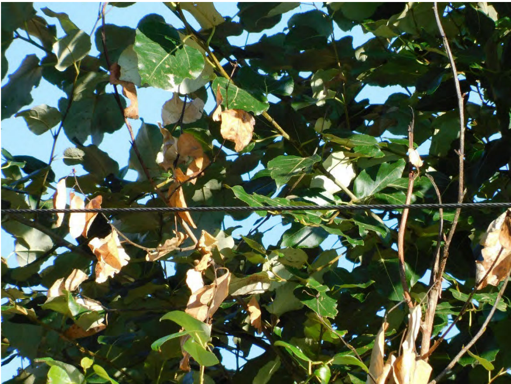
Probable violation B.18: Tree shows evidence of contacting primary conductors on Maples Street North, Keizer. (45.0137, -123.0621)
