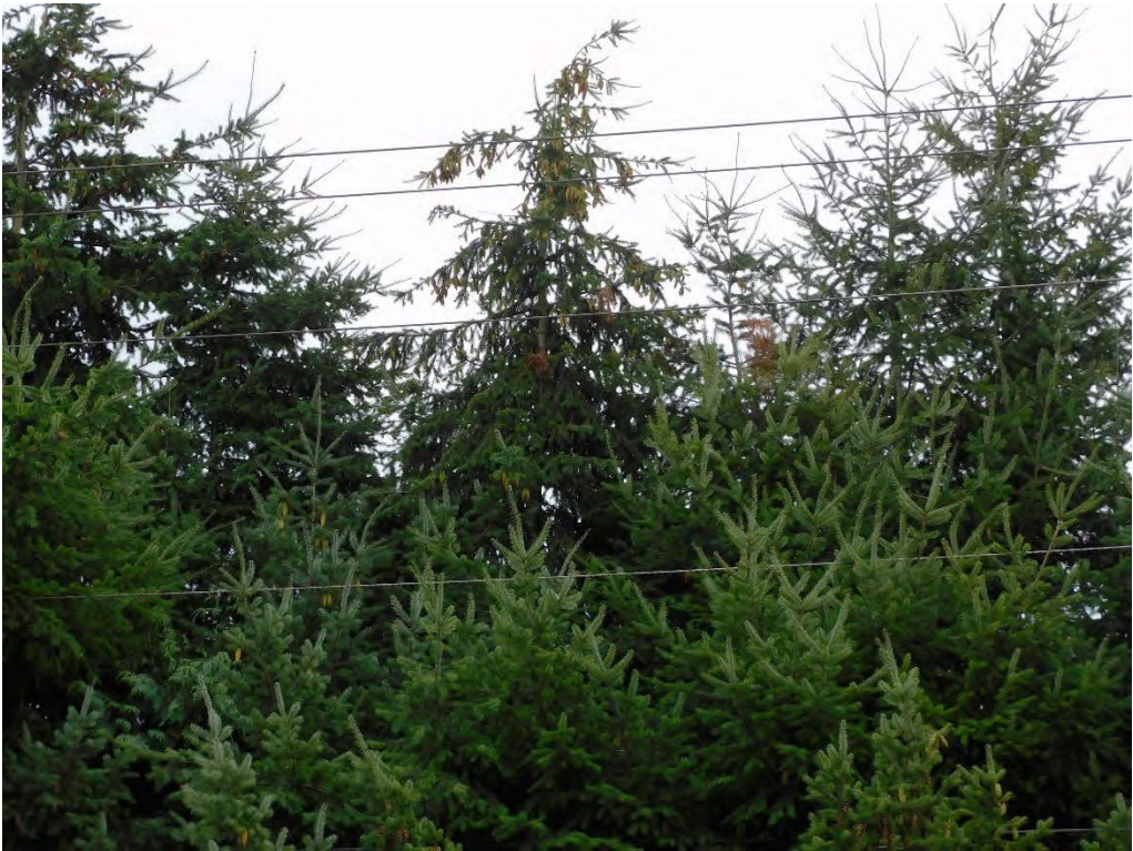
Probable violation B.367: Multiple trees show evidence of contacting primary conductors on NE Glisan Street, Portland. (45.5263, -122.5283)
