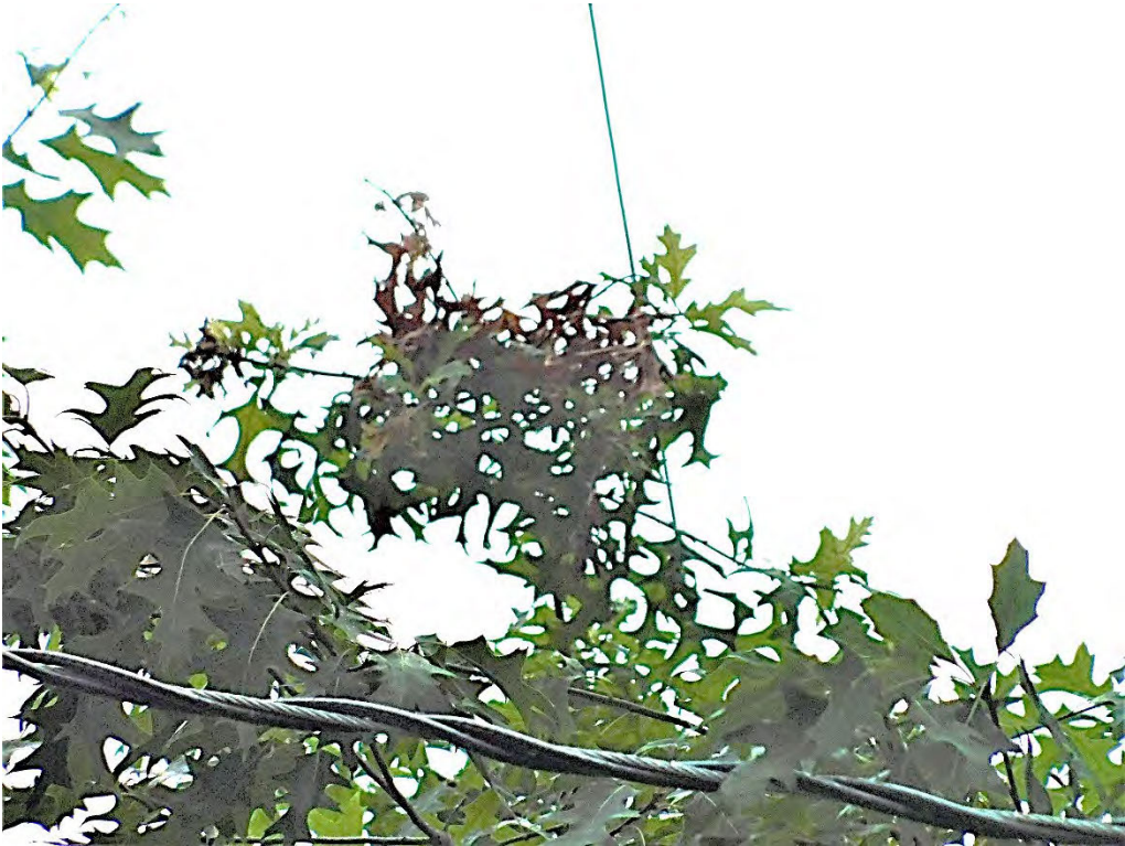
Probable violation B.157: Tree shows evidence of contacting primary conductors at 15103 SE Kellogg Avenue, Portland. (45.4137, -122.6286)
