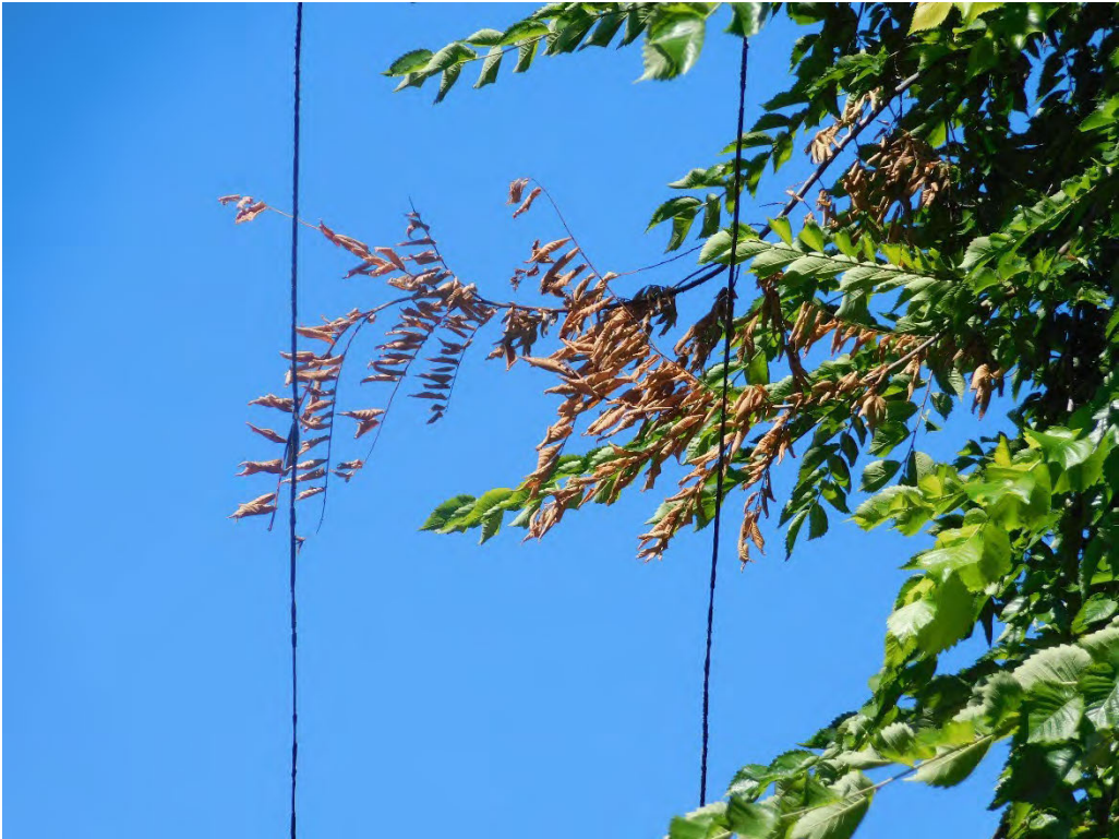
Probable violation B.65: Tree shows evidence of contacting primary conductors at 1931 NW Flanders Street, Portland. (45.5263, -122.6913)
