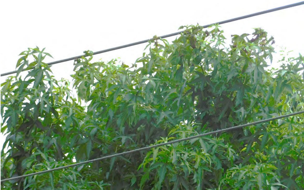
Probable violation B.191: Tree shows evidence of contacting primary conductors at 6306 SE Cedarcrest Drive, Portland. (45.4329, -122.5983)
