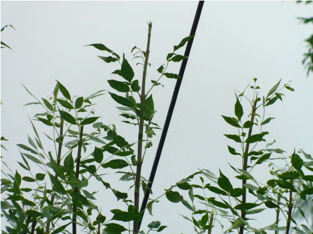
Probable violation B.91: Tree shows evidence of contacting primary conductors at 7175 SW Florence Lane, Portland. (45.4568, -122.7505)
