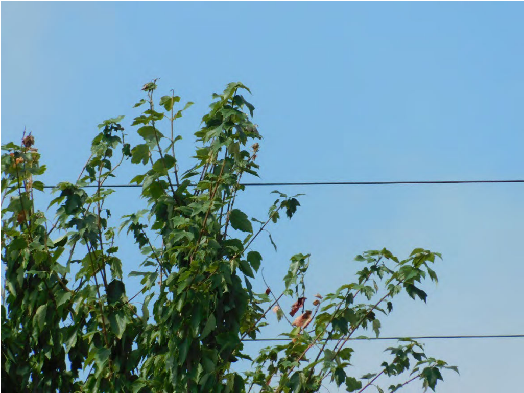
Probable violation B.148: Tree shows evidence of contacting primary conductors at 15117 SE McLoughlin Blvd., Portland. (45.4135, -122.6303)
