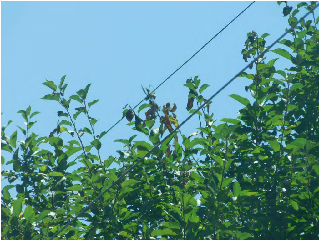
Probable violation B.326: Tree shows evidence of contacting primary conductors at 29264 South Marshal Road, Mulino. (45.1829, -122.5426)
