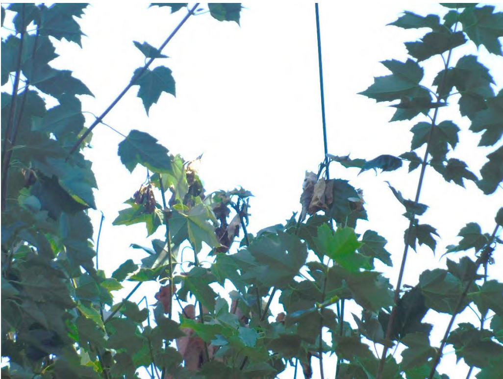
Probable violation B.232: Multiple trees show evidence of contacting the primary conductor at 6040 SE 32 nd Avenue, Portland. (45.4787, -122.6304)
