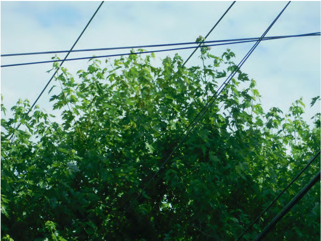
Probable violation A.15: Hazard: Readily climbable tree shows evidence of contacting the primary conductor at 4290 45 th Ave NE, Salem. (44.9813, -122.9730)
