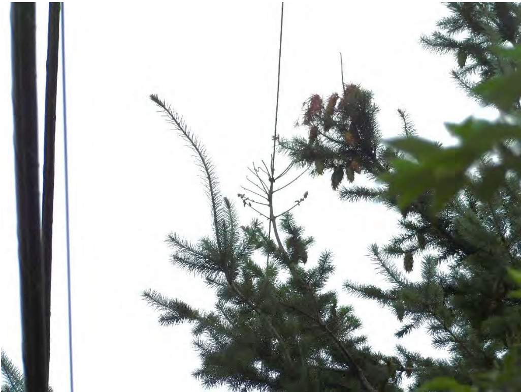
Probable violation B.186: Tree shows evidence of contacting primary conductors at 7411 SE Monroe Street, Portland. (45.4448, -122.5870)
