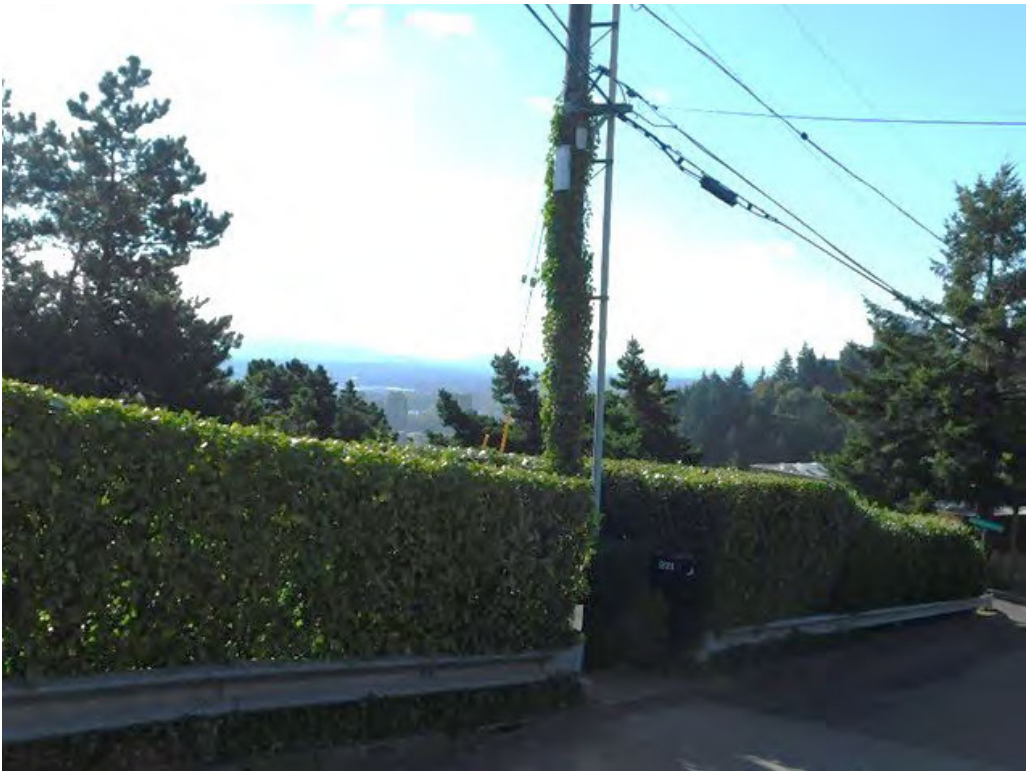
Probable violation C.18: Vines engulfing pole are creating a climbing hazard at 921 SW Davenport Street, Portland. (45.5054, -122.6879)
