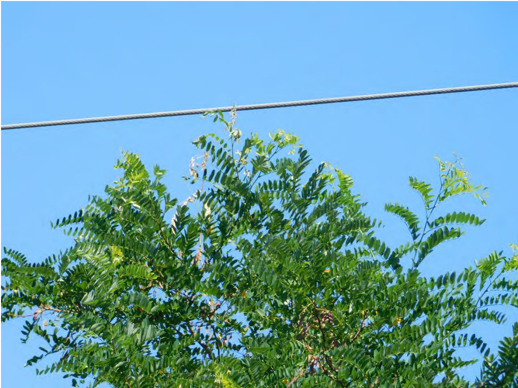
Probable violation B.128: Two trees show evidence of contacting the primary conductor at 5323 SE Jennings Avenue, Portland. (45.3928, -122.6088)
