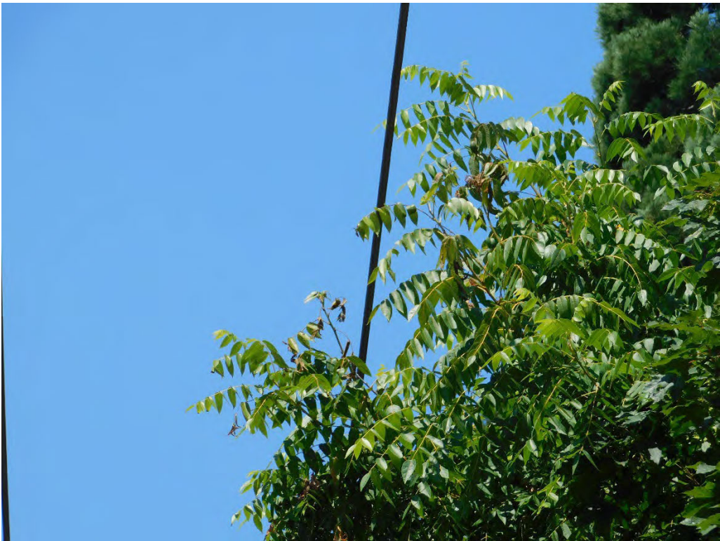
Probable violation B.172: Tree shows evidence of contacting primary conductors at 15106 SE Oatfield Road, Portland. (45.4138, -122.6239)
