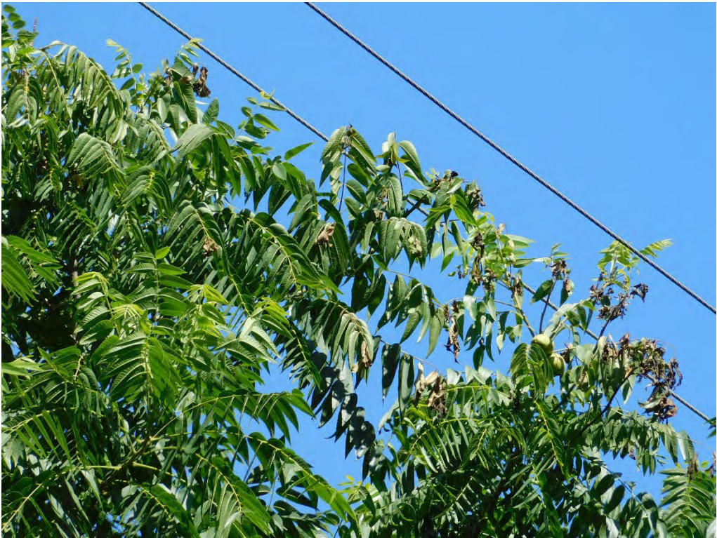
Probable violation B.298: Tree shows evidence of contacting primary conductors at 599 South Settlemier Avenue, Woodburn. (45.1386, -122.8640)
