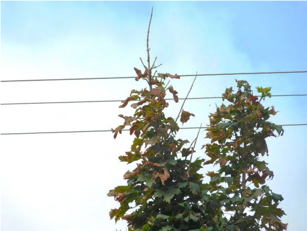
Probable violation B.149: Multiple trees show evidence of contacting the primary conductor at 14585 SE McLoughlin Blvd., Portland (45.4176, -122.6328)
