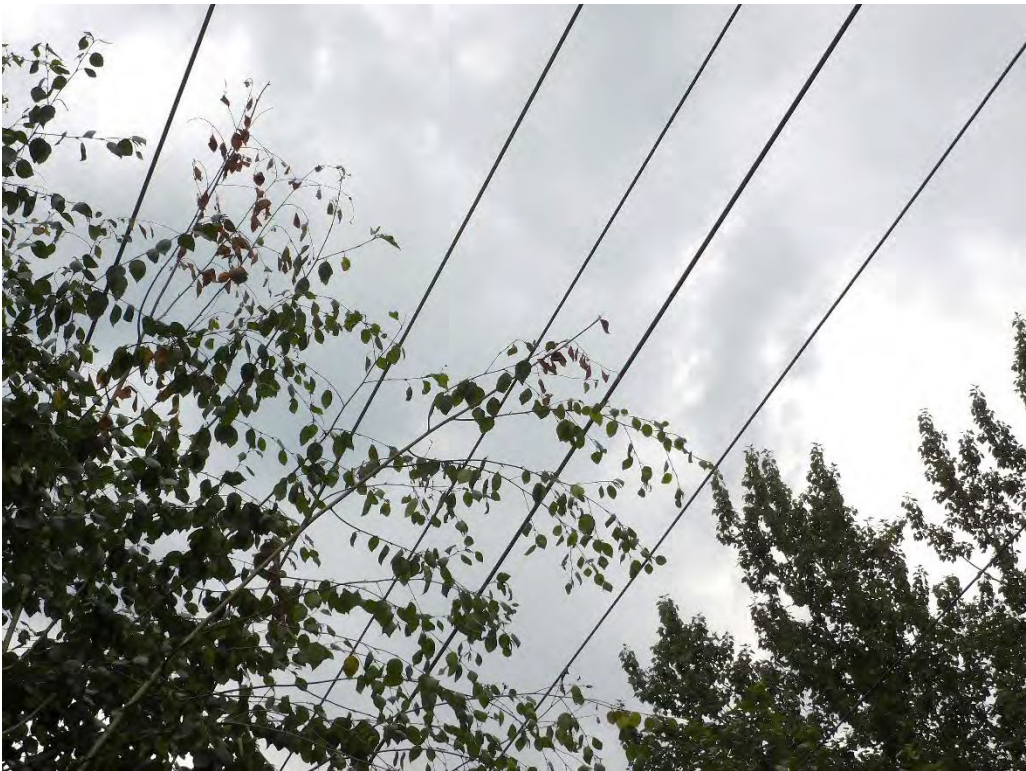
Probable violation B.358: Tree shows evidence of contacting primary conductors at 34727 SE Compton Road, Boring. (45.4327, -122.3059)
