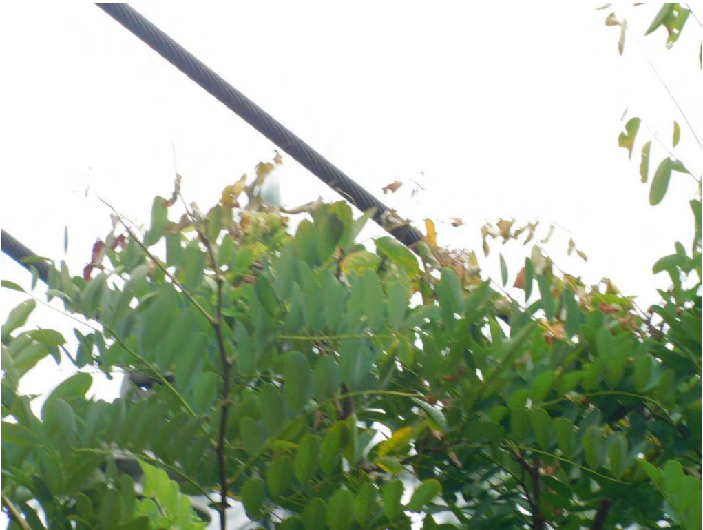
Probable violation B.104: Tree shows evidence of contacting primary conductors at 4509 SW Taylors Ferry Road, Portland. (45.4548, -122.7232)
