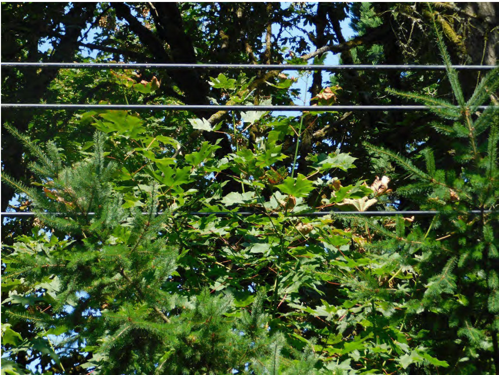
Probable violation B.79: Tree shows evidence of contacting primary conductors at the intersection of SW Arboretum Circle and West Burnside Road, Portland. (45.5191, -122.7227) HFRZ
