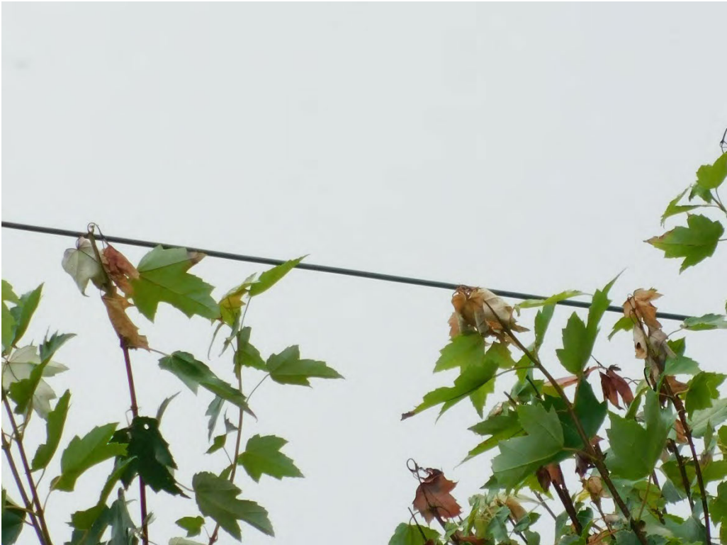
Probable violation A.12: Hazard: Readily climbable tree shows evidence of contacting the primary conductor at 1293 14 th Street, West Linn. (45.3413, -122.6553)
