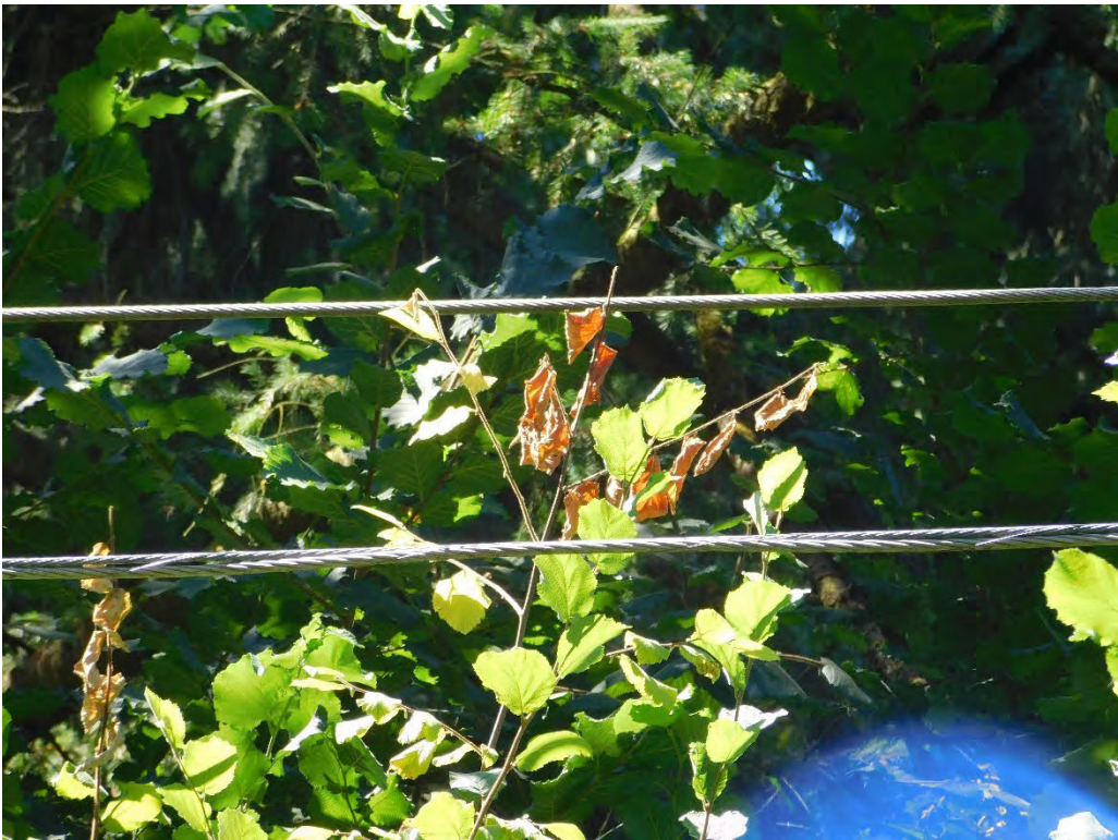
Probable violation B.22: Multiple trees show evidence of contacting the primary conductor at 26350 NE Butteville Road, Aurora. (45.2859, -122.7729)
