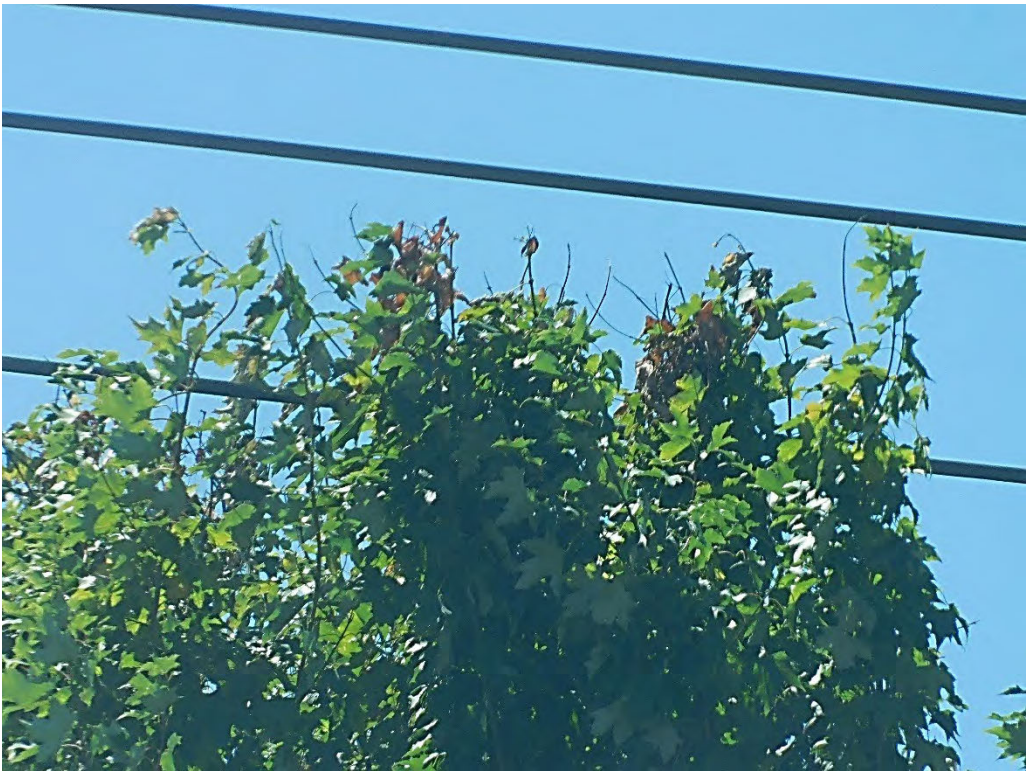
Probable violation B.75: Tree shows evidence of contacting primary conductors at 3275 NW 29 th Avenue, Portland. (45.5464, -122.7111)
