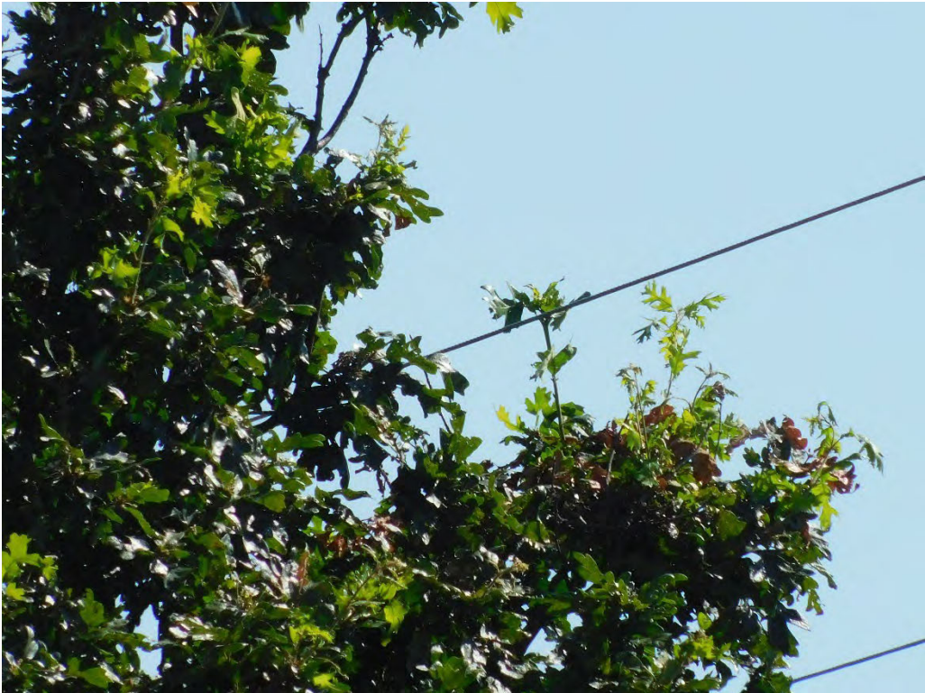
Probable violation B.313: Multiple trees show evidence of contacting primary conductors at 30286 South Molalla Avenue, Molalla. (45.1690, -122.5753)
