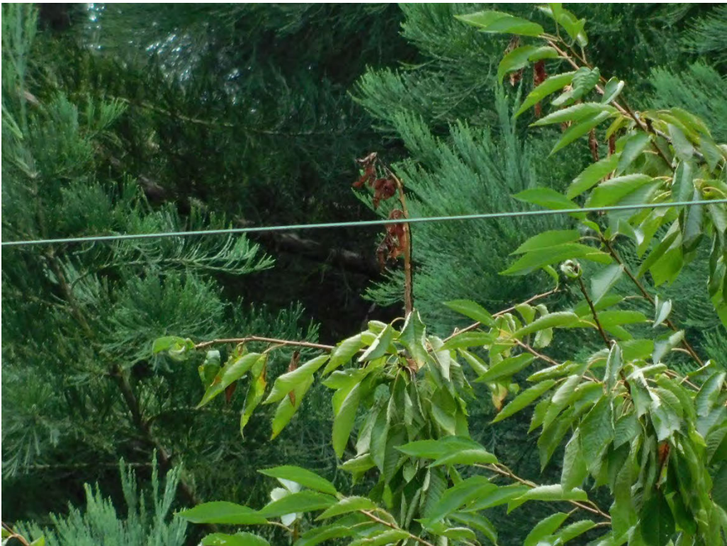
Probable violation B.236: Tree shows evidence of contacting primary conductors at 2665 SW Schaeffer Road, West Linn. (45.3492, -122.7041)
