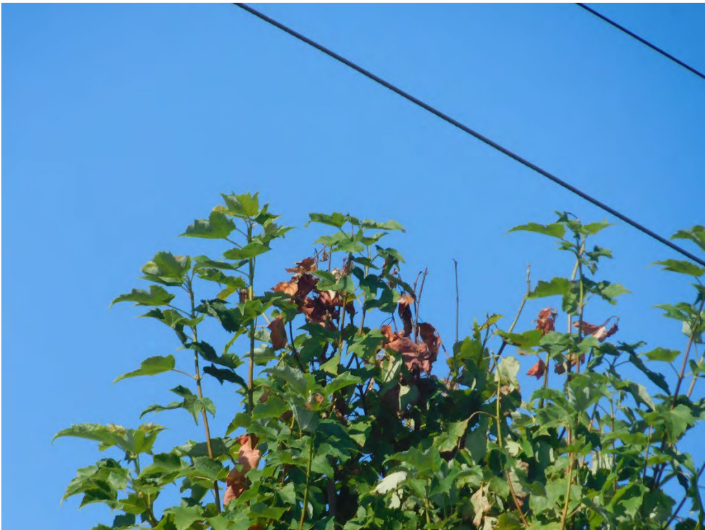
Probable violation B.206: Tree shows evidence of contacting primary conductors at 5707 SE 92 nd Avenue, Portland. (45.4813, -122.5692)
