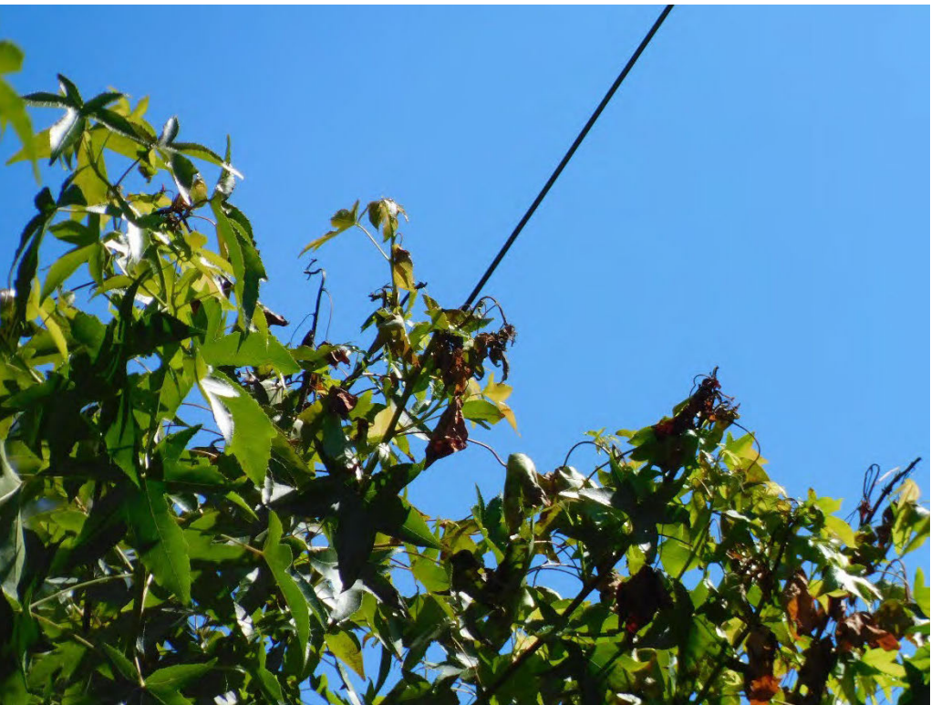
Probable violation B.140: Multiple trees show evidence of contacting the primary conductor at 2762 SE Vineyard Way, Portland. (45.4007, -122.6346)
