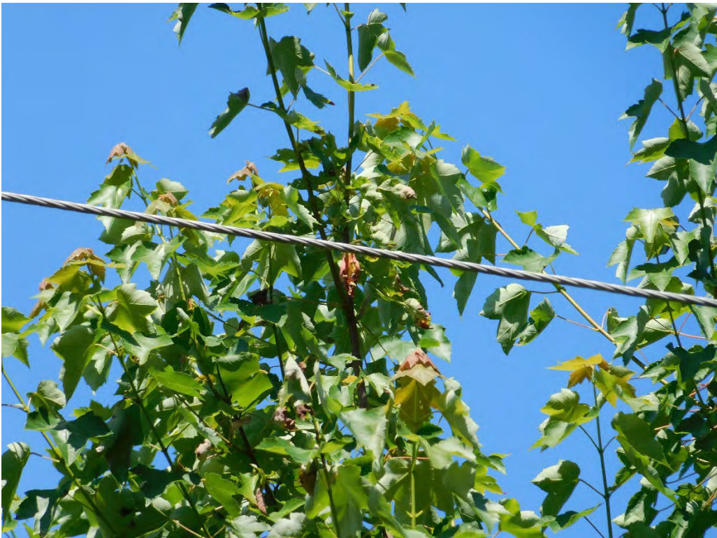
Probable violation B.253: Multiple trees show evidence of contacting primary conductors at 7937 Pine Tree Lane SE, Turner. (44.8398, -122.9309)
