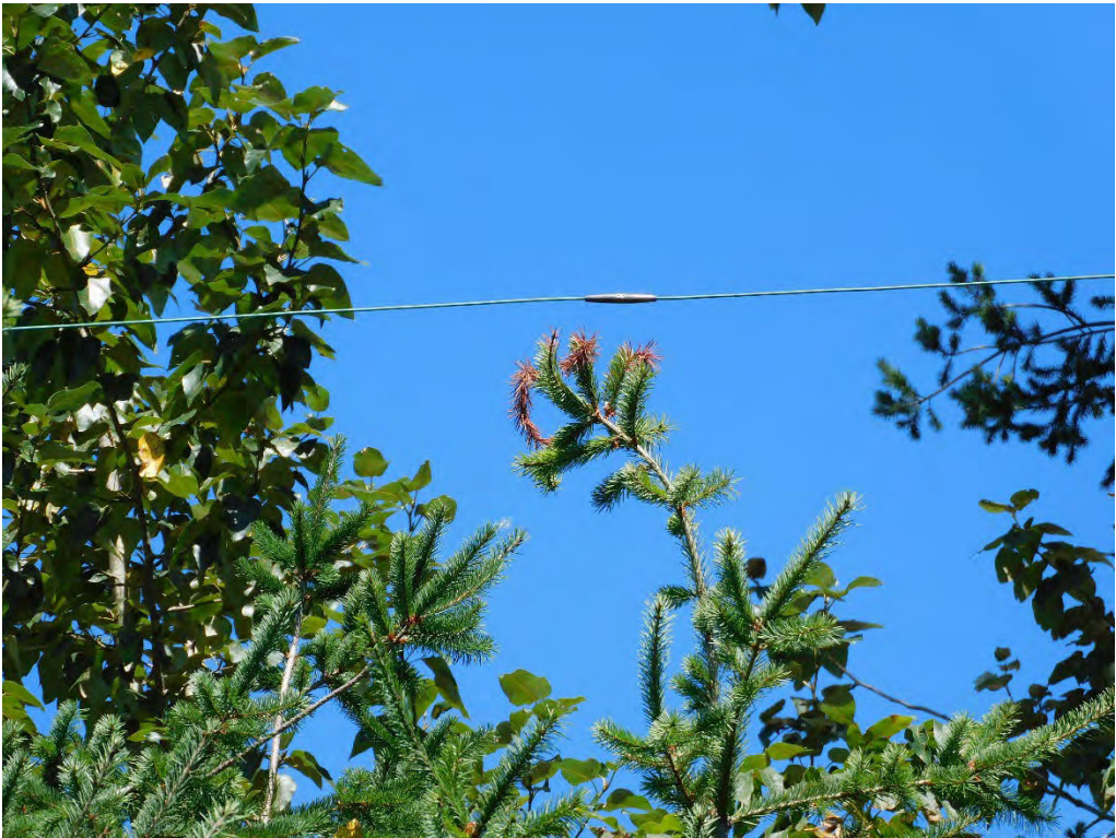
Probable violation B.349: Tree shows evidence of contacting primary conductors at 3514 SE 317th Avenue, Troutdale. (45.4976, -122.3367)
