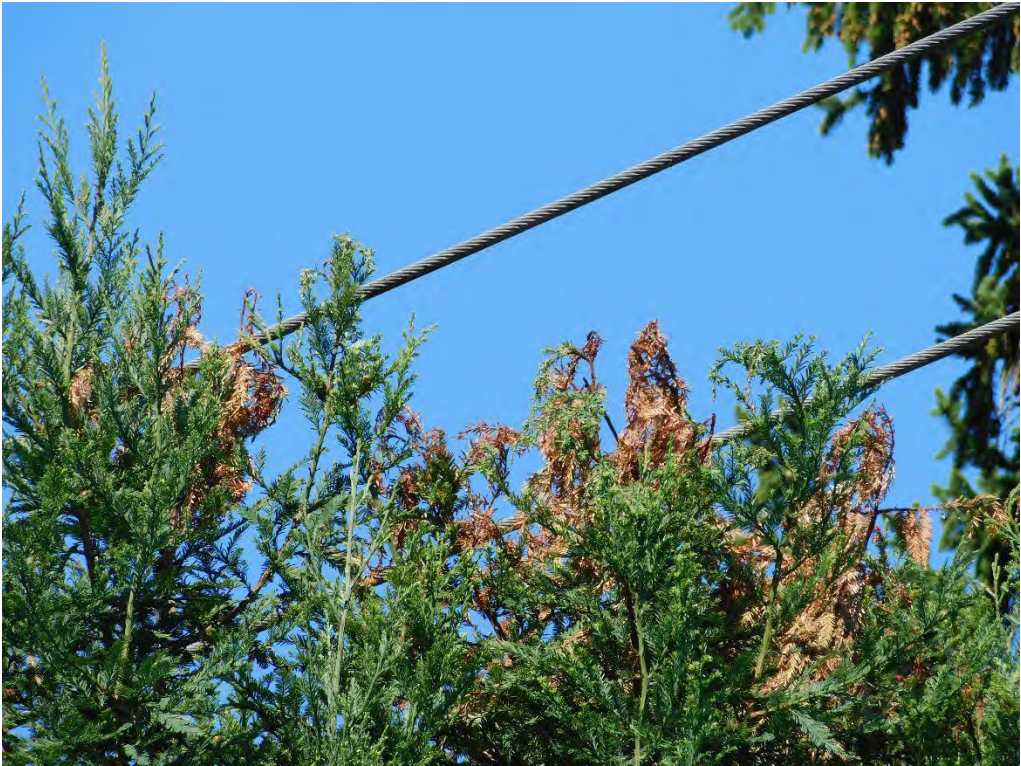
Probable violation B.127: Tree shows evidence of contacting primary conductors at the intersection of SE Emerald Drive and SE Jennings Avenue, Portland. (45.3948, -122.6041)
