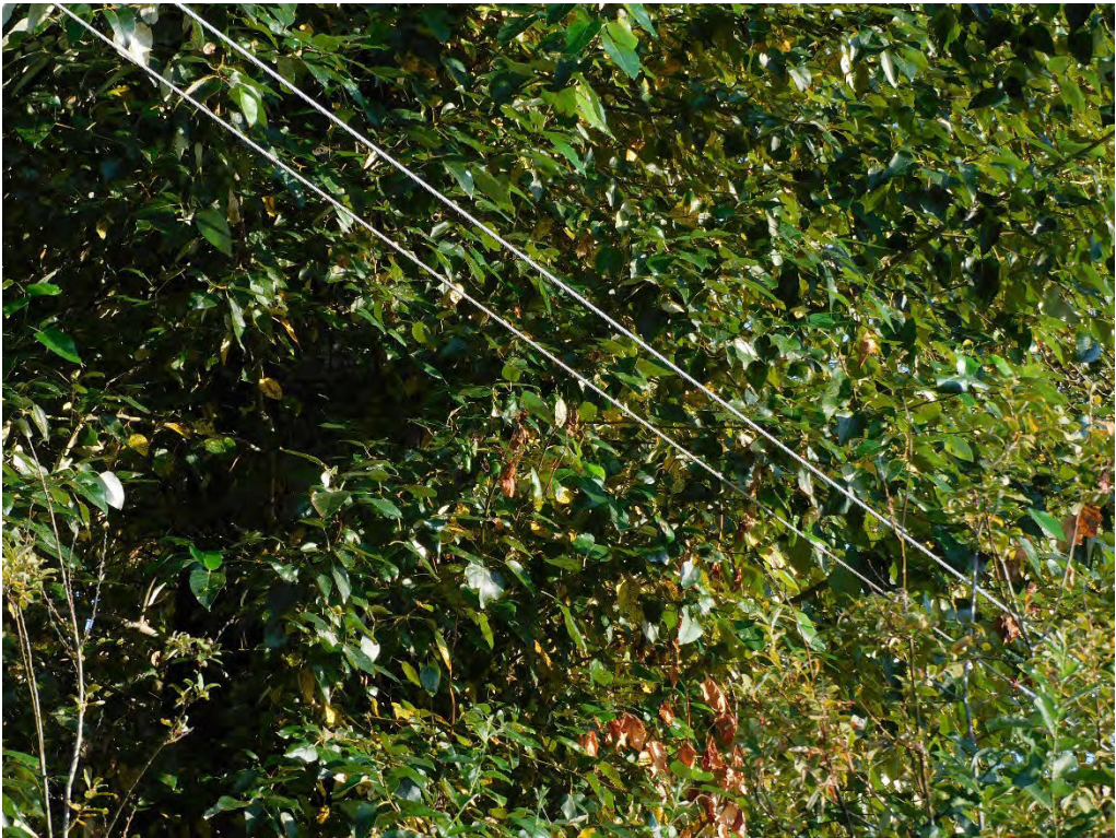
Probable violation B.343: Two trees show evidence of contacting primary conductors on South Gerber Road, Oregon City. (45.3737, -122.4433)
