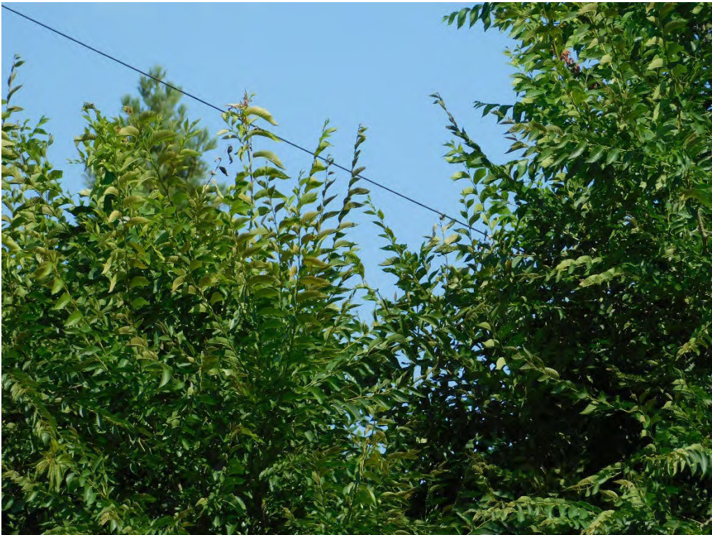
Probable violation B.268: Tree shows evidence of contacting primary conductors at 3507 Middle Grove Dr NE, Salem. (44.9703, – 122.9616)
