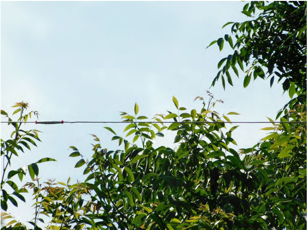
Probable violation B.1: Tree shows evidence of contacting primary conductors on Kuebler Blvd., South, Salem. (44.8832, -123.0847)
