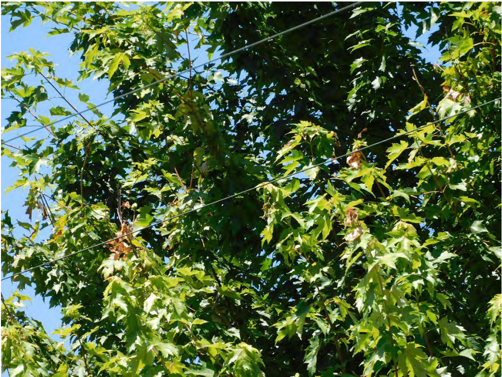
Probable violation B.54: Tree shows evidence of contacting primary conductors at 4065 SE Bentley Street, Hillsboro. (45.5123, -122.9410)
