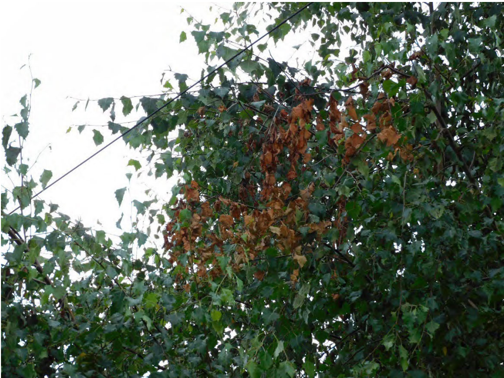
Probable violation B.364: Tree shows evidence of contacting primary conductors at 8444 SE Orient Drive, Gresham. (45.462, -122.3486)
