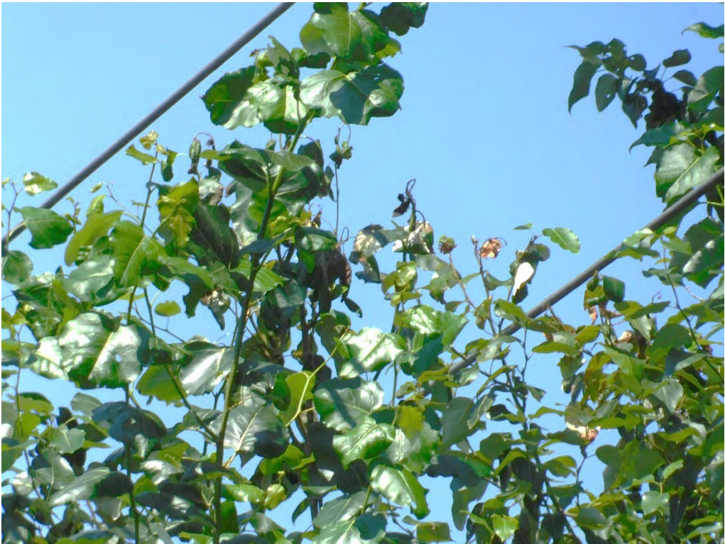
Probable violation B.171: Multiple trees show evidence of contacting the primary conductor at 16704 SE Oatfield Road, Portland. (45.4024, -122.6092)
