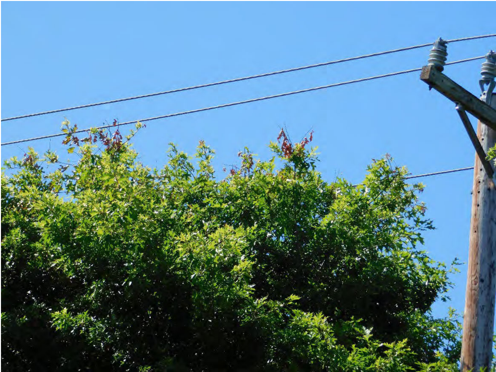
Probable violation B.135: Multiple trees show evidence of contacting the primary conductor at 19555 River Road, Portland. (45.3806, -122.6069)
