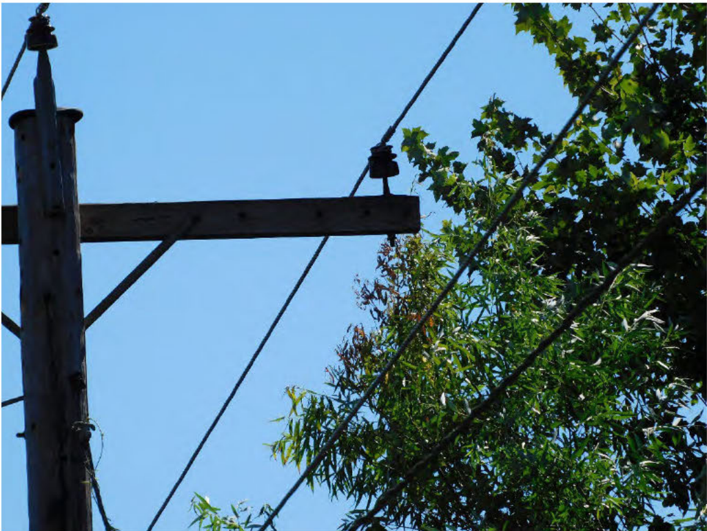
Probable violation B.348: Tree shows evidence of contacting primary conductors on US-30 Historic, Troutdale. (45.5189, -122.3367)
