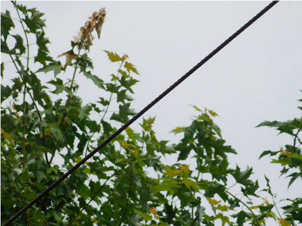
Probable violation B.194: Multiple spans show evidence of multiple trees contacting the primary conductor on SE Railroad Avenue, Portland. (45.4362, -122.6096) to (45.4430, -122.6236)
