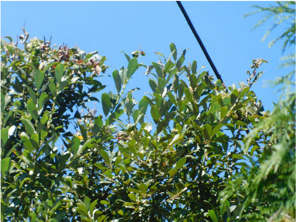
Probable violation B.76: Tree shows evidence of contacting primary conductors at 4465 NW Yeon Avenue, Portland. (45.5545, -122.7329)
