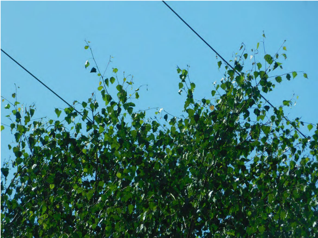
Probable violation B.293: Tree shows evidence of contacting primary conductors at 8646 Lakeside Drive NE, Salem. (45.0427, -122.9313)
