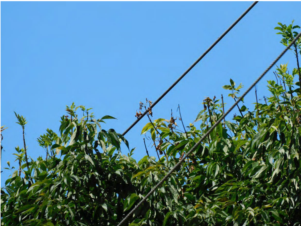
Probable violation B.354: Multiple trees show evidence of contacting primary conductors at the intersection of SE Dodge Park Blvd. and SE 302nd Avenue, Gresham. (45.4708, -122.3528)
