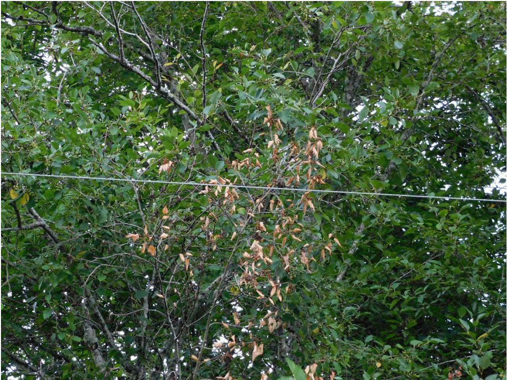
Probable violation B.365: Tree shows evidence of contacting primary conductors across from 8801 SE 307th Avenue, Boring. (45.4591, -122.3471)
