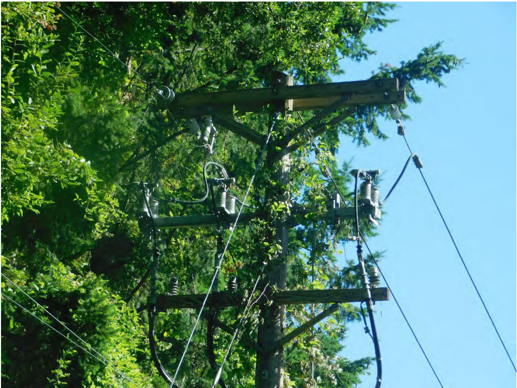
Probable violation C.9: Vines engulfing pole and approaching primary conductor are creating a hazard at 2710 SE Rutland Terrace, Portland. (45.5209, -122.7082)
