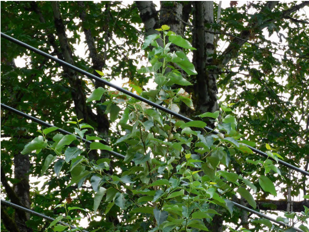
Probable violation B.377: Tree shows evidence of contacting primary conductors on SE Regner Road, Gresham. (45.4782, -122.4292)
