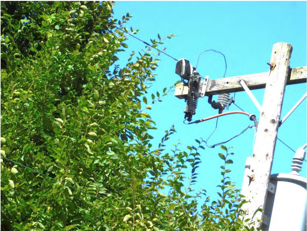
Probable violation B.133: Tree shows evidence of contacting primary conductors at 4785 SE La Cour Court, Portland. (45.3815, -122.6148)
