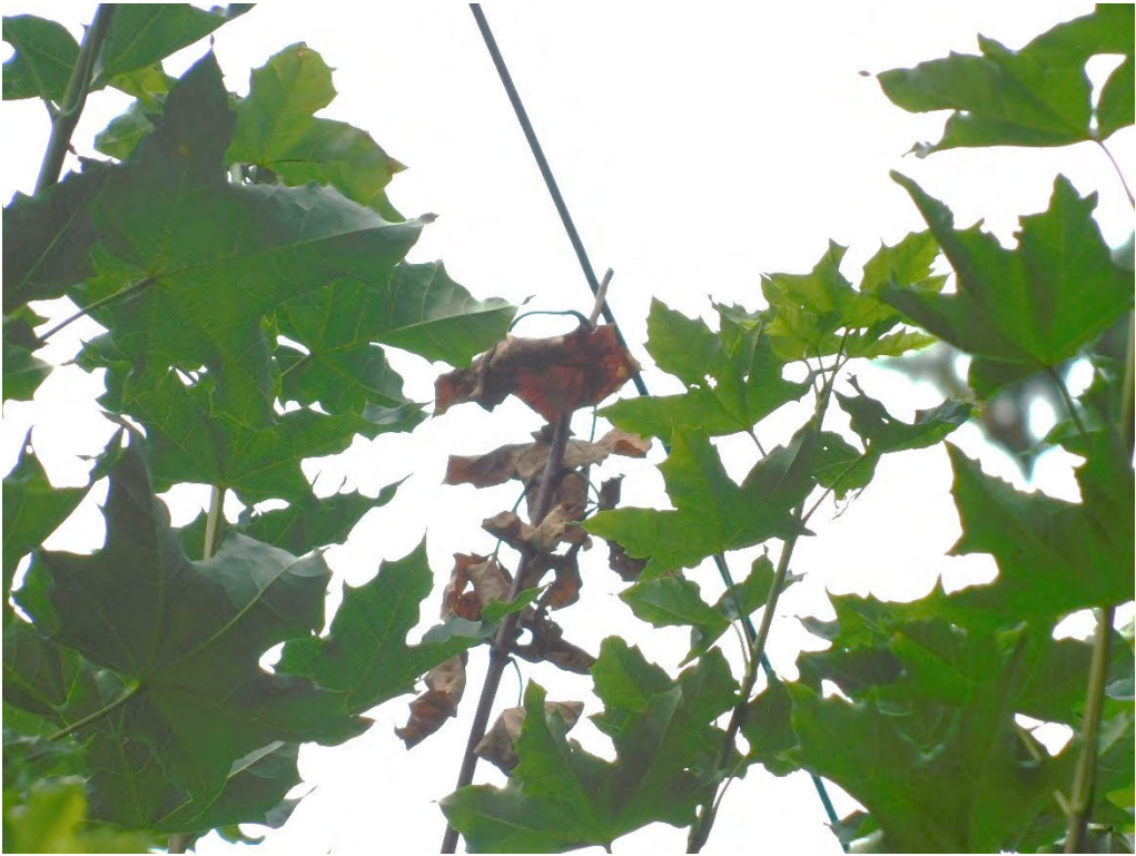
Probable violation B.100: Tree shows evidence of contacting primary conductors at 9423 SW 62 nd Drive, Portland. (45.4572, -122.7418)
