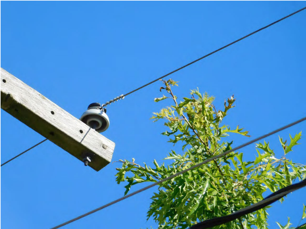
Probable violation B.312: Tree shows evidence of contacting primary conductors at 30330 South Molalla Avenue, Molalla. (45.1678, -122.5757)
