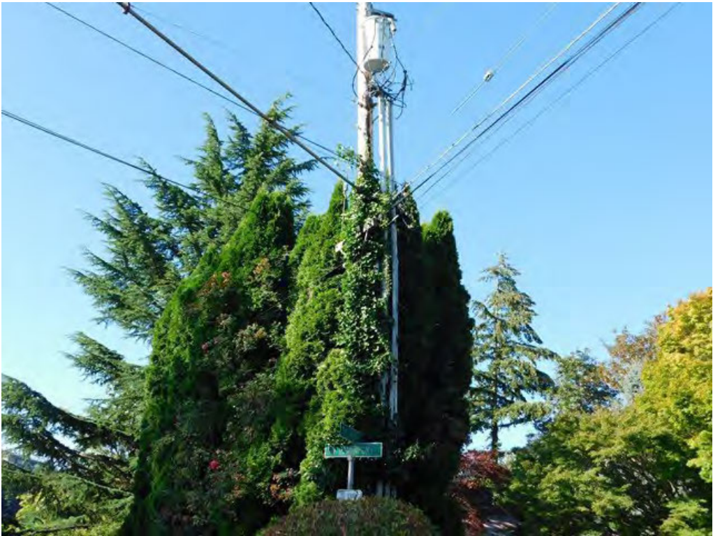
Probable violation C.19: Vines engulfing pole are creating a climbing hazard at 840 SW Canning Street, Portland. (45.5046, -122.6879)
