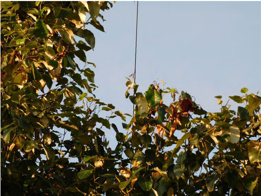
Probable violation B.340: Tree shows evidence of contacting primary conductors at 15908 South Springwater Road, Oregon City. (45.3753, -122.4744)
