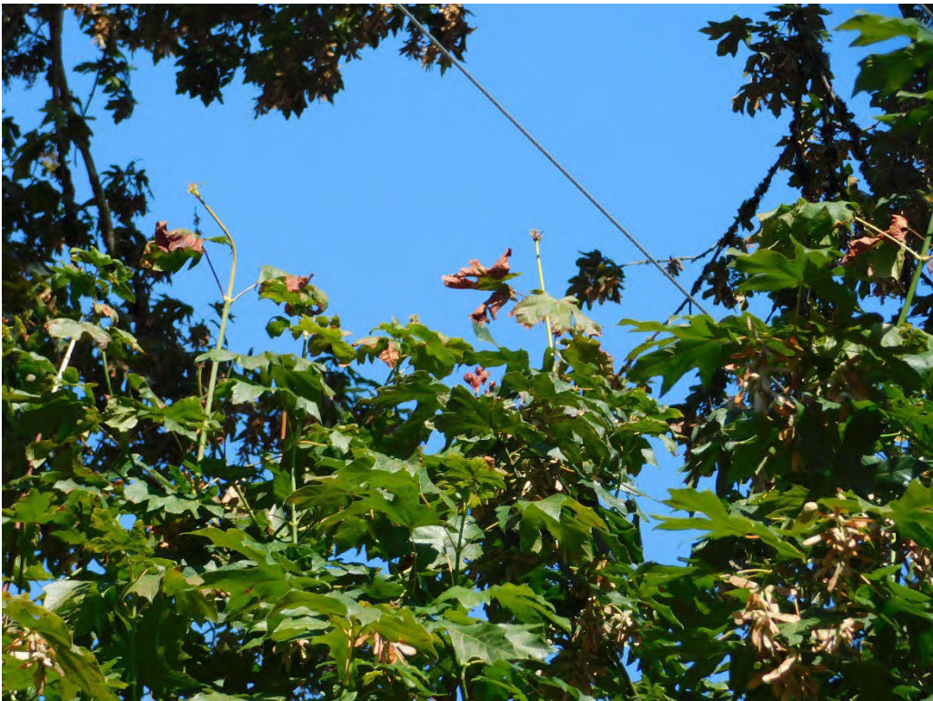
Probable violation B.130: Tree shows evidence of contacting primary conductors at 4215 SE Jennings Avenue, Portland. (45.3891, -122.6195)
