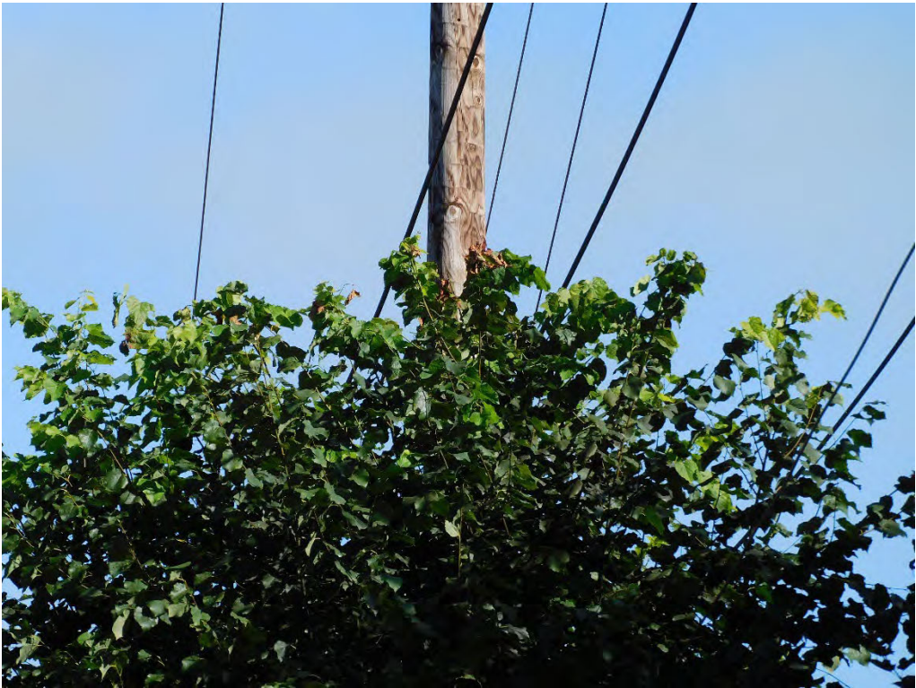
Probable violation B.345: Tree shows evidence of contacting primary conductors at 13780 SE Bluff, Sandy. (45.4238, -122.2742)
