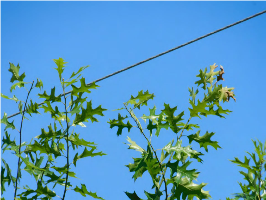
Probable violation B.296: Tree shows evidence of contacting primary conductors at 110 Lincoln Street, Mount Angel. (45.0677, -122.8022)
