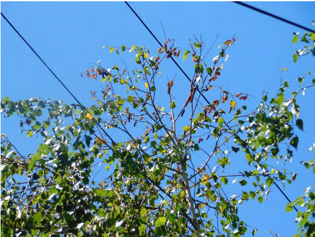
Probable violation B.71: Multiple trees show evidence of contacting the primary conductor at 2844 NW Raleigh Street, Portland. (45.5338, -122.7097)
