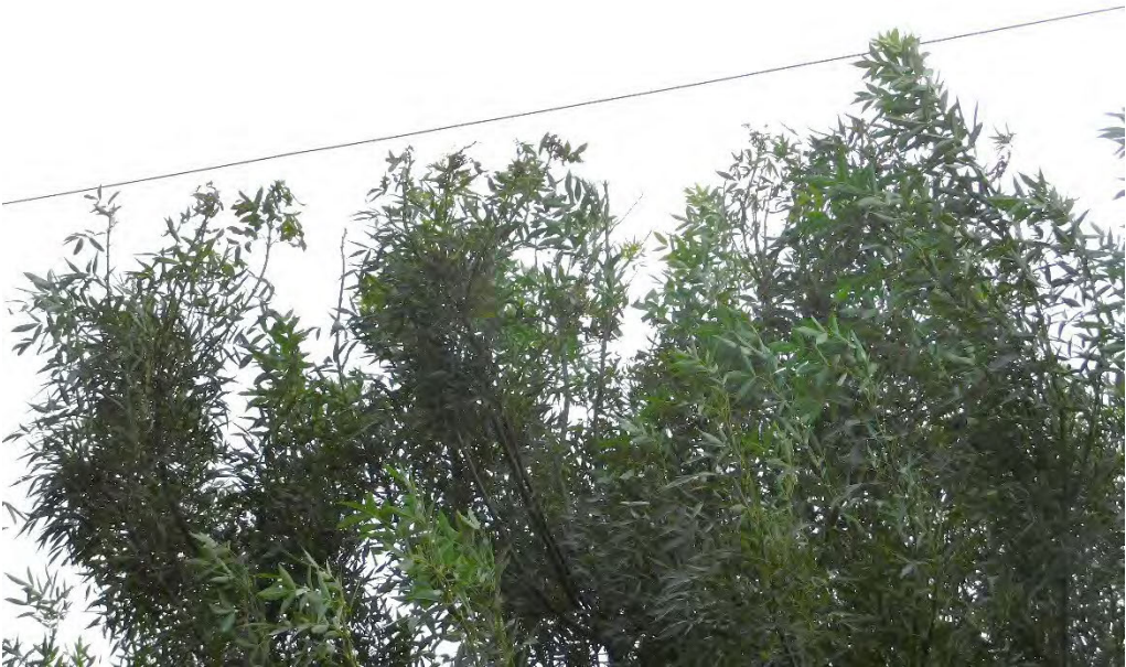
Probable violation B.187: Tree shows evidence of contacting primary conductors at 6710 SE Catalina Lane, Portland. (45.4426 , -122.5941)
