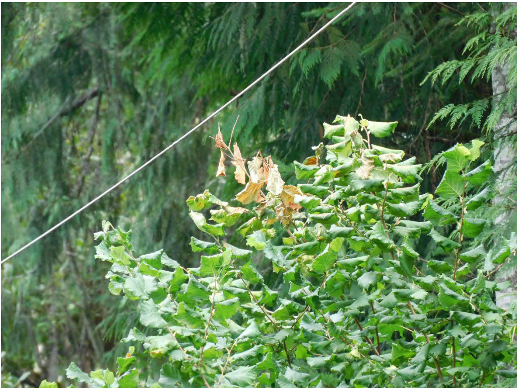
Probable violation B.39: Tree shows evidence of contacting primary conductors on NW Davidson Road, Banks. (45.6463, -123.0835) HFRZ
