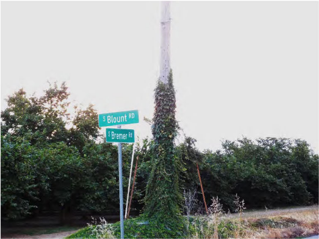
Probable violation C.23: Vines engulfing pole are creating a climbing hazard at the intersection of South Blount Road and South Bremer Road, Canby. (45.2711, -122.6557)
