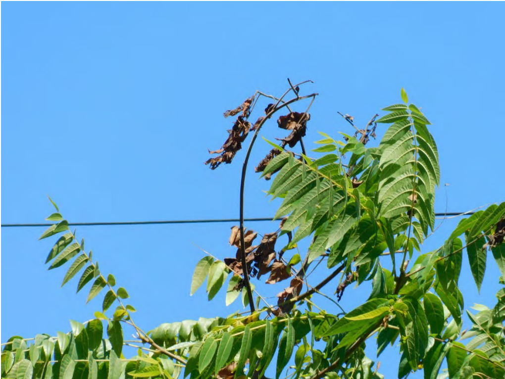
Probable violation B.112: Tree shows evidence of contacting primary conductors at 1737 SW Canby Street, Portland. (45.4691, -122.6960)
