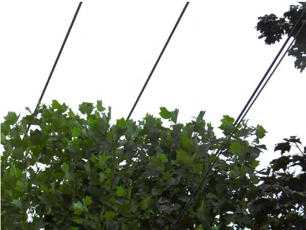
Probable violation B.182: Multiple trees show evidence of contacting the primary conductor at 11200 SE Fuller Road, Portland. (45.4418, -122.5817)
