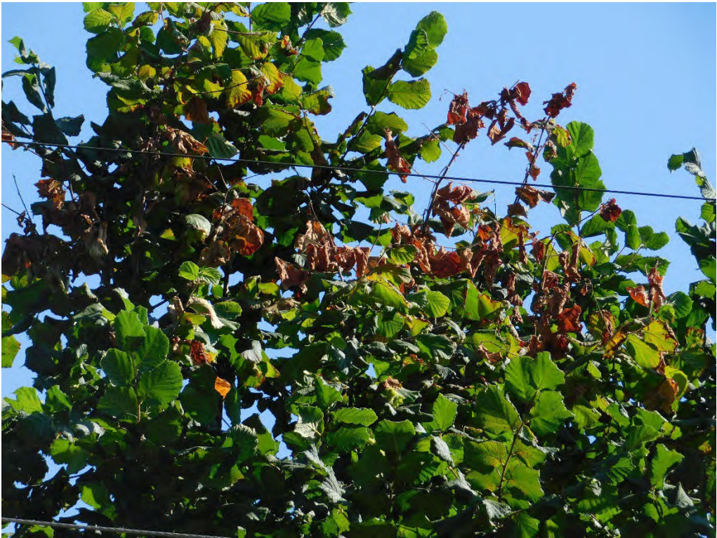
Probable violation B.290: Two trees in an orchard, creating a hazard , show evidence of contacting the primary conductor across from 6060 Brooklake Road NE, Salem. (45.0417, -122.9362)
