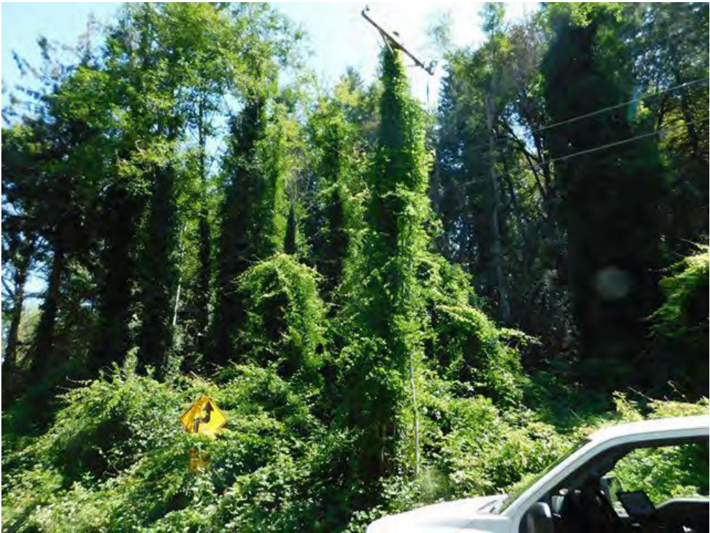
Probable violation C.11: Vines engulfing pole and approaching primary conductor are creating a hazard on SW Prosperity Park Road, Tualatin. (45.3712, -122.7300)
