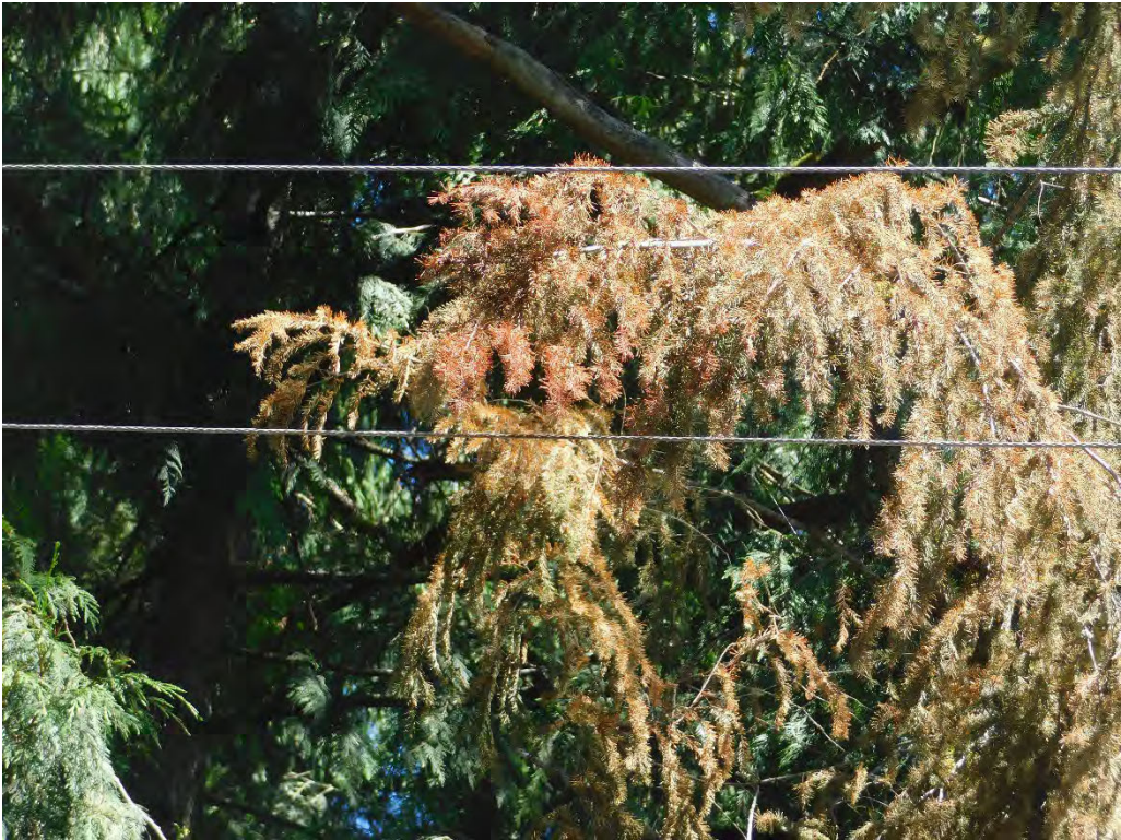
Probable violation B.319: Tree shows evidence of contacting primary conductors across from 25949 South Hillockburn Road, Estacada. (45.2303, -122.3247)
