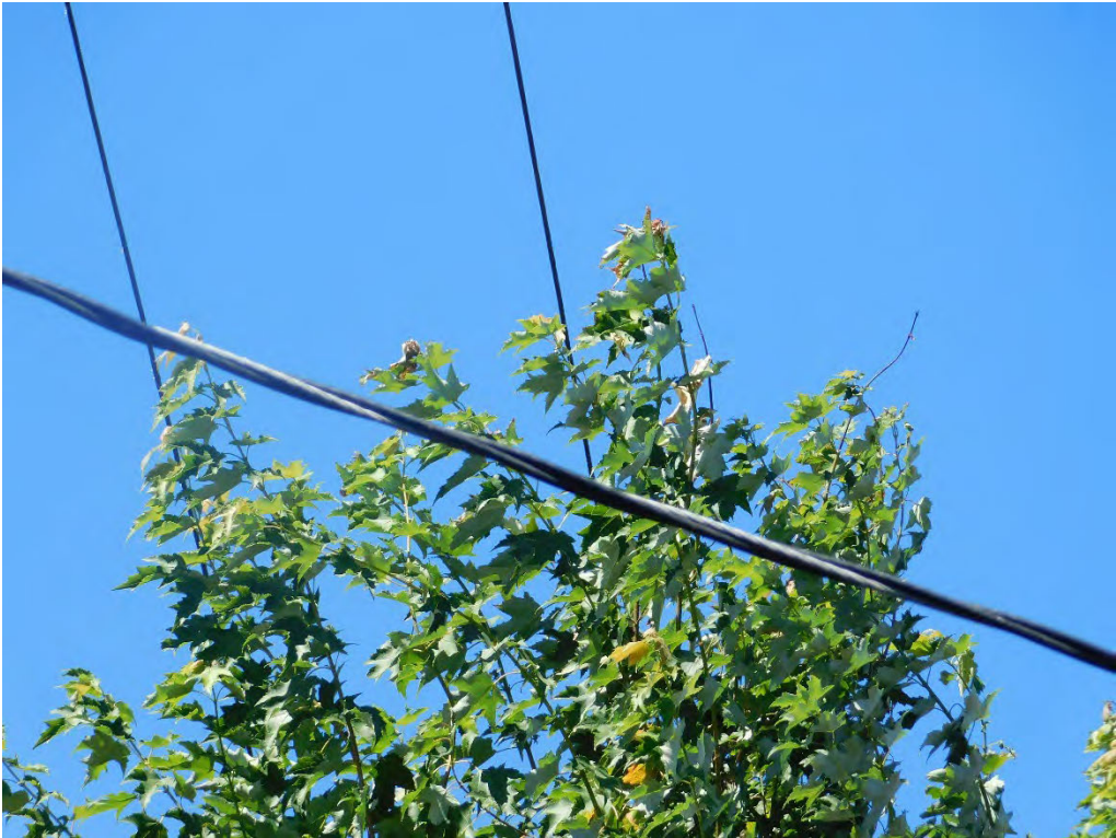
Probable violation B.66: Tree shows evidence of contacting primary conductors at 2230 NW Glisan Street, Portland. (45.5262, -122.6973)
