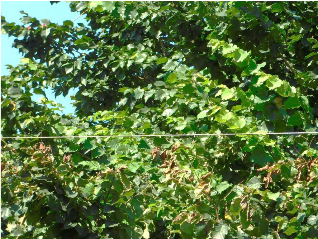
Probable violation B.9: Multiple trees show evidence of contacting the primary conductor on Jackson Hill Road SE, Salem. (44.8322, -123.0301)
