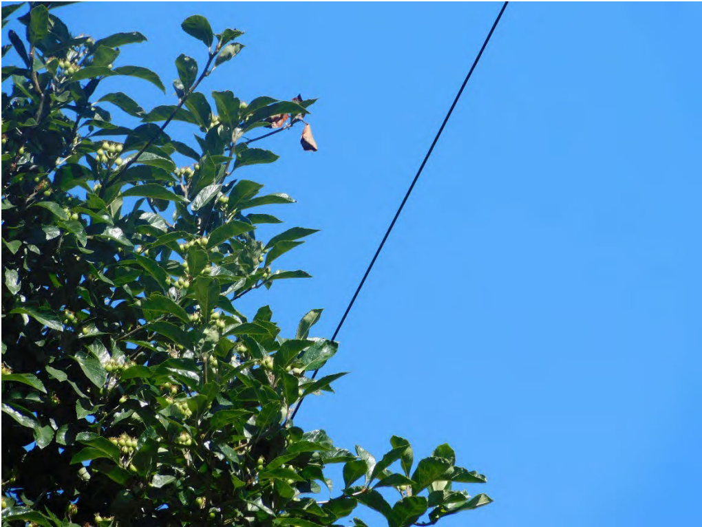
Probable violation B.60: Tree shows evidence of contacting primary conductors at 2610 NW Cornell Road, Portland. (45.5298, -122.7048)
