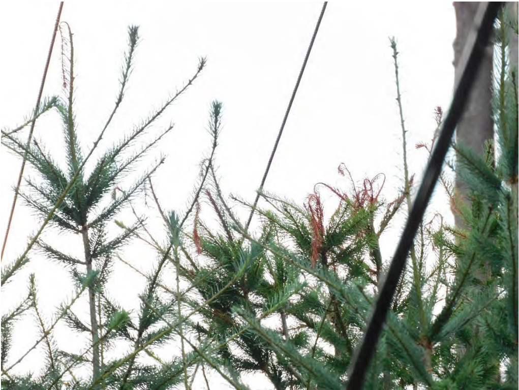
Probable violation B.359: Tree shows evidence of contacting primary conductors at 33755 SE Compton Road, Boring. (45.4327, -122.3154)
