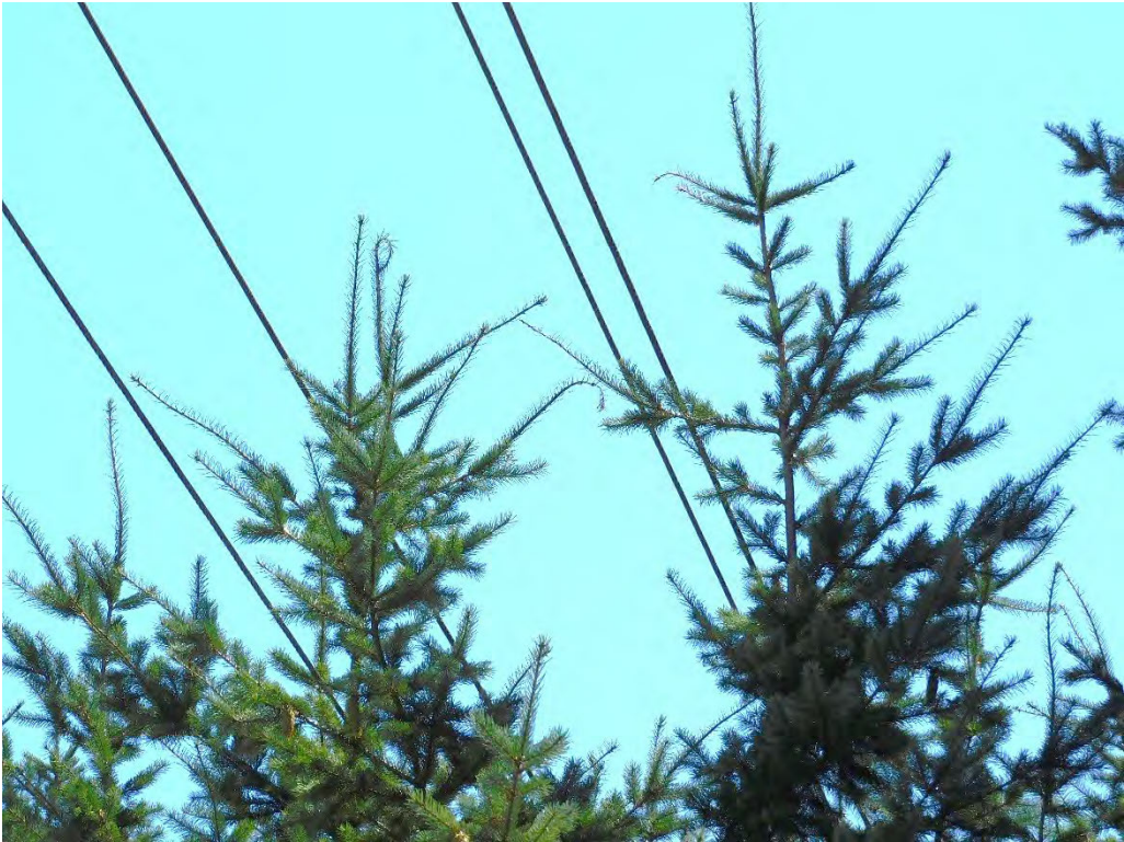
Probable violation B.33: Multiple trees show evidence of contacting the primary conductor at 32710 SW Tongue Lane, Cornelius. (45.4849, -123.0141)
