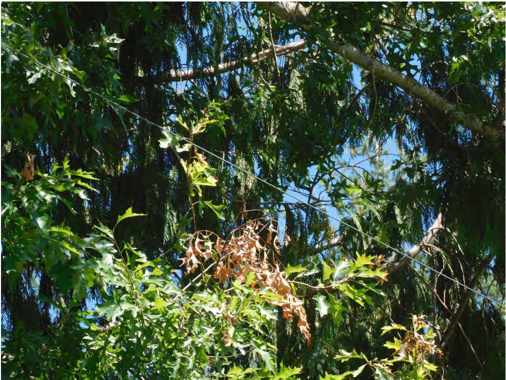
Probable violation B.355: Tree shows evidence of contacting primary conductors on SE Jackson Road, Gresham. (45.4739, -122.3493)
