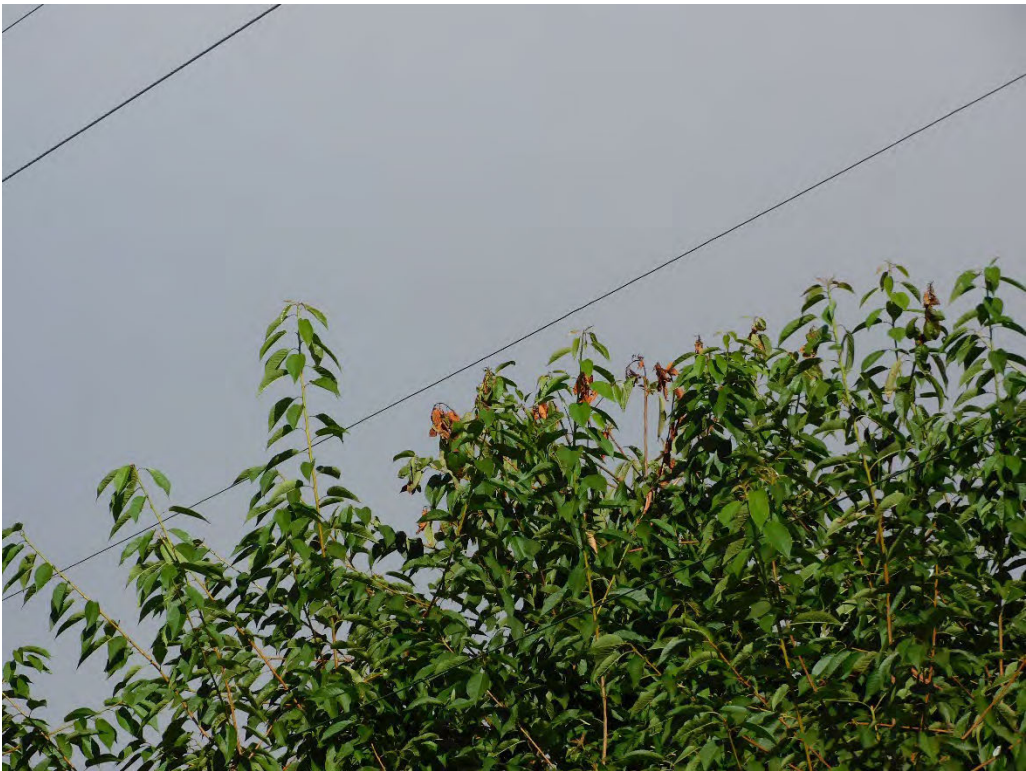
Probable violation B.346: Two trees show evidence of contacting primary conductors on SE Hudson Road, Boring. (45.4435, -122.2744)
