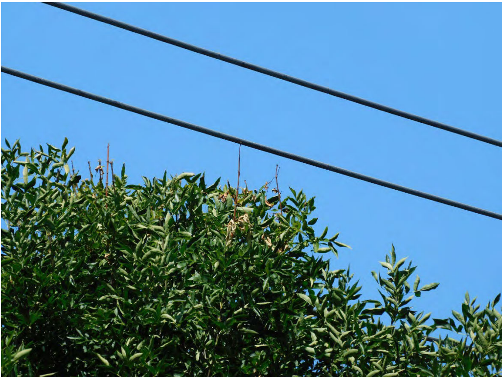
Probable violation B.53: Tree shows evidence of contacting primary conductors at 1276 NW Perl Way, Beaverton. (45.5288, -122.8891)
