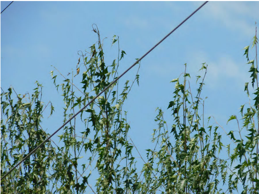
Probable violation B.273: Tree shows evidence of contacting primary conductors across from 10844 Kaufman Road NE, Silverton. (44.9697, -122.8388)
