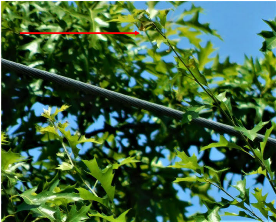
Probable violation B.260: Multiple trees show evidence of contacting primary conductors at 4579 Lancaster Drive NE, Salem. (44.9872, -122.9833)
