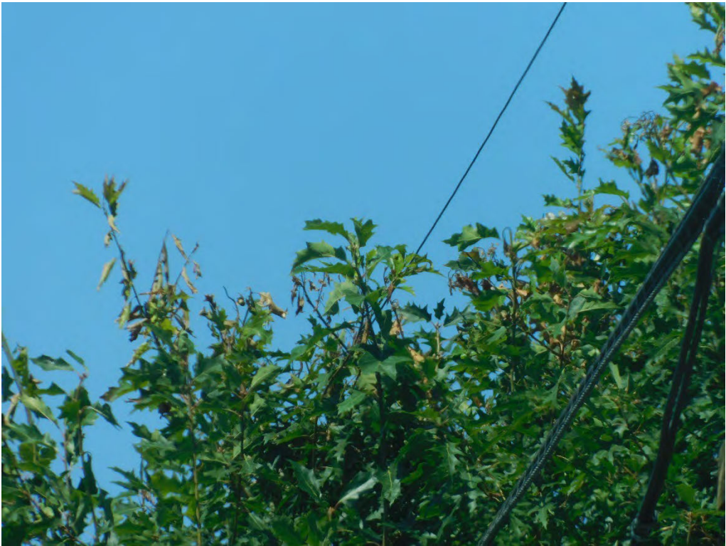
Probable violation B.215: Tree shows evidence of contacting primary conductors at 7005 SE Mitchell Street, Portland. (45.4857, -122.5912)
