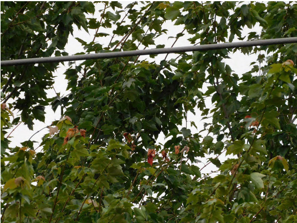
Probable violation B.344: Multiple trees show evidence of contacting primary conductors at 13300 SE Hubbard Road, Clackamas. (45.4140, -122.5274)
