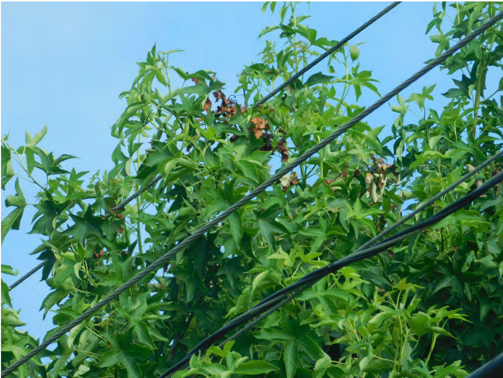
Probable violation B.280: Tree shows evidence of contacting primary conductors at 4565 Hazelgreen Road NE, Salem. (45.0046, -122.9677)
