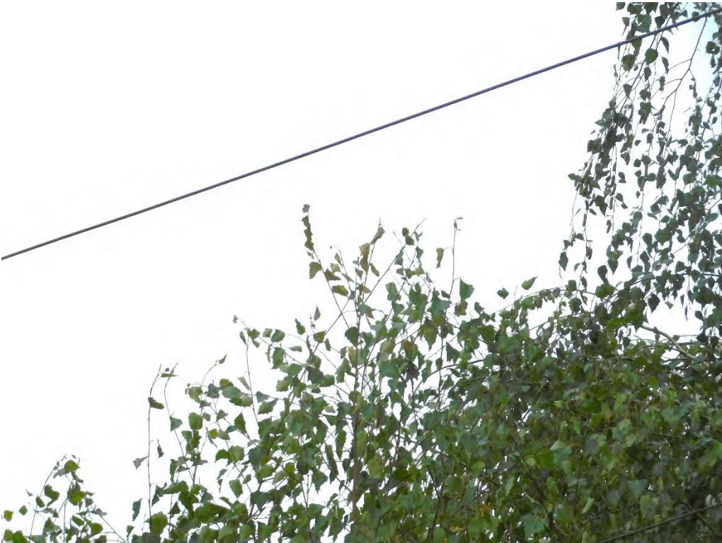
Probable violation B.195: Tree shows evidence of contacting primary conductors at 5411 SE Monroe Street, Portland. (45.4448, -122.6076)
