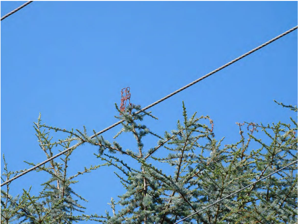
Probable violation B.50: Tree shows evidence of contacting primary conductors at 895 NE Melinda Court, Hillsboro. (45.5389, -122.9755)
