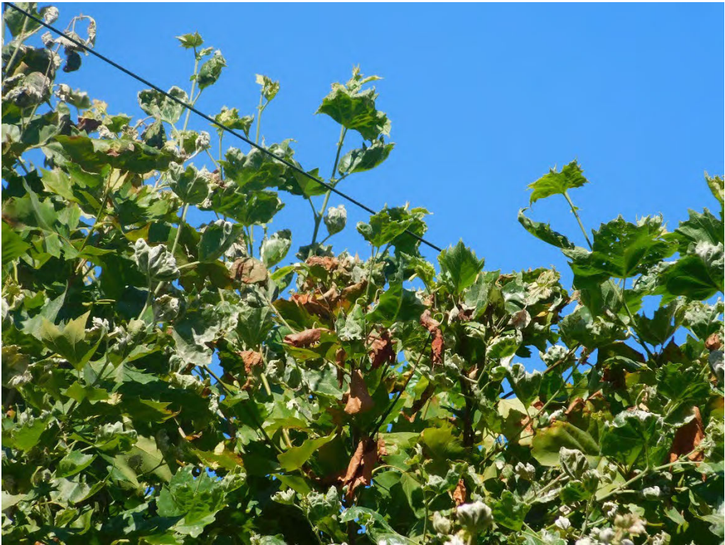
Probable violation B.58: Multiple trees show evidence of contacting the primary conductor behind 1264 NW Summit Avenue, Portland. (45.5323, -122.7083)
