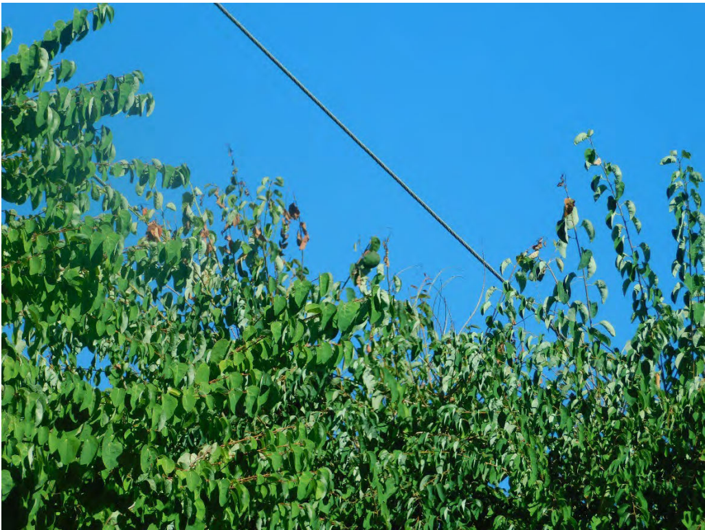
Probable violation B.57: Tree shows evidence of contacting primary conductors at 127 SE Kingston Avenue, Portland. (45.5231, -122.7069)
