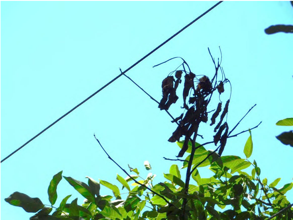
Probable violation B.302: Tree shows evidence of contacting primary conductors at 20337 Pacific Highway East, Aurora. (45.2133, -122.7700)
