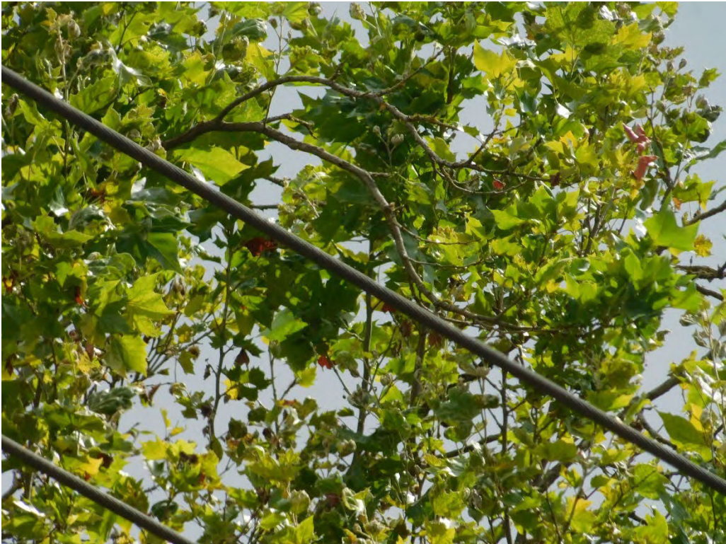
Probable violation B.192: Multiple trees show evidence of contacting the primary conductor the intersection of SE Railroad Avenue and SE Harmony Road, Portland. (45.4324, -122.5997)
