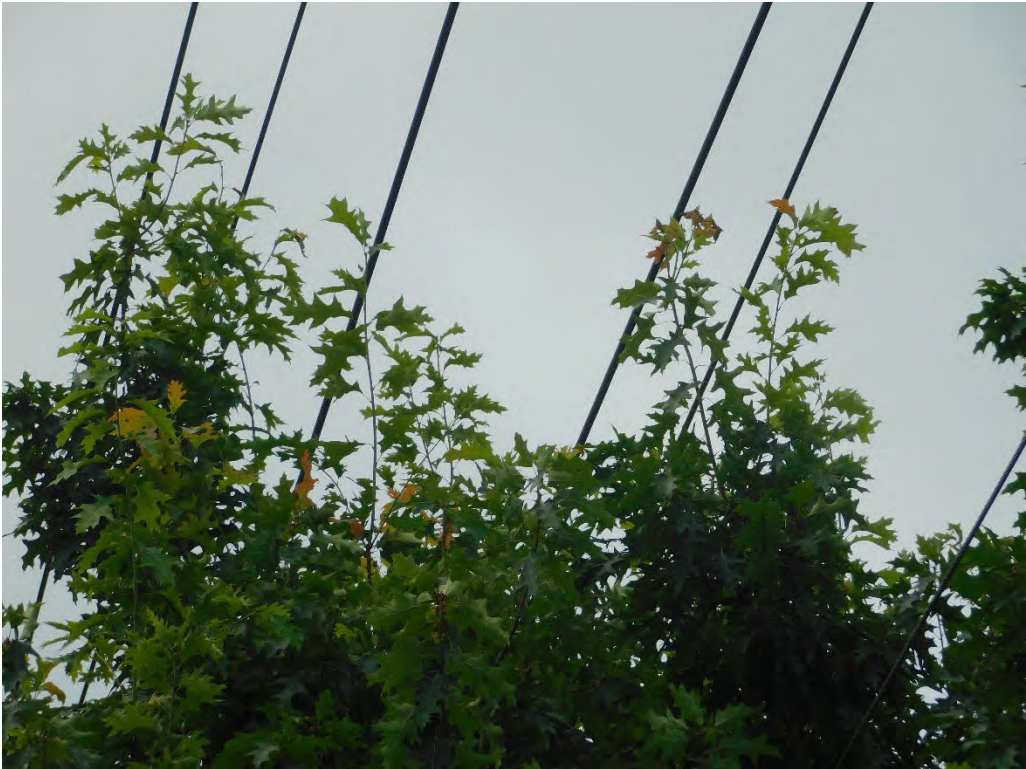
Probable violation B.150: Tree shows evidence of contacting primary conductors at 2096 SE Pinelane Street, Portland. (45.4195, -122.6418)
