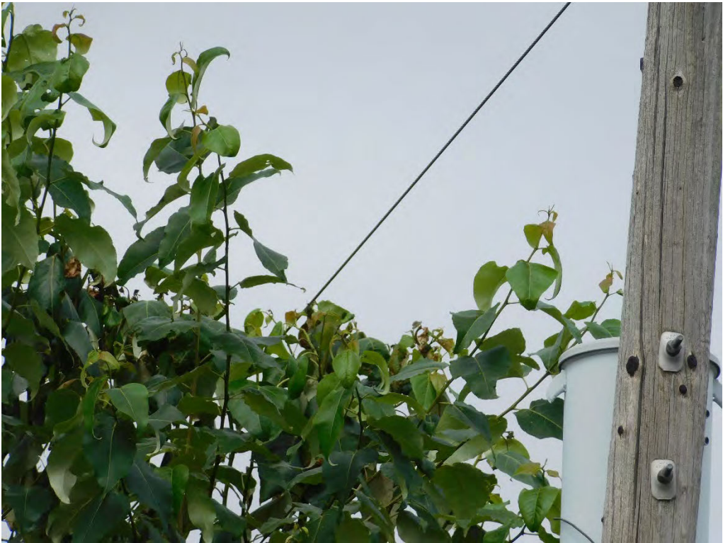
Probable violation B.115: Tree shows evidence of contacting primary conductors at 20395 SW Stafford Street, Tualatin. (45.3722, -122.7051)
