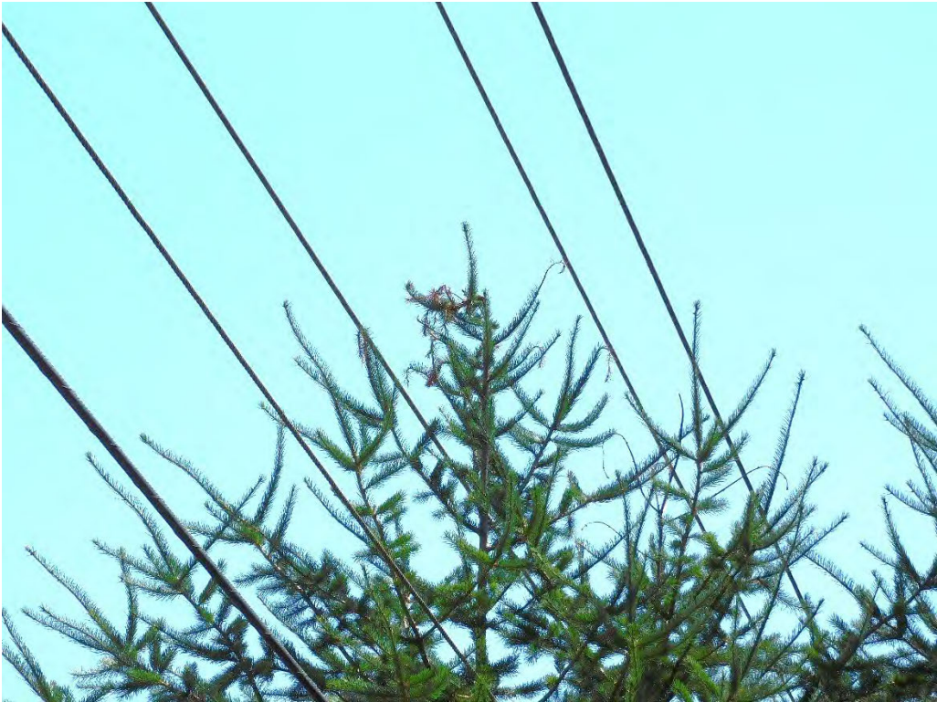
Probable violation B.31: Multiple trees show evidence of contacting the primary conductor on SW Tongue Lane, Cornelius. (45.4838, -123.0480)
