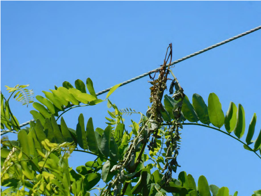
Probable violation B.305: Two trees show evidence of contacting primary conductors at 765 South Pacific Highway, Woodburn. (45.1290, -122.8526)
