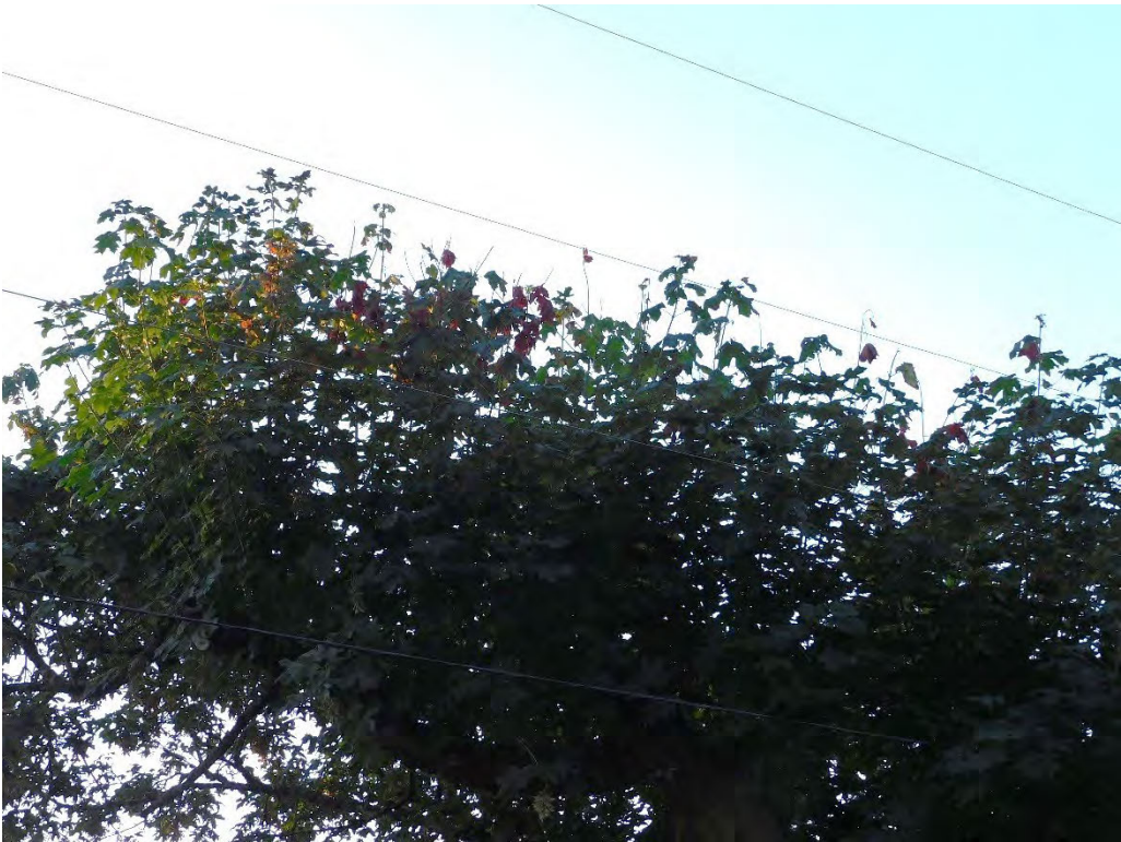
Probable violation B.338: Tree shows evidence of contacting primary conductors at 15618 South Carus Road, Oregon City. (45.2714, -122.5469)
