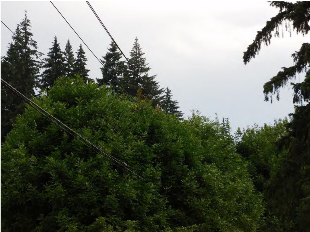
Probable violation B.362: Multiple trees show evidence of contacting primary conductors at 11422 SE Revenue Road, Boring. (45.4411, -122.3315)
