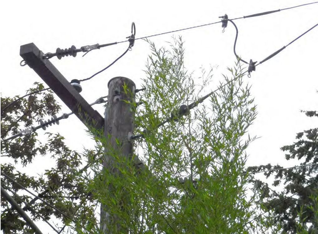
Probable violation B.125: Tree shows evidence of contacting primary conductors at 2991 Glen Haven Road, Lake Oswego (45.4021, -122.7073)
