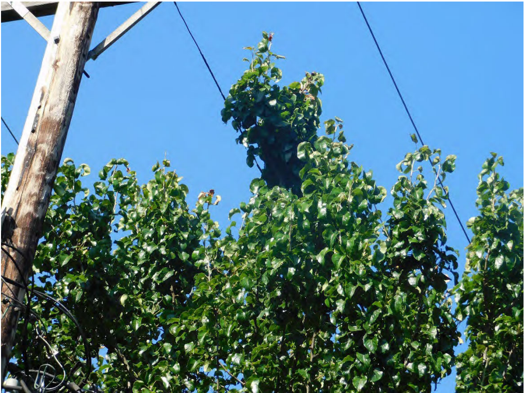
Probable violation B.207: Multiple trees show evidence of contacting the primary conductor at 8940 SE Reedway Street, Portland. (45.4813, -122.5703)
