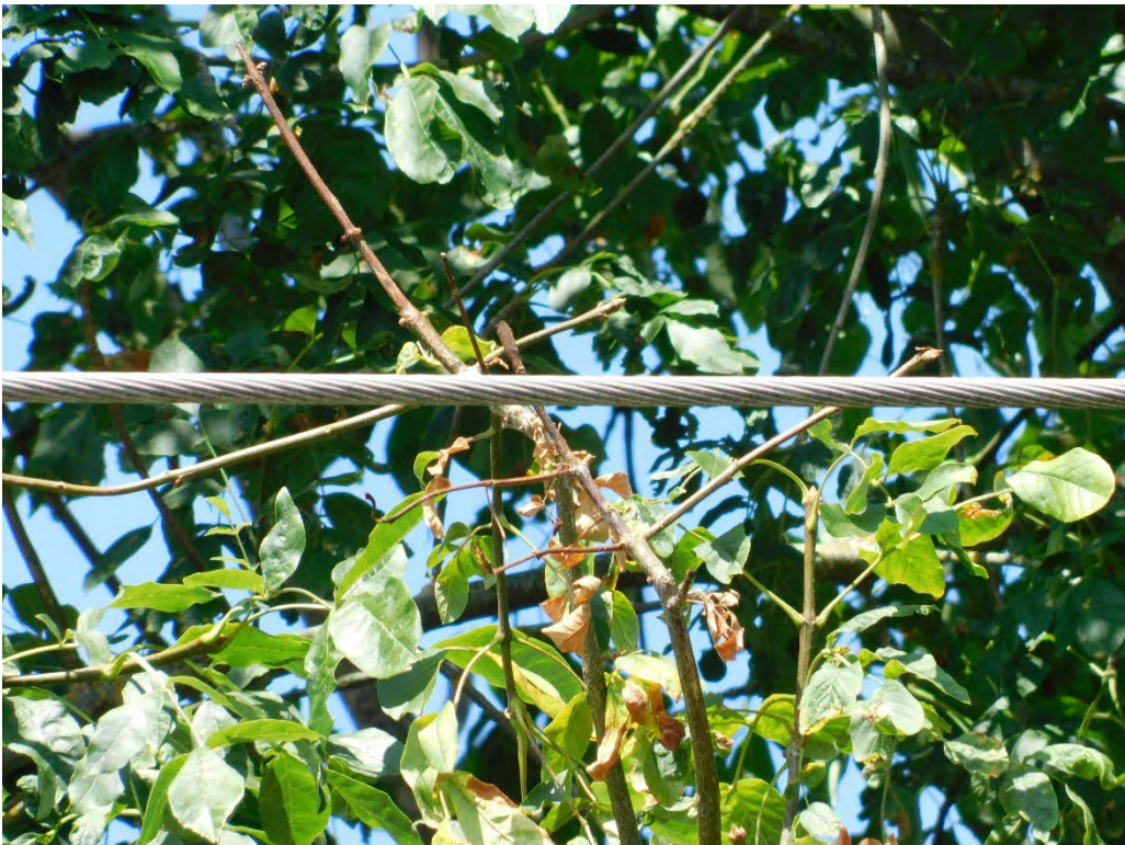
Probable violation B.234: Tree shows evidence of contacting primary conductors on SW Ek Road, West Linn. (45.3670, -122.7054)
