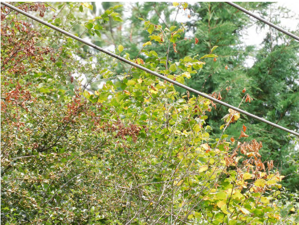
Probable violation B.378: Multiple trees show evidence of contacting primary conductors on SE Clatsop Street, Happy Valley. (45.4614, -122.5195)
