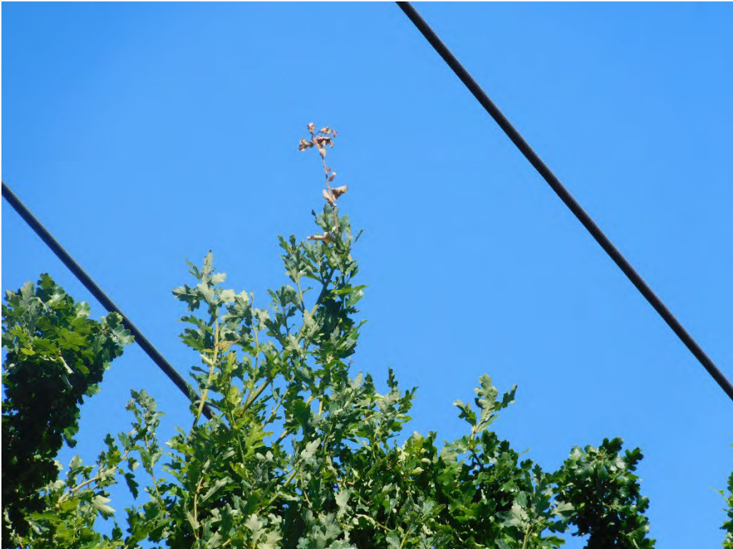
Probable violation B.67: Tree shows evidence of contacting primary conductors at 1137 NW 23 rd Avenue, Portland. (45.5312, -122.6988)
