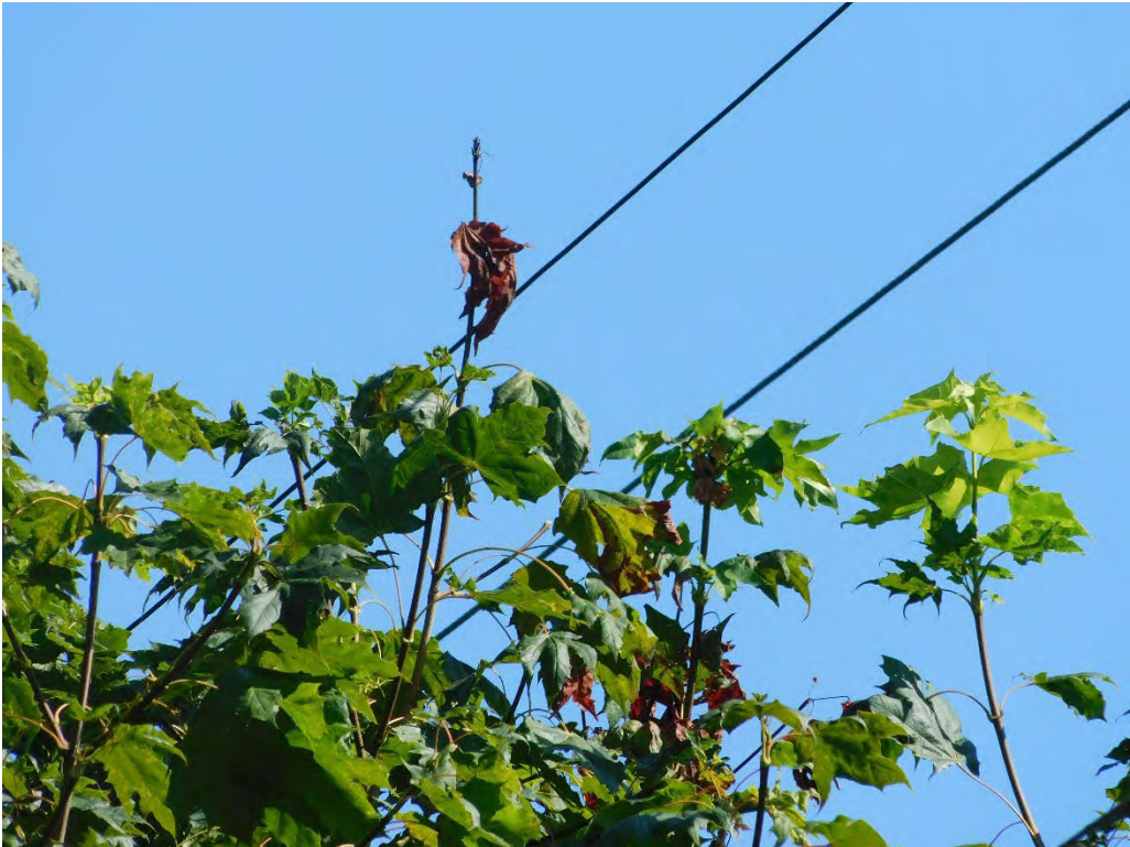
Probable violation B.228: Tree shows evidence of contacting primary conductors across from 5609 SE 48 th Avenue, Portland. (45.4818, -122.6133)
