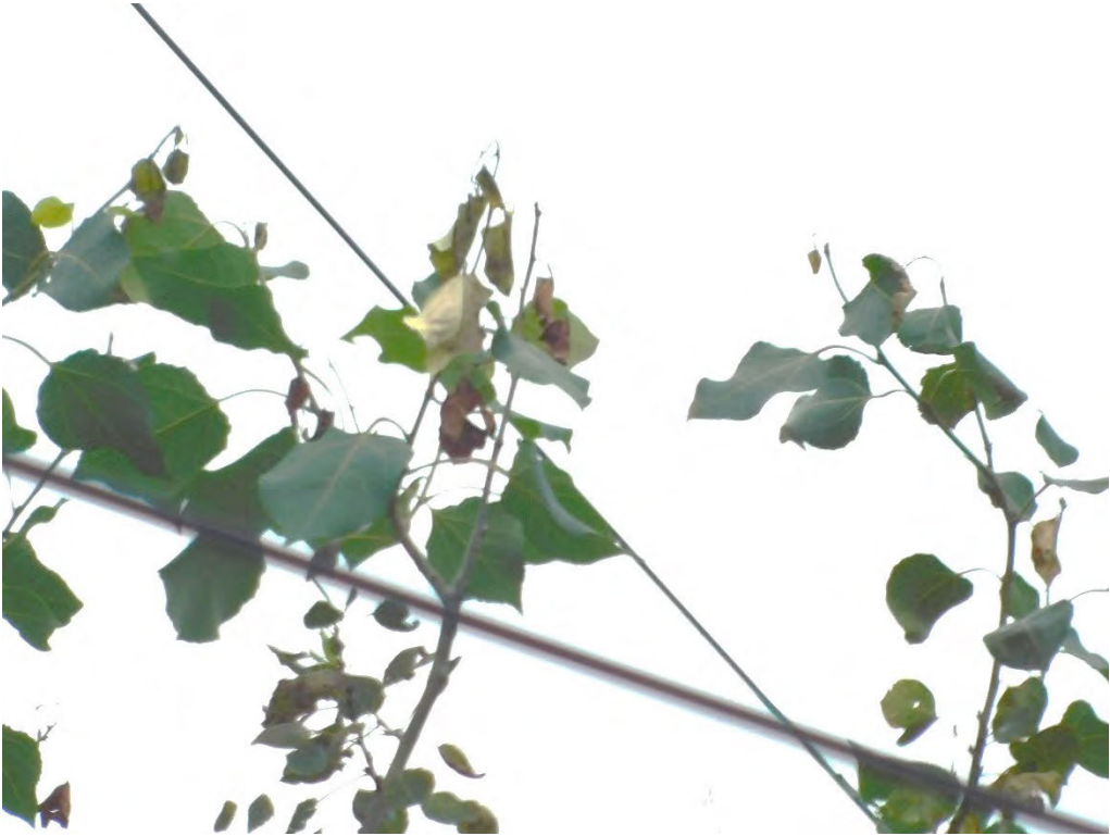
Probable violation B.102: Tree shows evidence of contacting primary conductors at 9711 SW 50 th Avenue, Portland. (45.4552, -122.7285)
