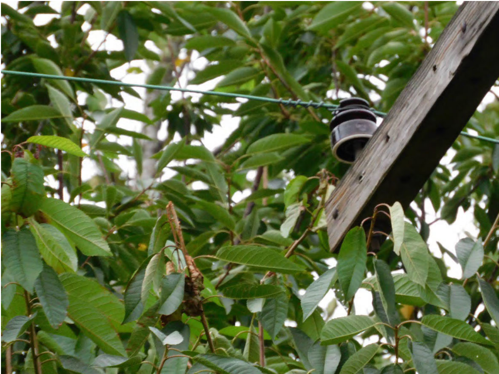
Probable violation B.372: Multiple trees show evidence of contacting primary conductors on SE Ridgeway Drive, Happy Valley. (45.4539, -122.5505)
