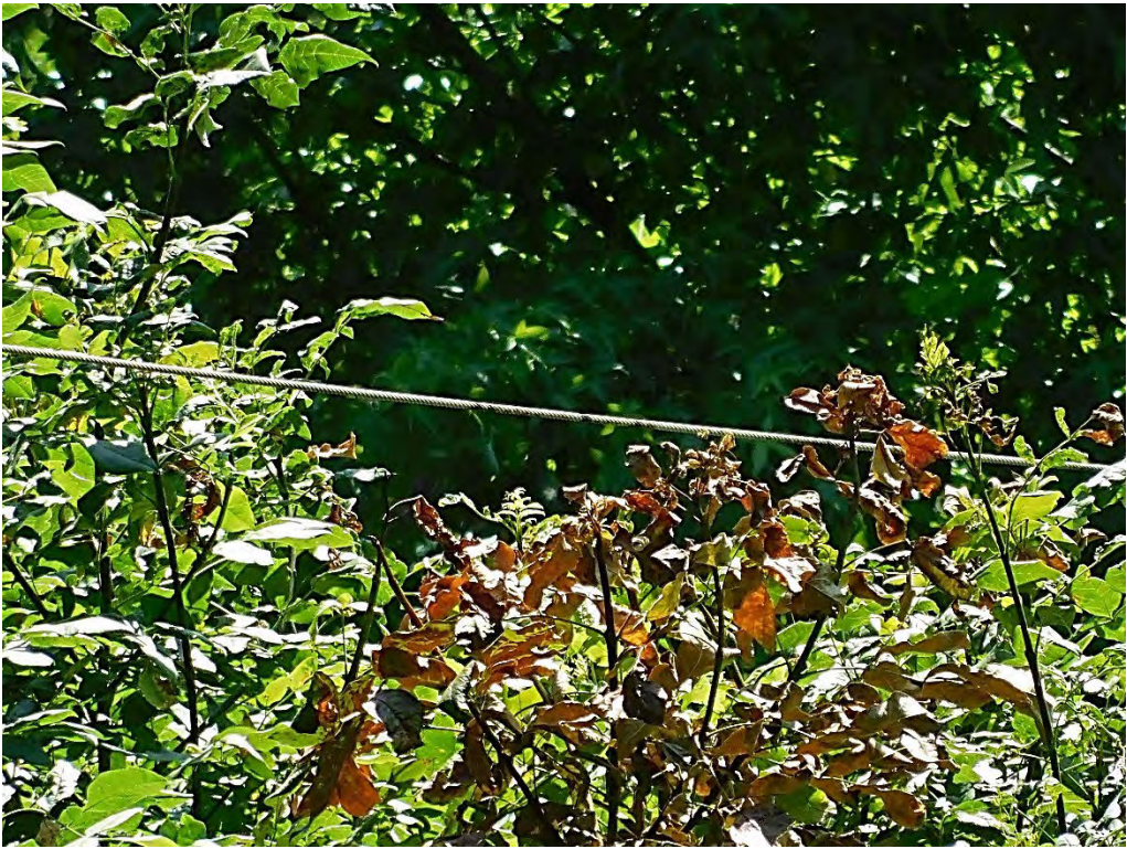
Probable violation B.7: Tree shows evidence of contacting primary conductors at 5089 Riverdale Road South, Salem. (44.8824, -123.1270)
