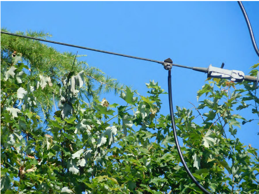
Probable violation B.208: Multiple trees show evidence of contacting the primary conductor at 3223 SE 92 nd Avenue, Portland. (45.4988, -122.5684)
