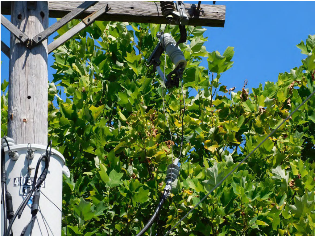
Probable violation B.52: Tree shows evidence of contacting primary conductors at 211 NW Gina Way, Beaverton. (45.5216, -122.8878)
