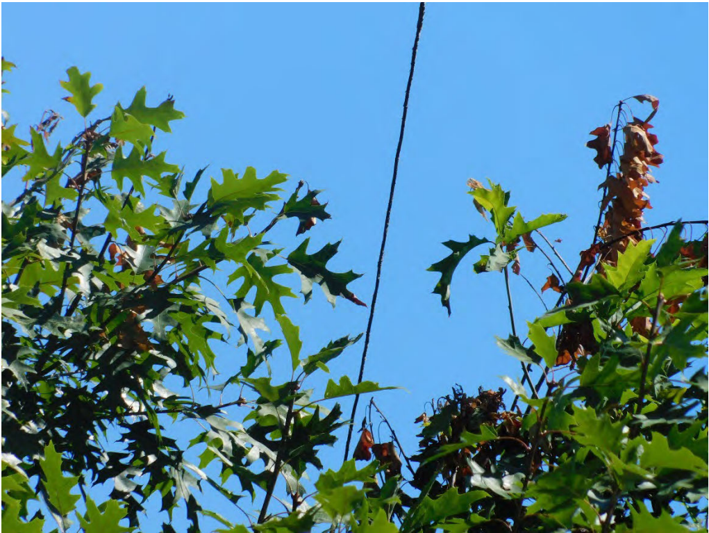
Probable violation B.70: Multiple trees show evidence of contacting the primary conductor at 2066 NW Pettygrove Street, Portland. (45.5327, -122.6942)
