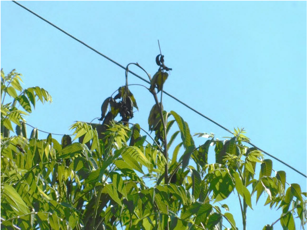
Probable violation B.310: Tree shows evidence of contacting primary conductors at 14985 Woodburn/Monitor Road NE, Woodburn. (45.1021, -122.7528)
