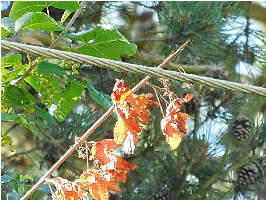
Probable violation B.8: Tree shows evidence of contacting primary conductors on River Road South, Salem. (44.9021, -123.1019)
