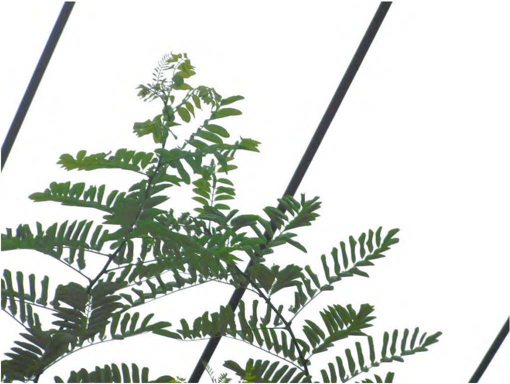
Probable violation B.90: Tree shows evidence of contacting primary conductors across from 7333 SW Pine Street, Tigard. (45.4433, -122.7533)
