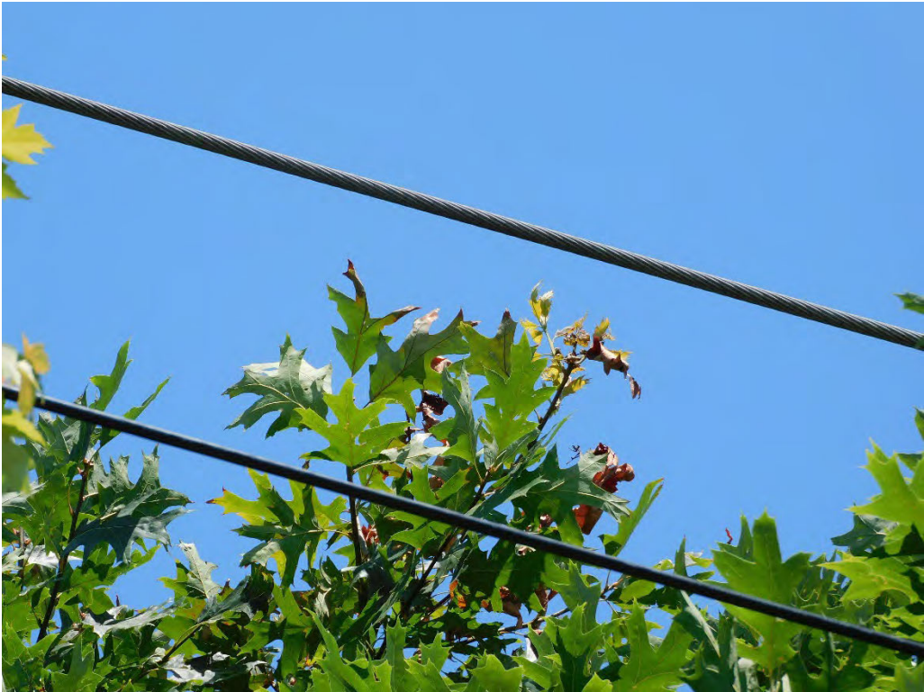
Probable violation B.29: Tree shows evidence of contacting primary conductors on SW Beef Bend Road, Portland. (45.4018, -122.8299)
