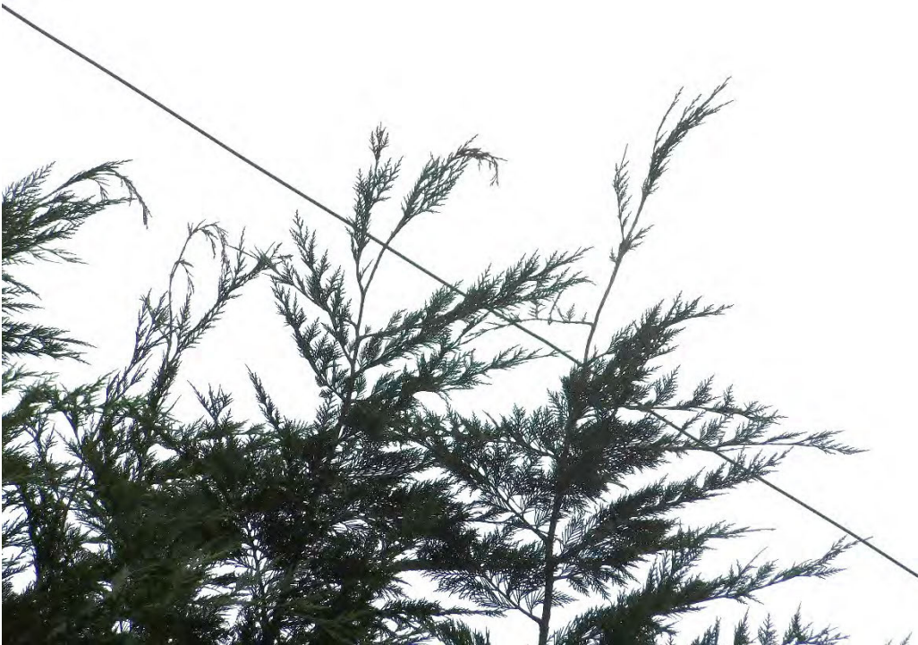
Probable violation B.156: Tree shows evidence of contacting primary conductors at 3310 SE Westview Road, Portland. (45.4060, -122.6283)
