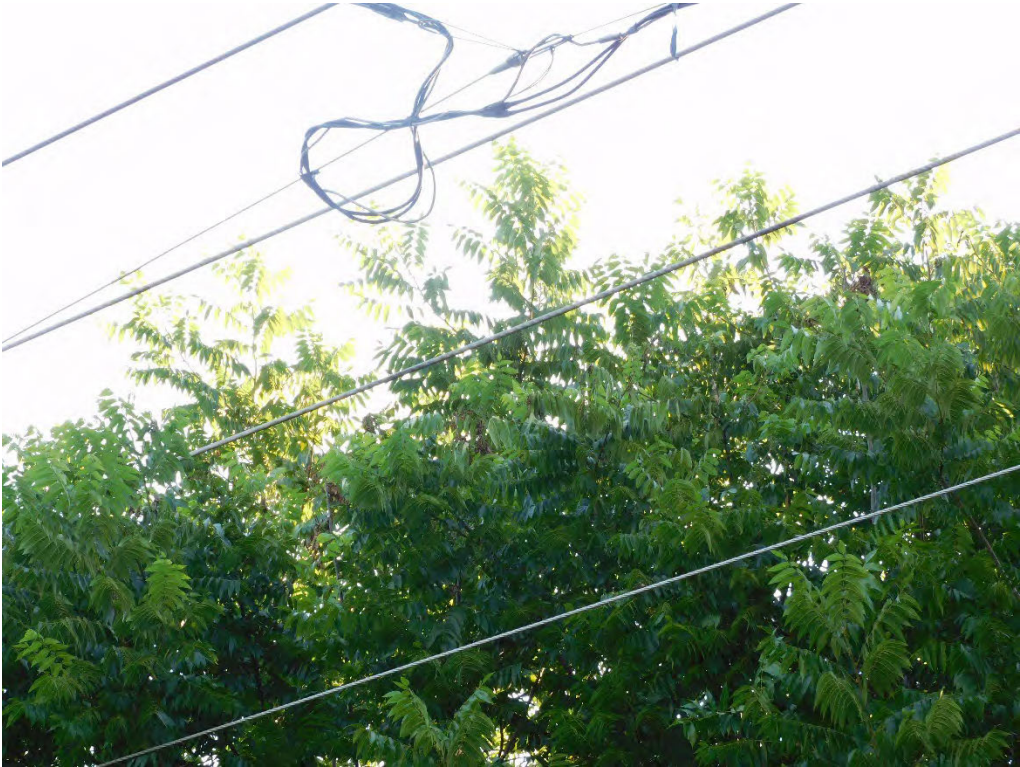
Probable violation B.30: Tree shows evidence of contacting primary conductors at 630 SW Dennis Avenue, Hillsboro. (45.5157, -122.9958)
