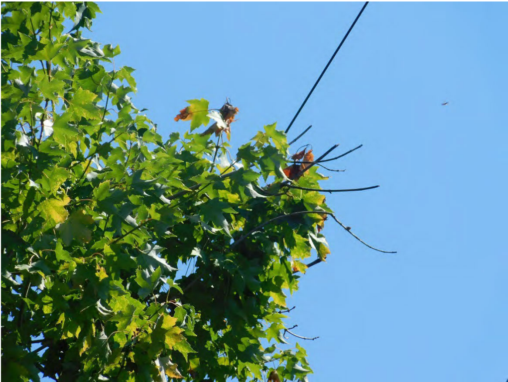
Probable violation B.221: Tree shows evidence of contacting primary conductors at 3808 SE Henry Street, Portland. (45.4762, -122.6233)
