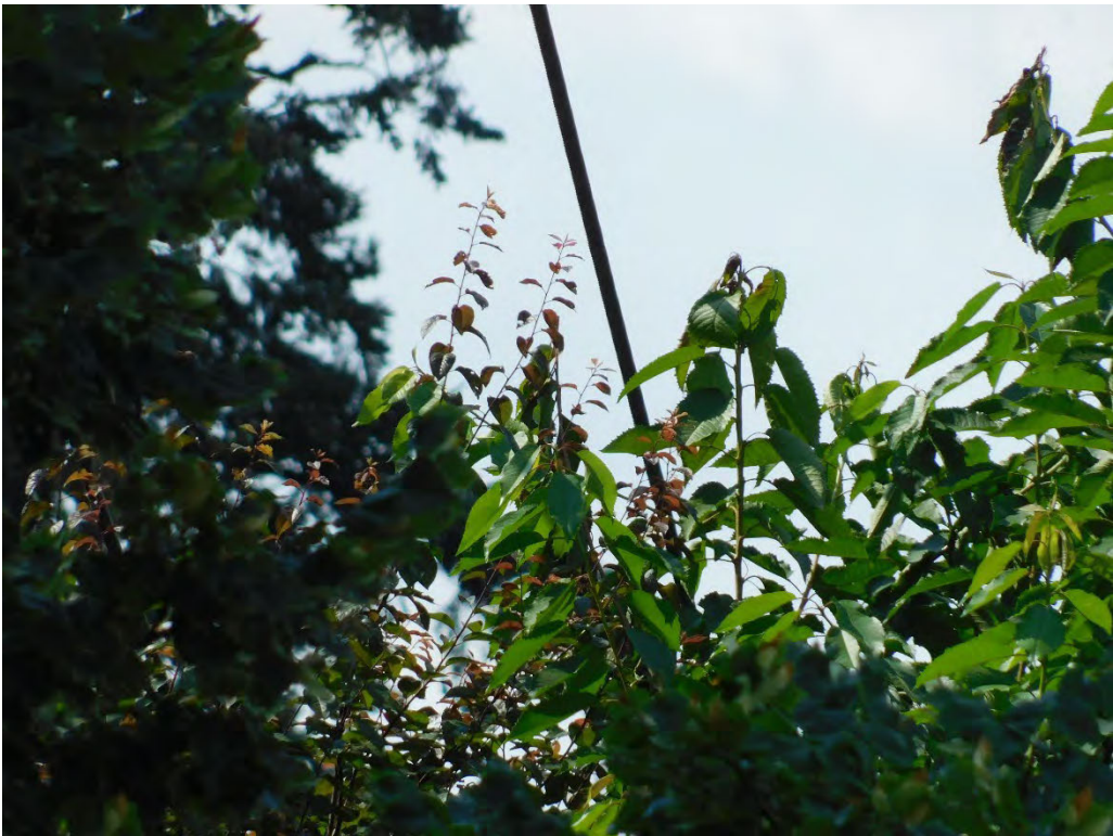
Probable violation B.267: Tree shows evidence of contacting primary conductors at 4410 Cordon Road NE, Salem. (44.9854, -122.9552)
