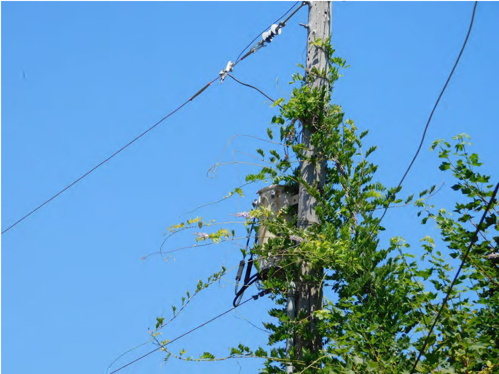
Probable violation C.2: Vines engulfing pole and approaching primary conductor are creating a hazard at 12473 Ferry Road NE, Aurora. (45.2132, -122.8056)
