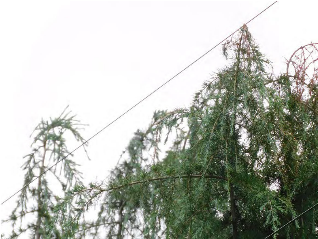
Probable violation B.36: Tree shows evidence of contacting primary conductors at 38760 NW Harrison Road, Banks. (45.6216, -123.0760)
