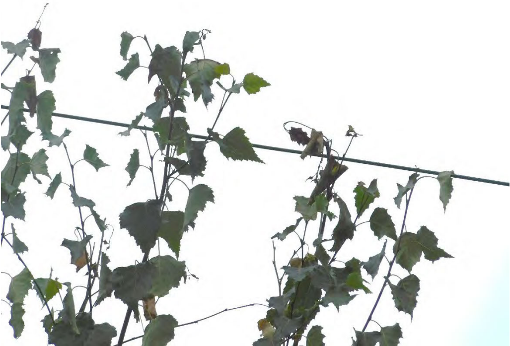
Probable violation B.99: Tree shows evidence of contacting primary conductors at 9529 SW 62 nd Drive, Portland. (45.4571, -122.7391)
