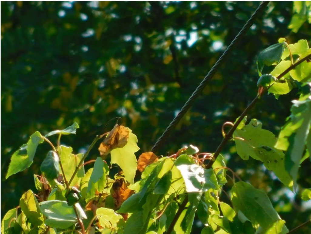
Probable violation B.14: Tree shows evidence of contacting primary conductors at 1340 Nebraska Avenue NE, Salem. (44.9472, -123.0193)
