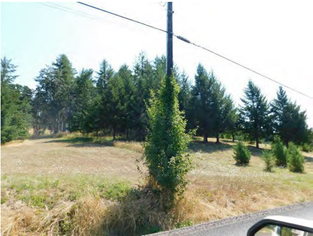
Probable violation C.14: Vines engulfing pole are creating a climbing hazard on SW Golpher Valley Road, Sheridan. (45.1694, -123.3783)
