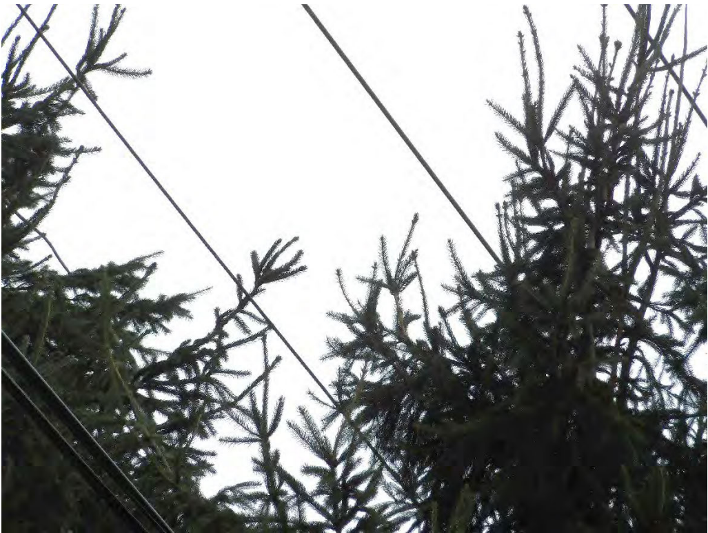
Probable violation B.118: Tree shows evidence of contacting primary conductors at 2100 SW Borland Road, Tualatin. (45.3691, -122.6972)
