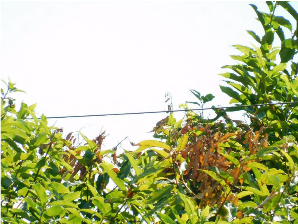
Probable violation A.5: Hazard: Two readily climbable trees show evidence of contacting the primary conductor at 22281 SW 55 th Avenue, Tualatin. (45.3588, -122.7330)
