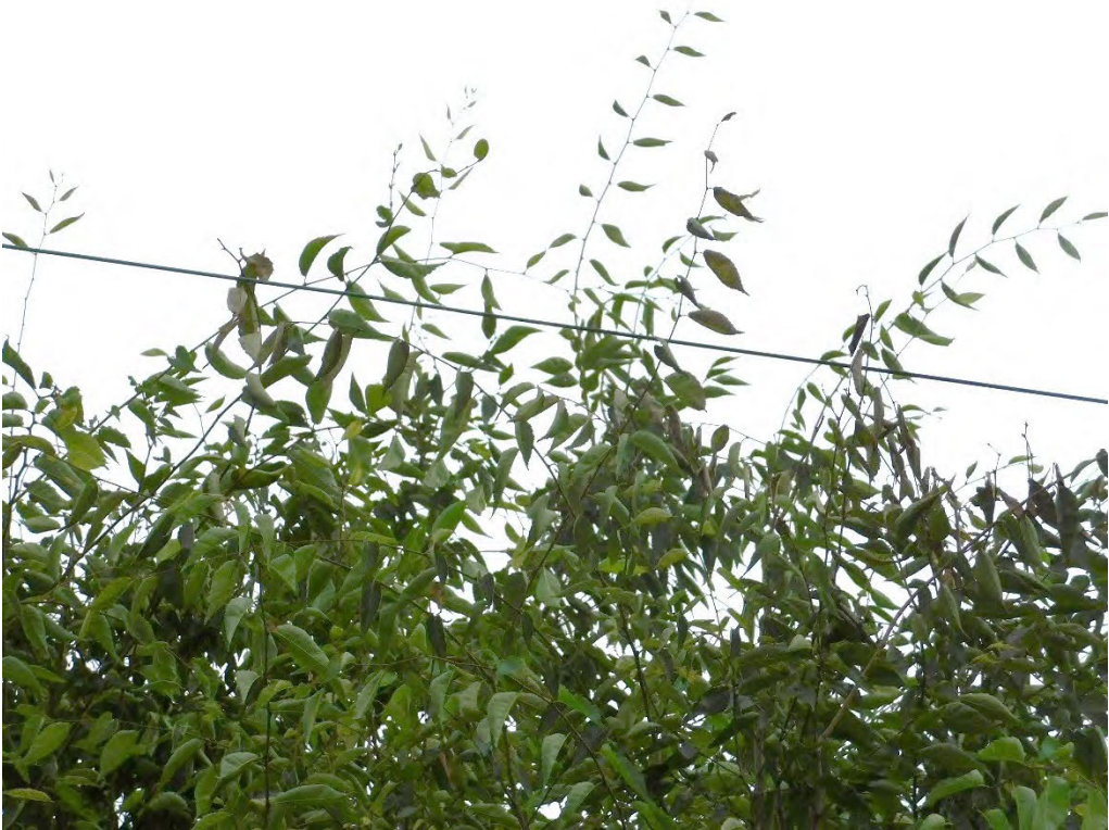
Probable violation B.175: Multiple trees show evidence of contacting the primary conductor at 7919 SE Sunnyside Drive, Portland. (45.4337, -122.5807)
