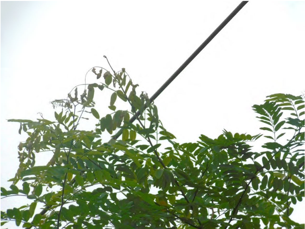
Probable violation B.92: Tree shows evidence of contacting primary conductors at 6571 SW Taylors Ferry Road, Portland. (45.4550, -122.7443)
