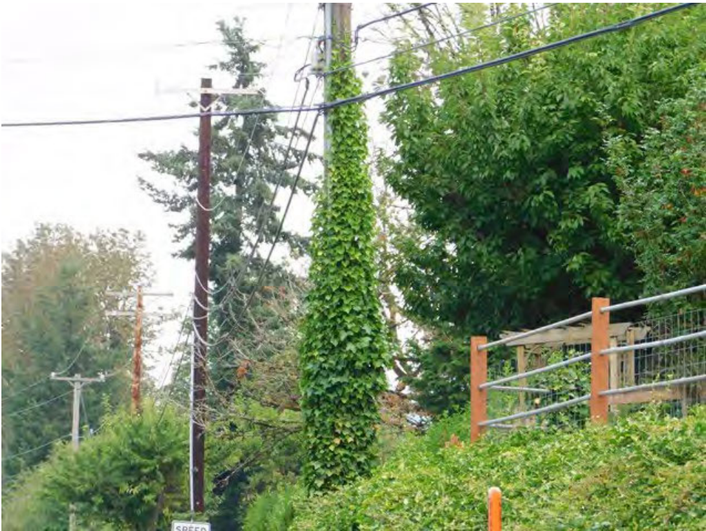
Probable violation C.12: Vines engulfing pole are creating a climbing hazard on SW Mountain Road, West Linn. (45.3536, -122.7098)
