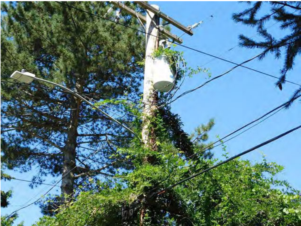
Probable violation C.22: Vines engulfing pole and approaching primary conductor are creating a hazard at 3539 SW Nevada Court, Portland. (45.4726, -122.7134)
