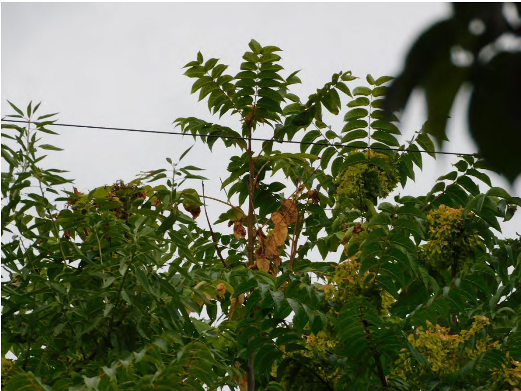
Probable violation B.332: Tree shows evidence of contacting primary conductors at 507 3rd Street, Oregon City. (45.3537, -122.6087)
