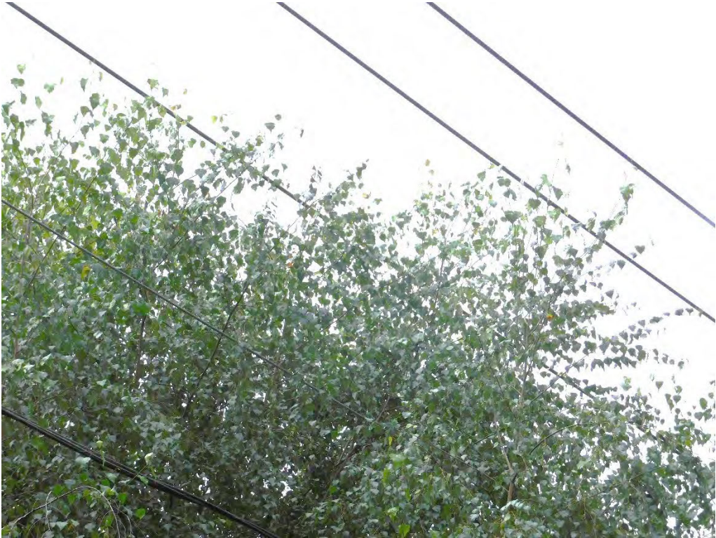
Probable violation B.201: Tree shows evidence of contacting primary conductors at 4016 SE Rosewell Street, Portland. (45.4584, -122.6220)
