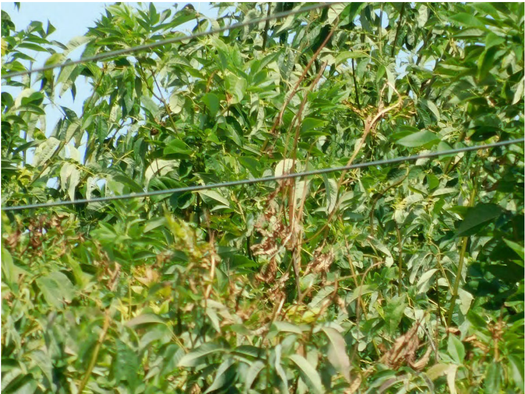
Probable violation A.10: Hazard: Multiple readily climbable trees show evidence of contacting the primary conductor at 1555 SW Borland Road, West Linn. (45.3654, -122.6925)
