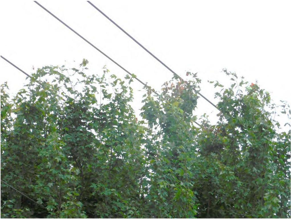
Probable violation B.197: Tree shows evidence of contacting primary conductors at 3902 SE King Street, Portland. (45.4480, -122.6229)
