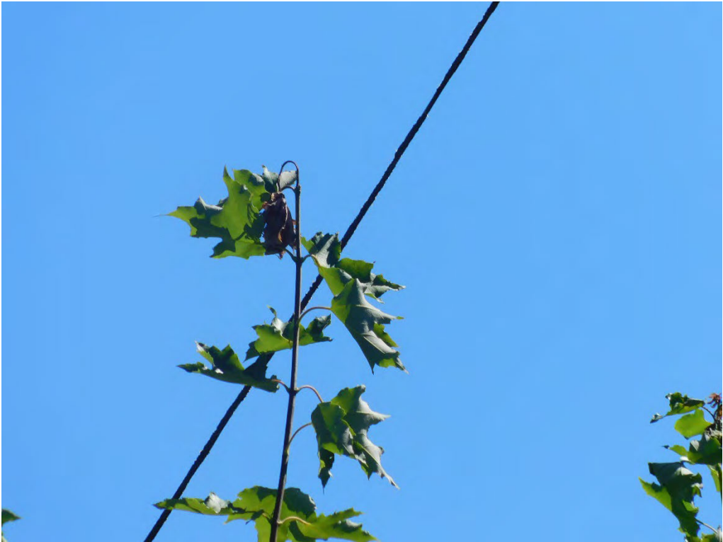
Probable violation B.72: Tree shows evidence of contacting primary conductors at 2926 NW Raleigh Street, Portland. (45.5338, -122.7115)
