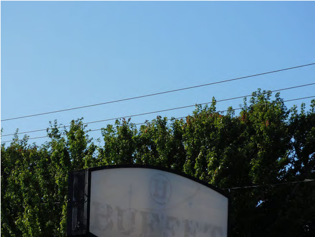
Probable violation B.44: Two trees show evidence of contacting the primary conductor at 1050 SW Baseline Street, Hillsboro. (45.5191, -123.0017)
