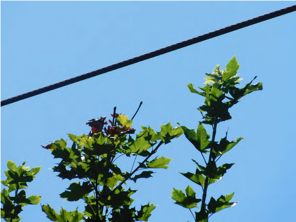
Probable violation B.222: Multiple trees show evidence of contacting the primary conductor at 6025 SE 34 th Avenue, Portland. (45.4789 -122.6283)
