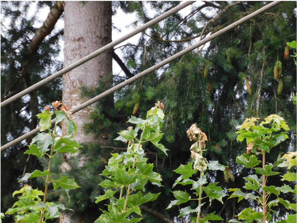
Probable violation B.363: Two trees show evidence of contacting primary conductors at 10905 SE Revenue Road, Boring. (45.4438, -122.3322)
