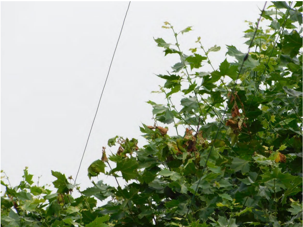
Probable violation B.244: Multiple trees show evidence of contacting the primary conductor on Volpp Street, West Linn. (45.3393, -122.6502)
