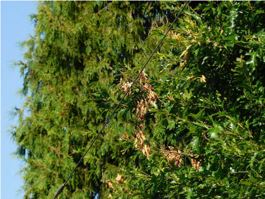
Probable violation B.49: Tree shows evidence of contacting primary conductors at 1549 NE Jackson School Road, Hillsboro. (45.5361, -122.9801)
