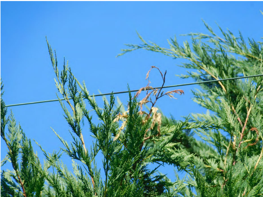
Probable violation B.132: Tree shows evidence of contacting primary conductors at 5035 SE Glen Echo Avenue, Portland. (45.3830, -122.6112)
