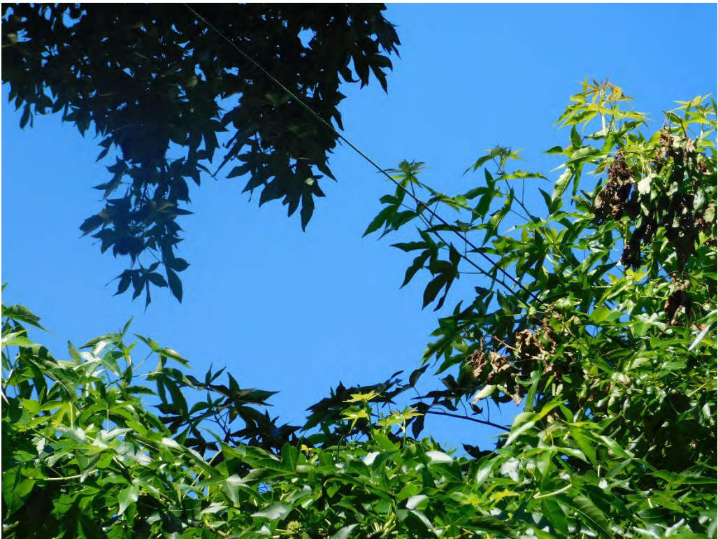
Probable violation B.59: Multiple trees show evidence of contacting the primary conductor at 2682 NW Cornell Road, Portland. (45.5313, -122.7068)
