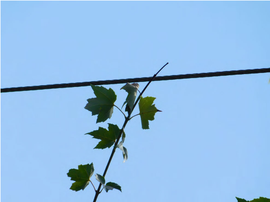
Probable violation A.4: Hazard: Readily climbable tree shows evidence of contacting the primary conductor at 5870 SW Delker Road, Tualatin. (45.3609, -122.7373)
