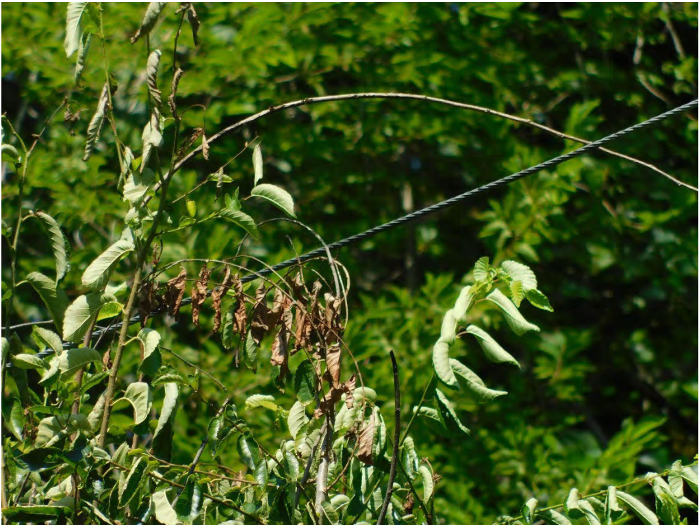
Probable violation B.233: Multiple trees show evidence of contacting the primary conductor at 6121 SE 32 nd Avenue, Portland. (45.4780, -122.6311)
