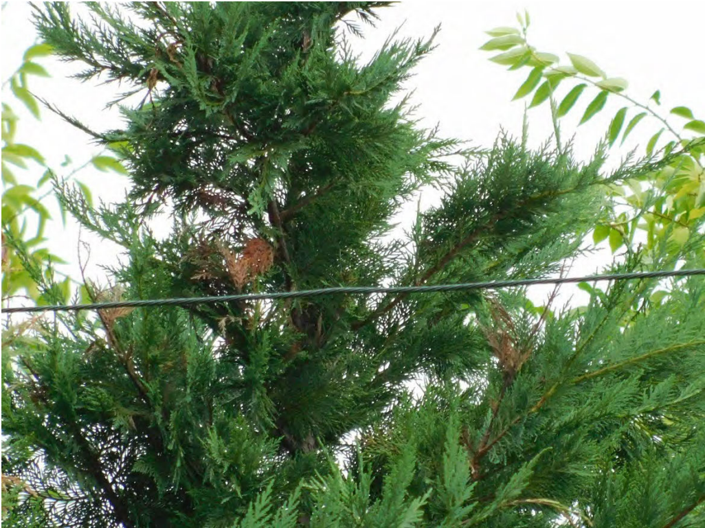
Probable violation B.26: Tree shows evidence of contacting primary conductors at 1038 Hwy 47, Carlton. (45.2872, -123.1748)
