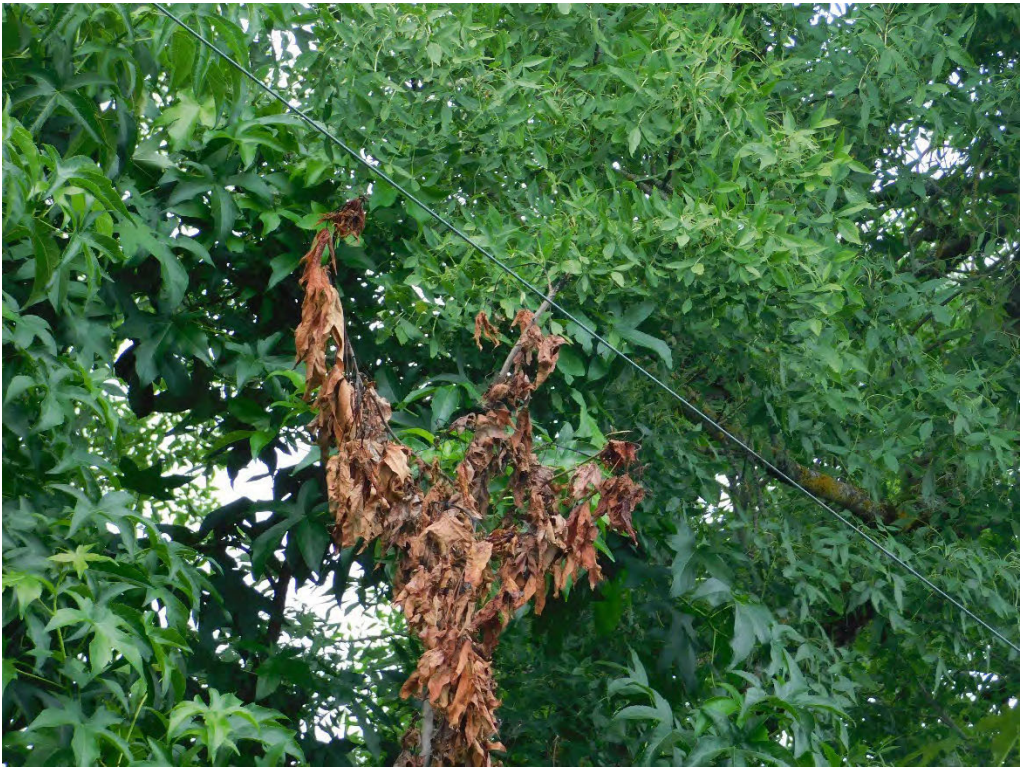
Probable violation B.189: Tree shows evidence of contacting primary conductors at 7245 SE Harmony Drive, Portland. (45.4411, -122.5883)
