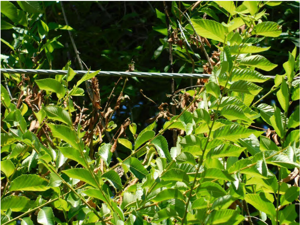
Probable violation B.322: Tree shows evidence of contacting primary conductors at 29444 South Salo Road, Mulino. (45.1799, -122.5229)
