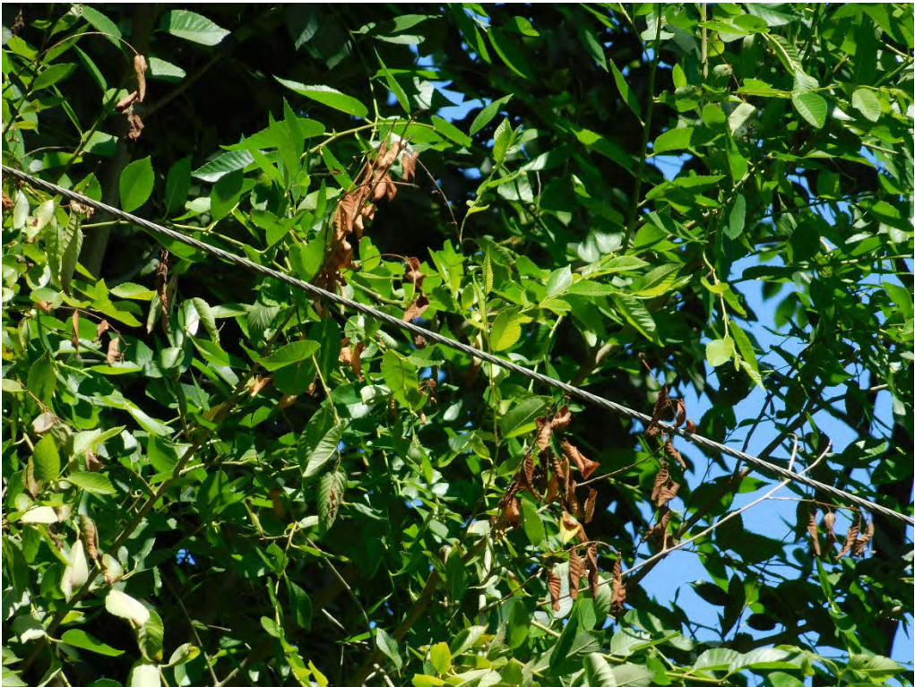
Probable violation B.324: Tree shows evidence of contacting primary conductors at 15704 South Windy City Road, Mulino. (45.1941, -122.5416)
