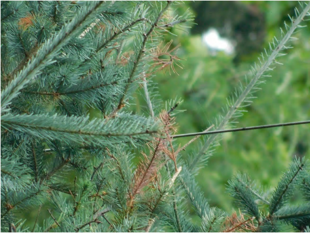
Probable violation B.328: Tree shows evidence of contacting primary conductors at 23939 SW Gage Road, Wilsonville. (45.3472, -122.7305)
