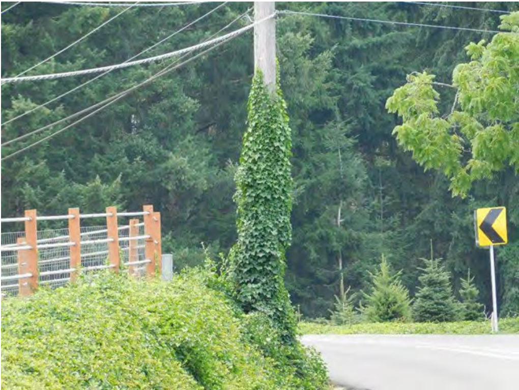
Probable violation C.13: Vines engulfing pole are creating a climbing hazard on SW Schaeffer Road, West Linn. (45.3527, -122.7088)
