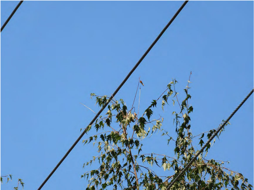
Probable violation B.32: Tree shows evidence of contacting primary conductors at 36260 SW Tongue Lane, Cornelius. (45.4838, -123.0498)
