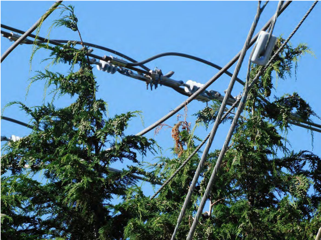
Probable violation B.47: Two trees show evidence of contacting the primary conductor at 1485 NE Sunrise Lane, Hillsboro. (45.5367, -122.9665)
