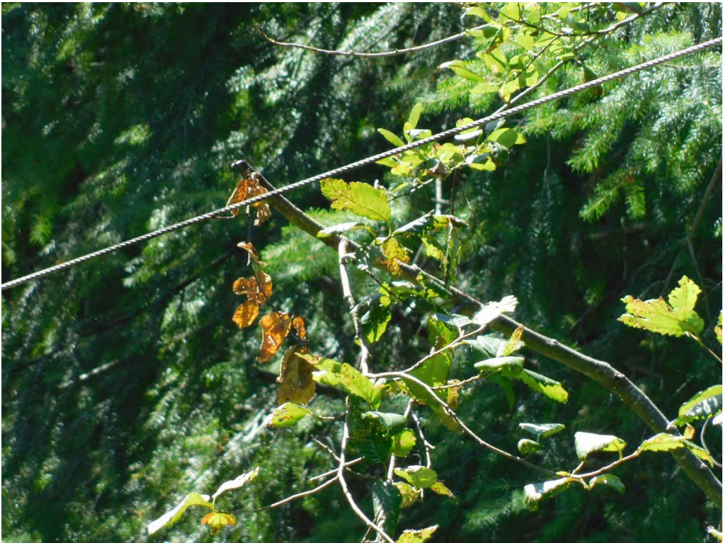
Probable violation B.88: Tree shows evidence of contacting primary conductors on NW Skyline Blvd., Portland. (45.6689, -122.9109) HFRZ
