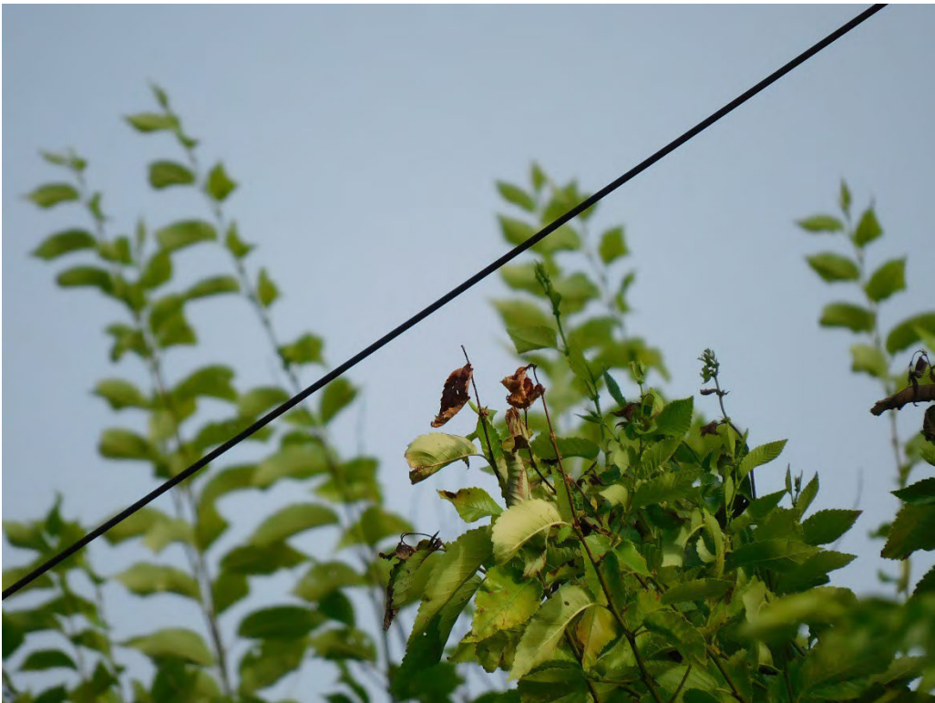
Probable violation B.35: Tree shows evidence of contacting primary conductors at 46633 NW Sell Road, Banks. (45.4849, -123.0141)
