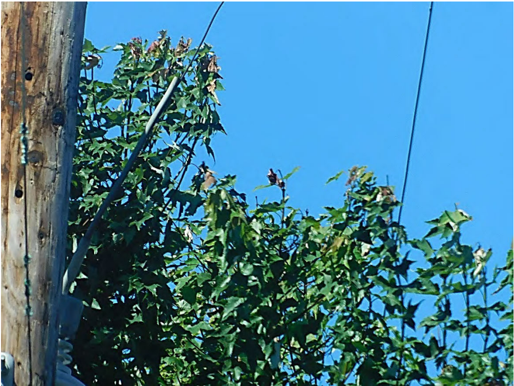
Probable violation B.62: Multiple trees show evidence of contacting the primary conductor at 2250 NW Kearny Street, Portland. (45.5290, -122.6976)
