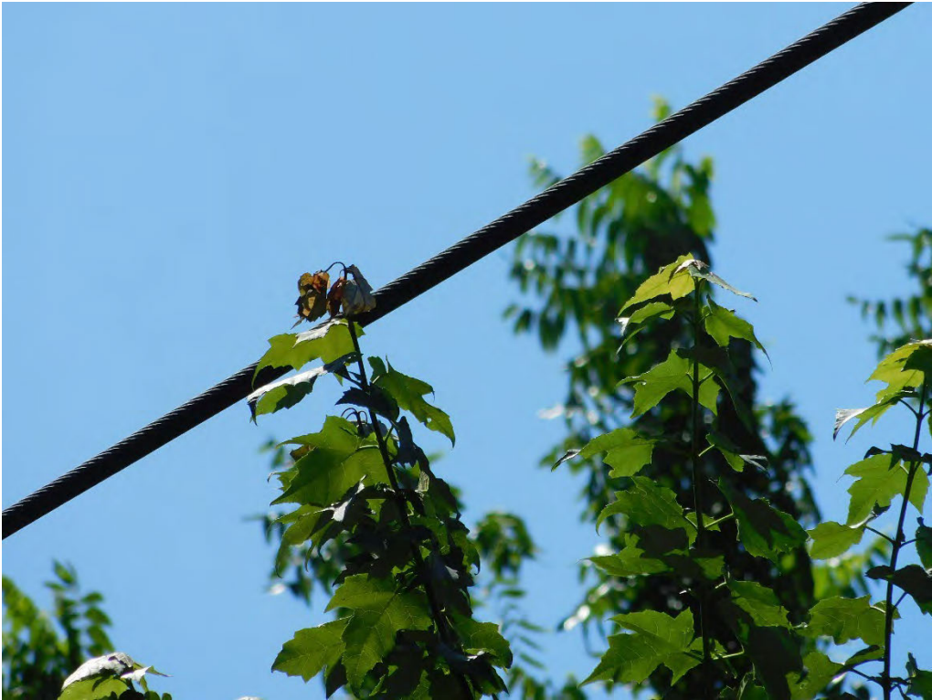
Probable violation B.304: Tree shows evidence of contacting primary conductors at 531 Doud Street, Woodburn. (45.1427, -122.8535)
