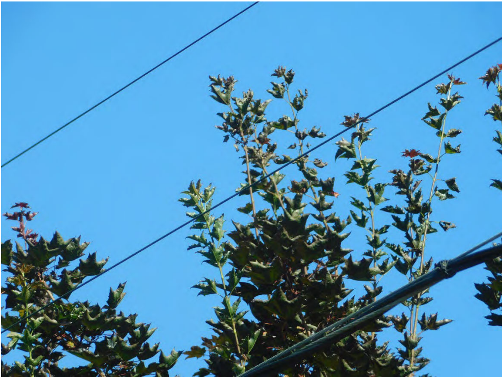
Probable violation B.288: Two trees show evidence of contacting primary conductors at 4433 Dover Avenue NE, Salem. (45.0185, -122.9718)
