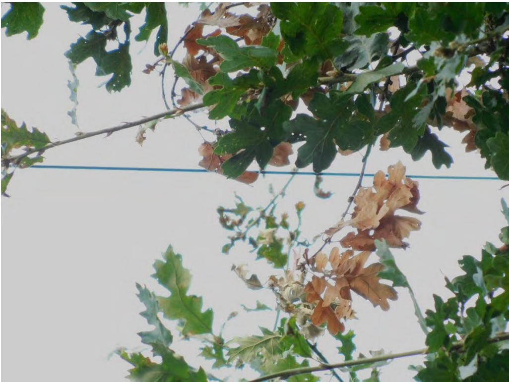
Probable violation B.327: Tree shows evidence of contacting primary conductors on SW Newland Road, Wilsonville. (45.3507, -122.7227)
