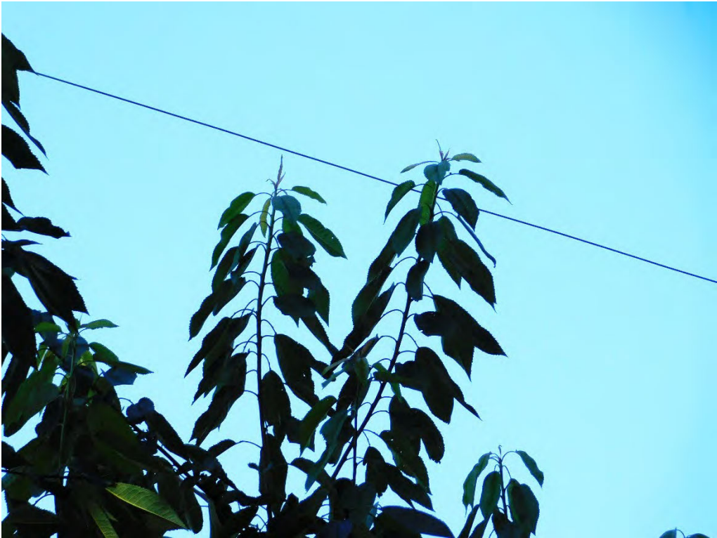
Probable violation B.286: Tree shows evidence of contacting primary conductors at 7296 54th Avenue NE, Salem. (45.0243, -122.9513)
