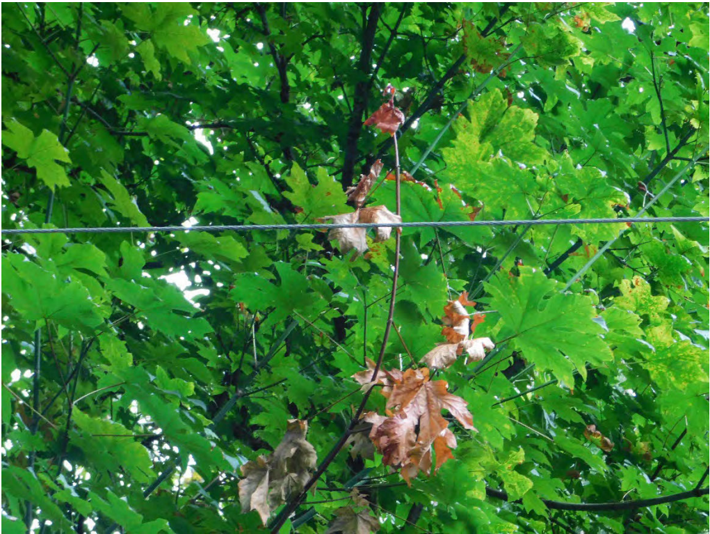
Probable violation B.237: Tree shows evidence of contacting primary conductors on SW Turner Road, West Linn. (45.3592, -122.6954)
