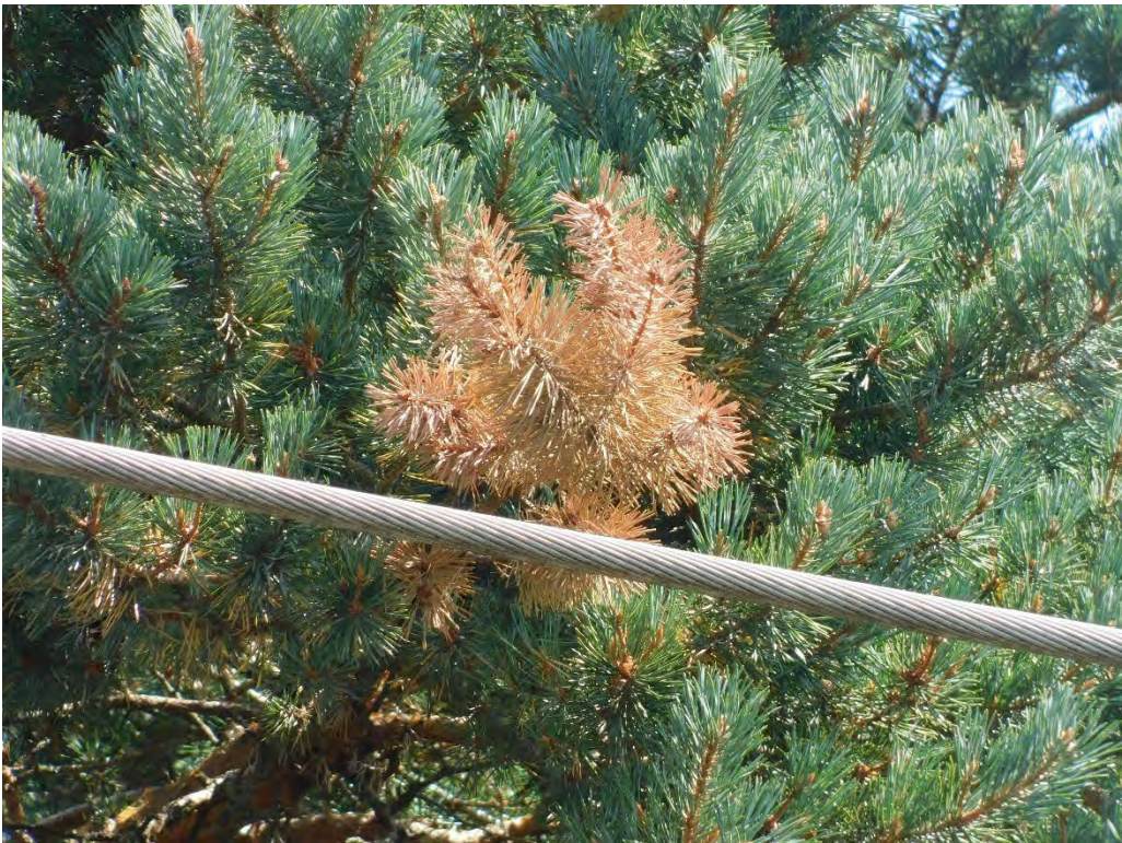
Probable violation B.162: Tree shows evidence of contacting primary conductors at 15318 SE Outfield Road, Portland. (45.4117 , -122.6217)
