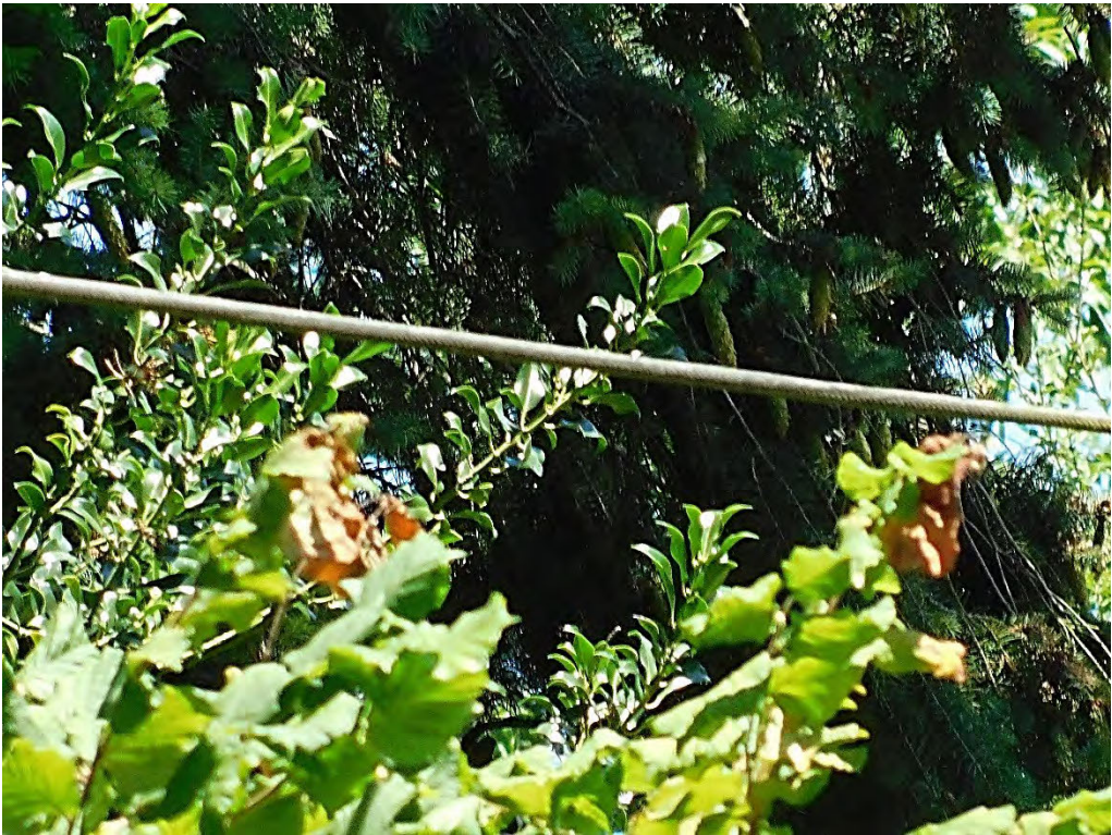
Probable violation B.23: Tree shows evidence of contacting primary conductors on NE Boones Ferry Road, Aurora. (45.2868, -122.7751)
