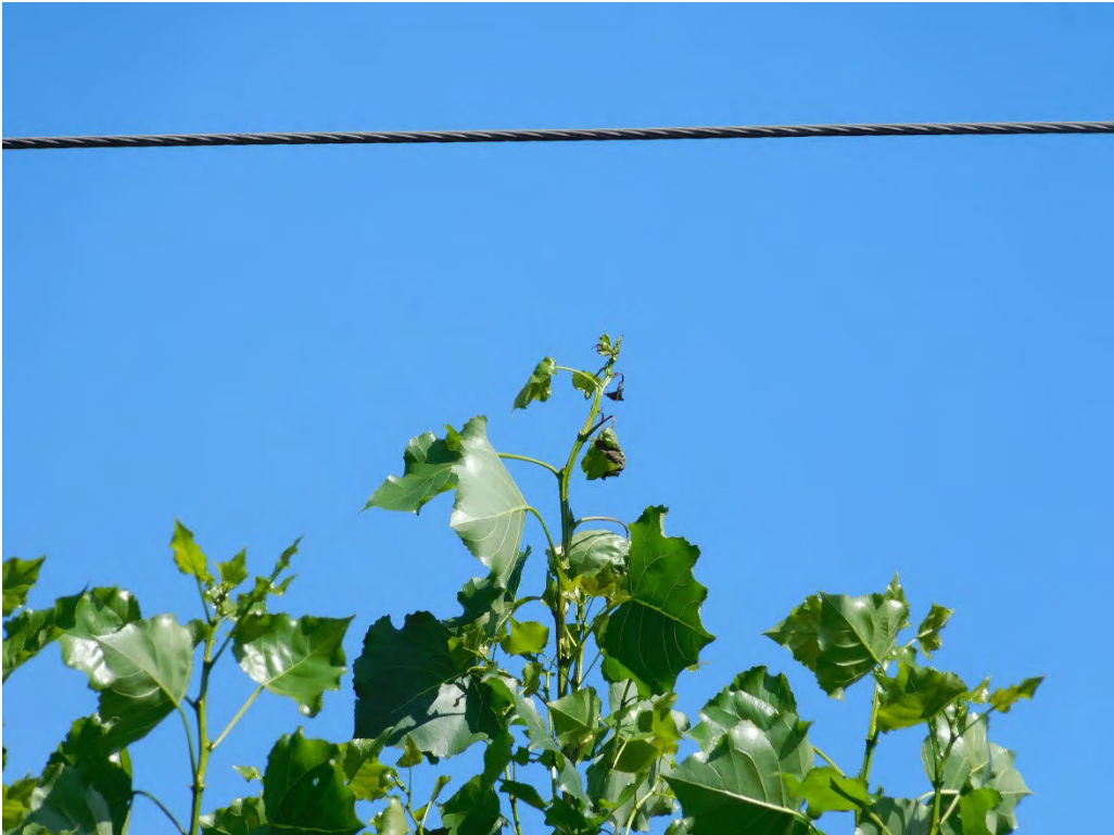
Probable violation B.297: Tree shows evidence of contacting primary conductors across from 9344 Mount Angel/Gervais Road, Gervais. (45.0932, -122.8710)
