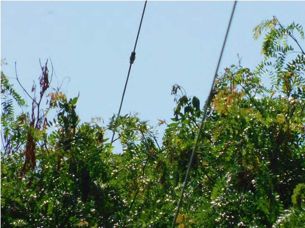
Probable violation B.311: Tree shows evidence of contacting primary conductors at 14779 South Vaughan Road, Molalla. (45.1596, -122.5639)
