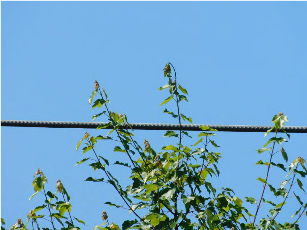
Probable violation B.259: Multiple trees show evidence of contacting primary conductors at 3925 Lancaster Drive NE, Salem. (44.9762, -122.9836)
