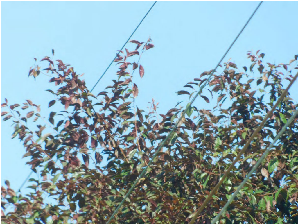
Probable violation B.289: Tree shows evidence of contacting primary conductors at 4251 Webb Avenue NE, Salem. (45.0177, -122.9753)
