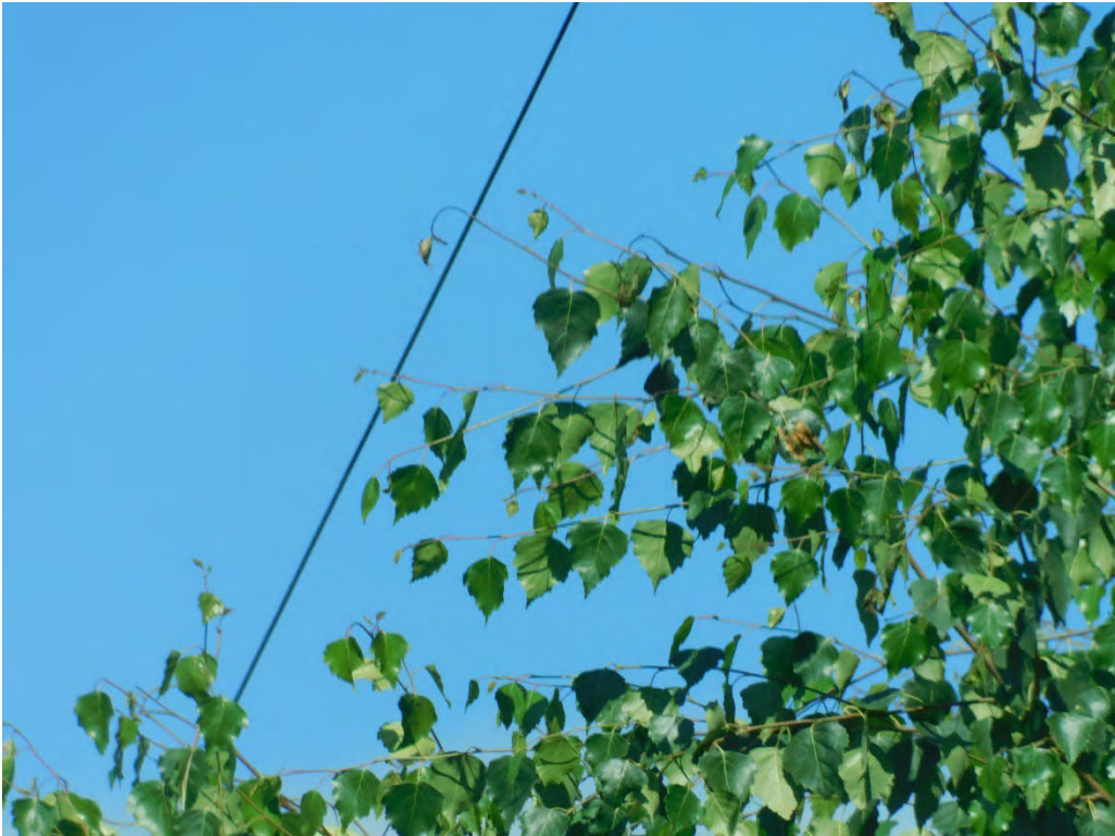
Probable violation B.287: Tree shows evidence of contacting primary conductors at 4267 Scott Avenue NE, Salem. (45.0202, -122.9734)
