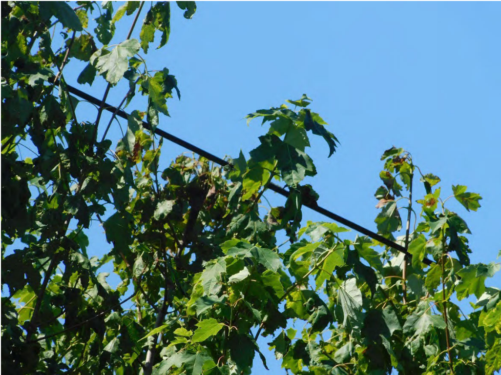
Probable violation B.83: Multiple trees show evidence of contacting the primary conductor behind 3756 NW Devoto Lane, Portland. (45.5512, -122.7714)
