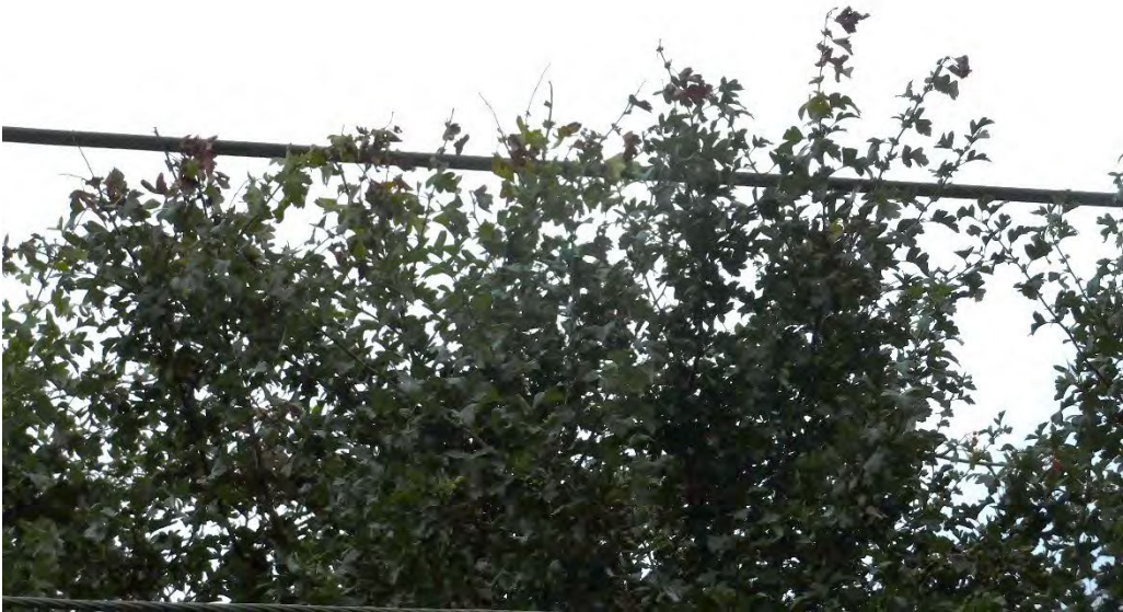
Probable violation B.198: Multiple trees show evidence of contacting the primary conductor at 10264 SE 37 th Avenue, Portland. (45.4491, -122.6247)
