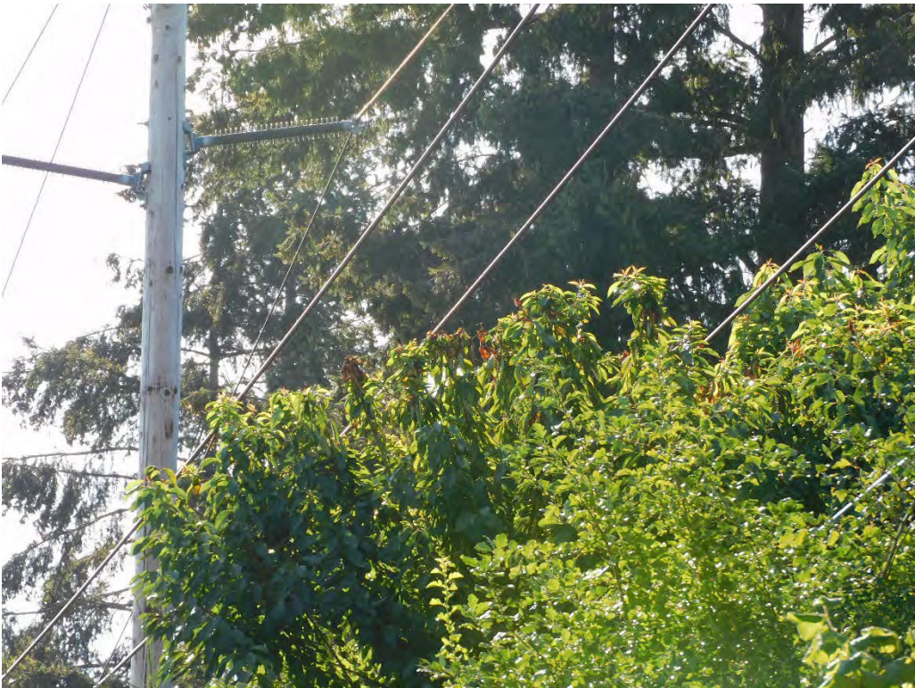
Probable violation B.43: Tree shows evidence of contacting primary conductors on SW Tualatin Valley Highway, Hillsboro. (45.5199, -123.0166)
