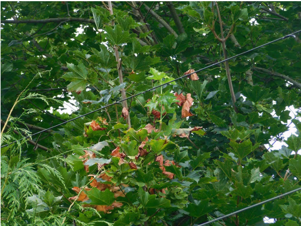
Probable violation B.190: Tree shows evidence of contacting primary conductors at 7643 SE Harmony Drive, Portland. (45.4411, -122.5844)
