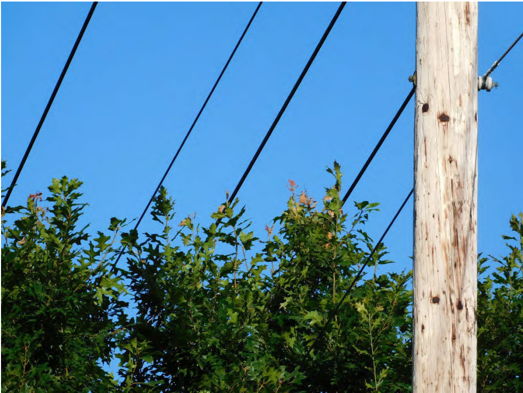
Probable violation B.42: Multiple trees show evidence of contacting the primary conductor at 3865 Baseline Street, Hillsboro. (45.5199, -123.0238)
