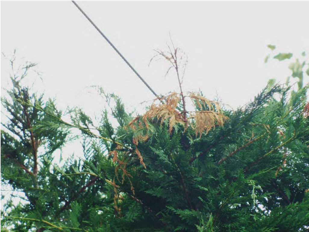
Probable violation B.202: Multiple trees show evidence of contacting the primary conductor at 8607 SE 29 th Avenue, Portland. (45.4605, -122.6330)
