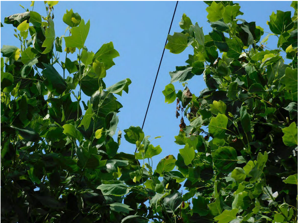
Probable violation B.333: Tree shows evidence of contacting primary conductors at 15275 South Maplelane Road, Oregon City. (45.3382, -122.553)
