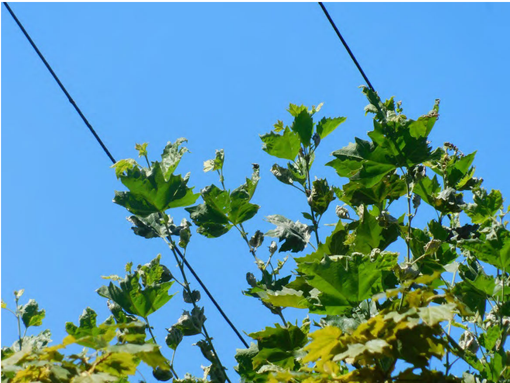
Probable violation B.69: Tree shows evidence of contacting primary conductors at 2376 NW Overton Street, Portland. (45.5318, -122.7002)
