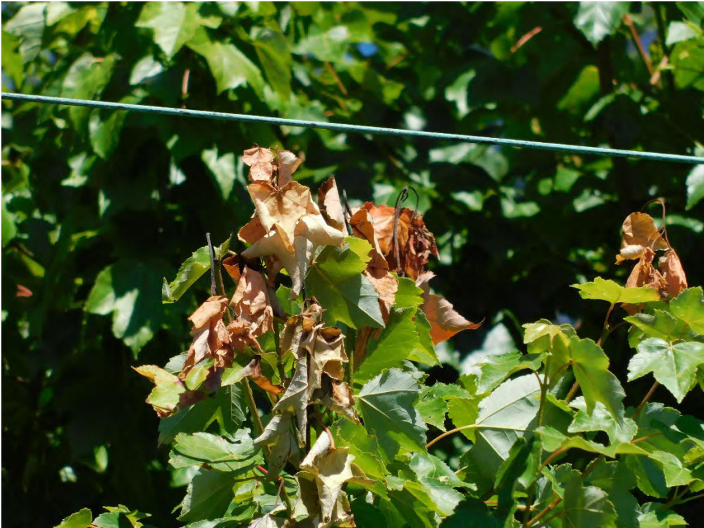
Probable violation B.138: Tree shows evidence of contacting primary conductors at 2911 SE Laurelwood Drive, Portland. (45.3987, -122.6326)
