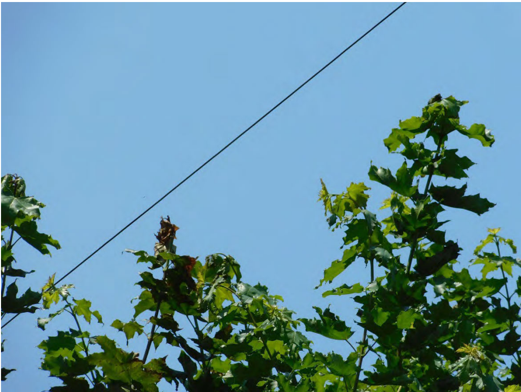
Probable violation B.275: Two trees show evidence of contacting primary conductors at 840 Barger Street, Silverton, Silverton. (44.9973, -122.7788)
