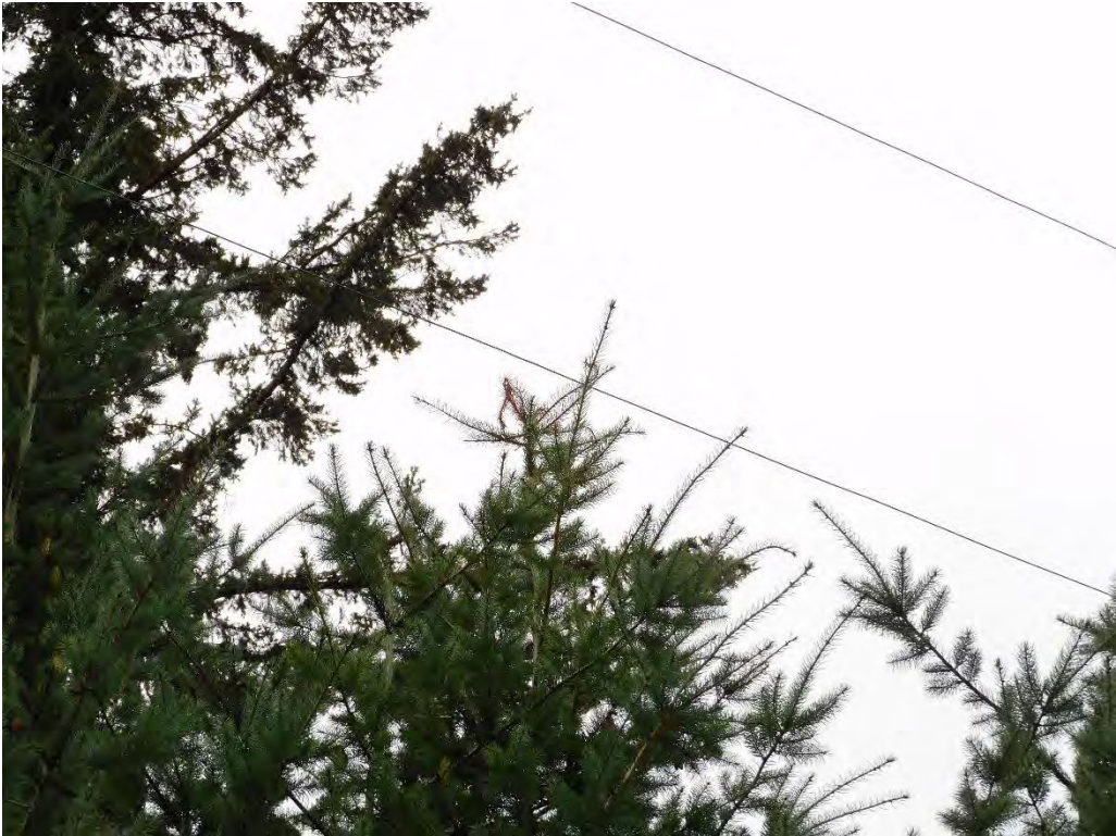
Probable violation B.370: Multiple trees show evidence of contacting primary conductors at 11528 SE Tyler Road, Happy Valley. (45.4504, -122.5438)
