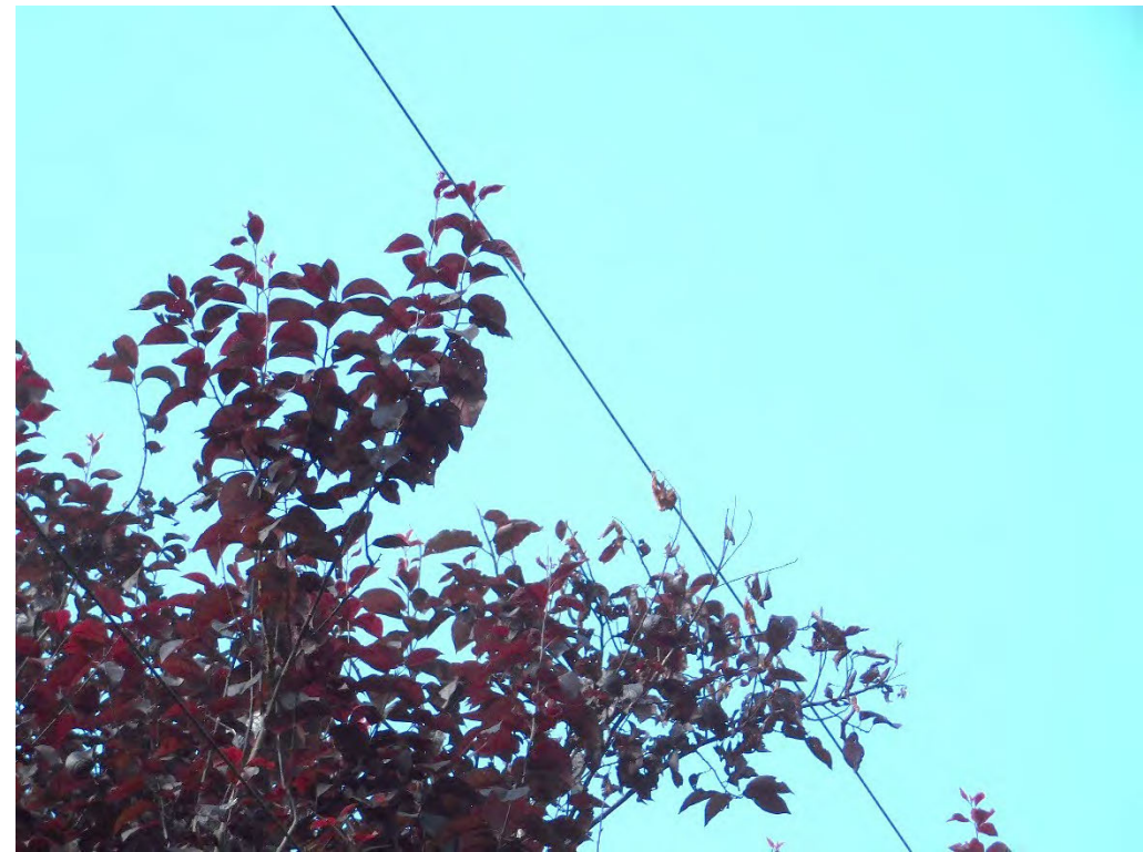
Probable violation B.284: Tree shows evidence of contacting primary conductors at 7215 Lakeside Drive NE, Salem. (45.0231, -122.9612)
