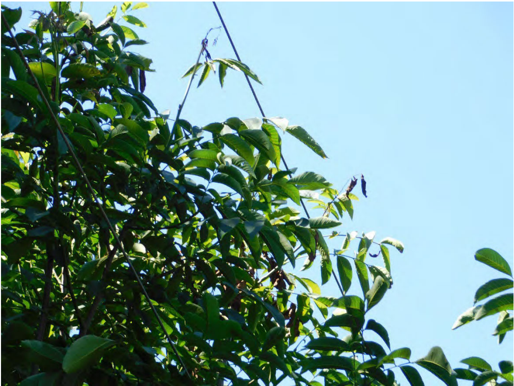
Probable violation B.316: Tree shows evidence of contacting primary conductors at 15143 South Macksburg Road, Molalla. (45.1660, -122.5473)
