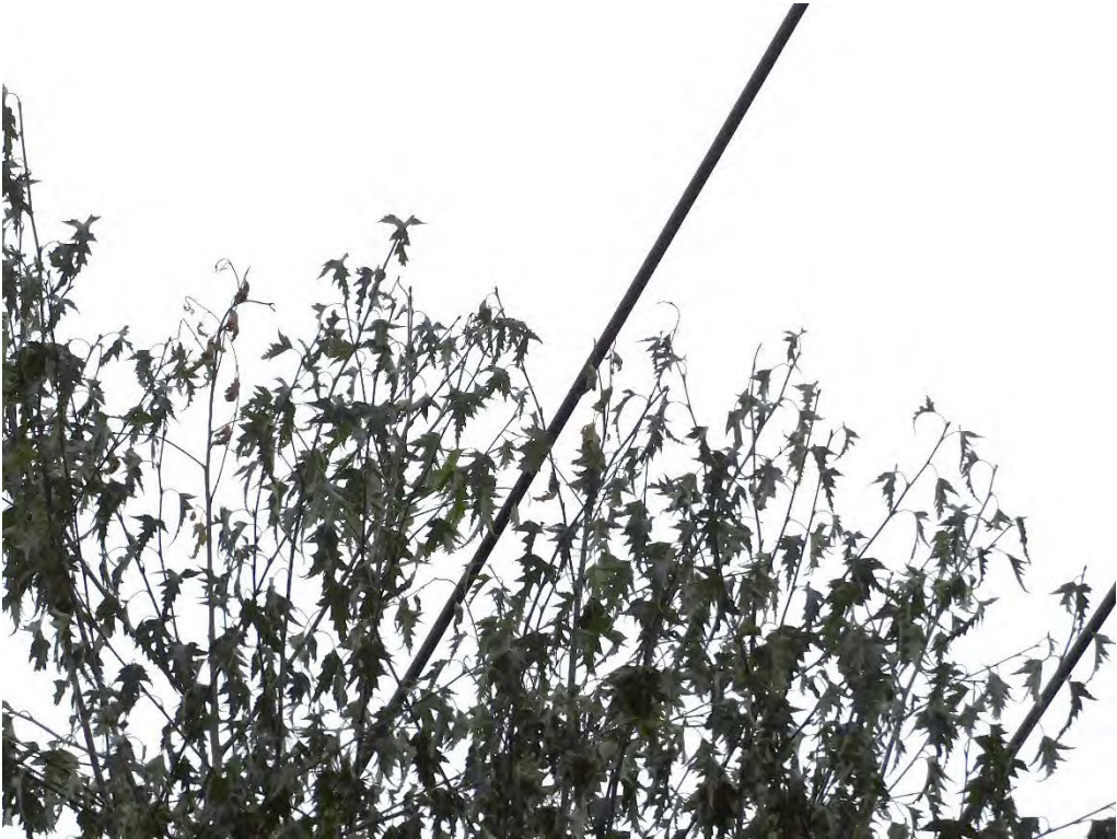
Probable violation B.369: Multiple trees show evidence of contacting primary conductors at 6625 SE 182nd Avenue, Gresham. (45.4745, -122.4757)
