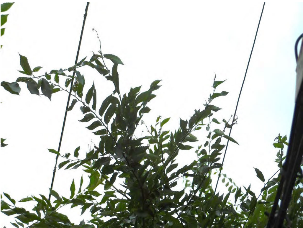
Probable violation B.154: Tree shows evidence of contacting primary conductors at 2710 SE Concord Road, Portland. (45.4063, -122.6349)
