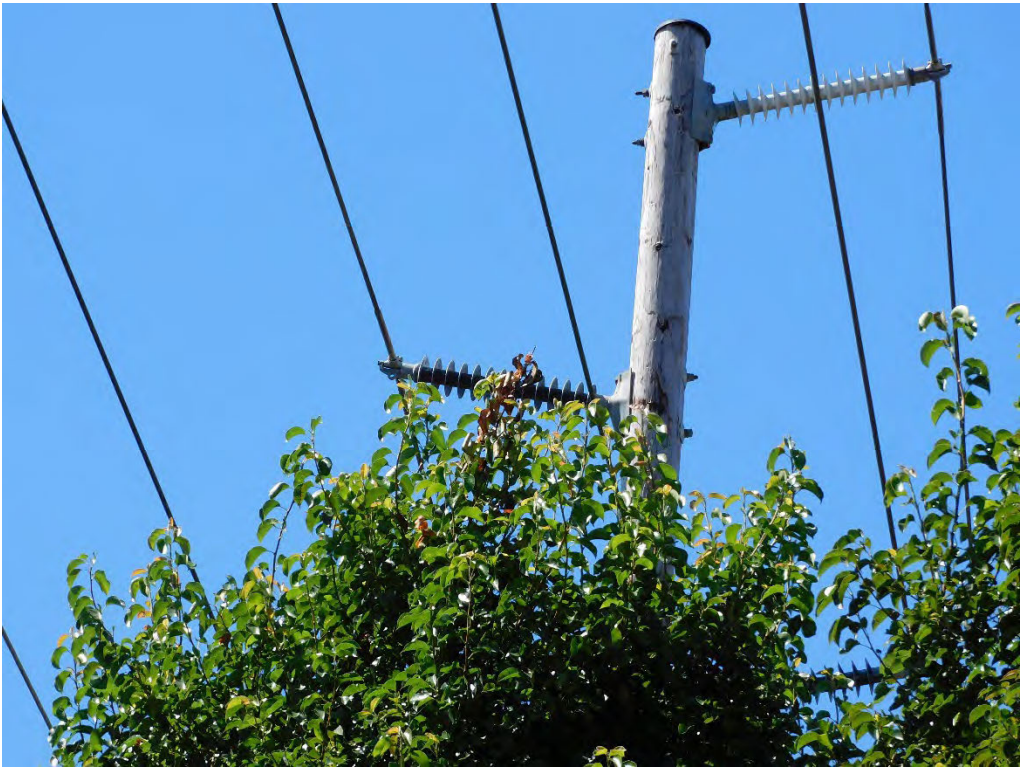
Probable violation B.353: Tree shows evidence of contacting primary conductors on SE Dodge Park Blvd., Gresham. (45.4705, -122.3475)
