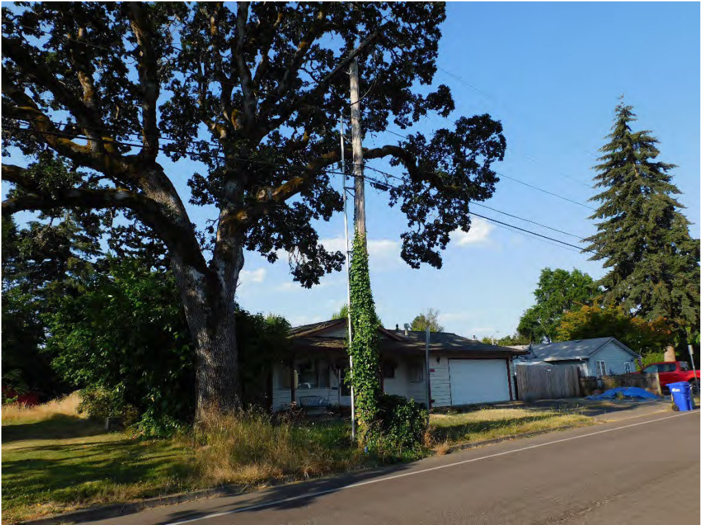
Probable violation C.1: Vines engulfing pole are creating a climbing hazard at 1537 South Dogwood Street, Cornelius. (45.5166, -123.0526)
