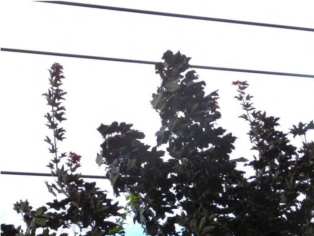
Probable violation B.193: Tree shows evidence of contacting primary conductors at 11415 SE Stanley Avenue, Portland. (45.4403, -122.6037)
