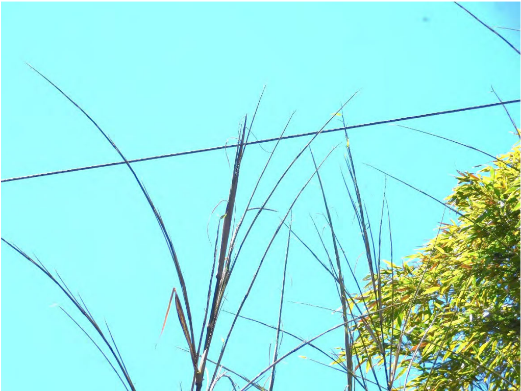
Probable violation B.145: Tree shows evidence of contacting primary conductors at 15695 SE Dana Avenue, Portland. (45.4093, -122.6489)
