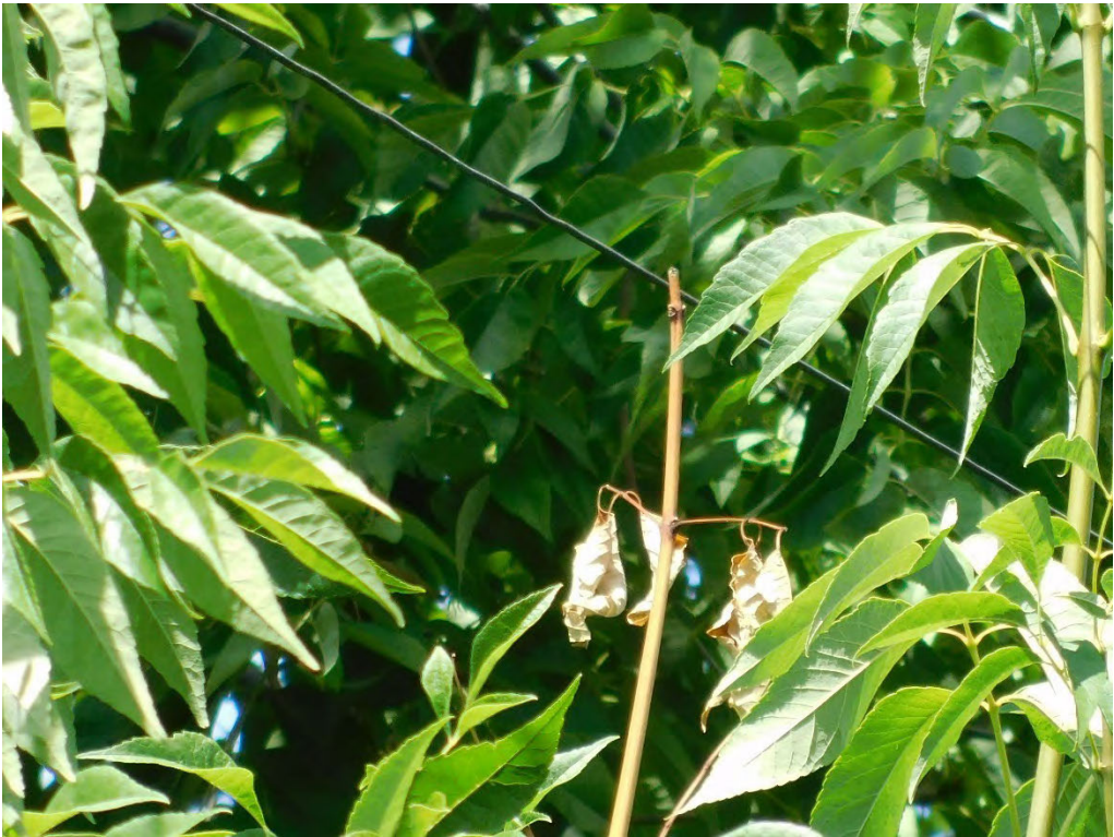
Probable violation B.13: Tree shows evidence of contacting primary conductors at 631 Winter Street NE, Salem. (44.9446, -123.0294)
