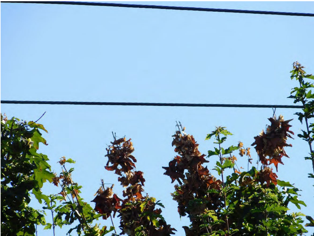
Probable violation B.10: Tree shows evidence of contacting primary conductors on Boone Road SE, Salem. (44.8823, -123.0458)
