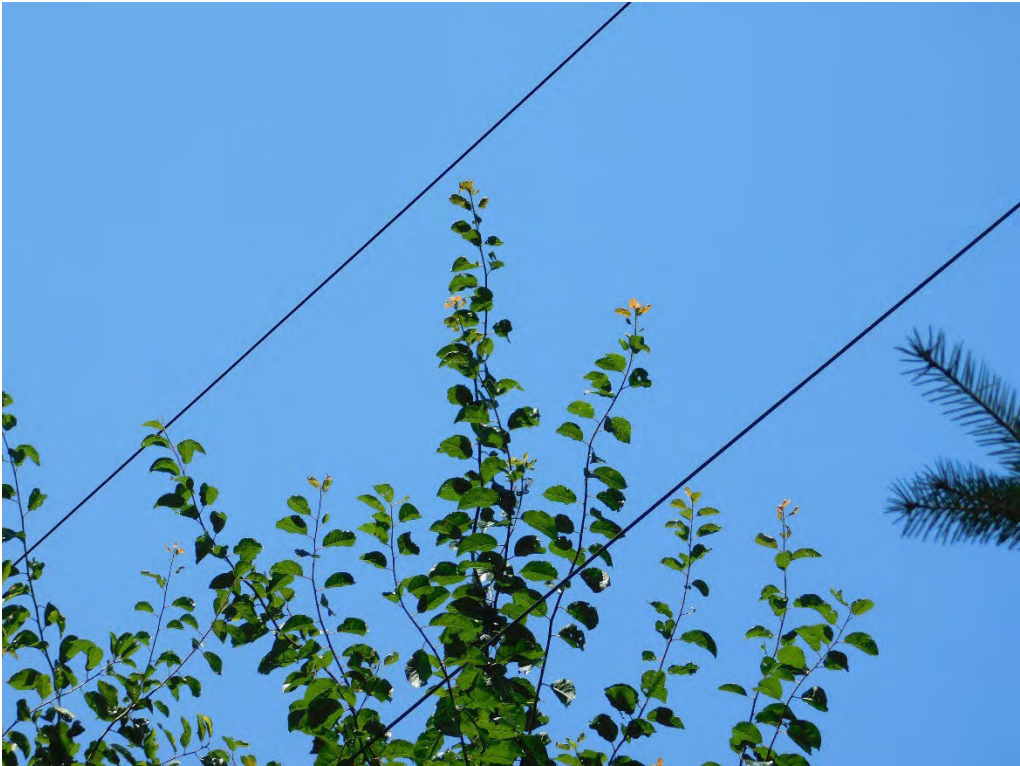
Probable violation B.278: Tree shows evidence of contacting primary conductors at 11151 South Wildcat Road, Molalla. (45.0783, -122.6367) HFRZ
