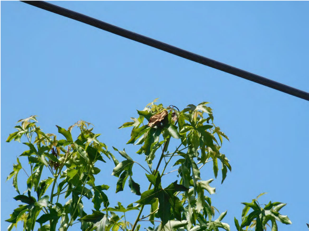
Probable violation B.168: Tree shows evidence of contacting primary conductors at 6050 SE Alderhill Loop, Portland. (45.4171, -122.6004)
