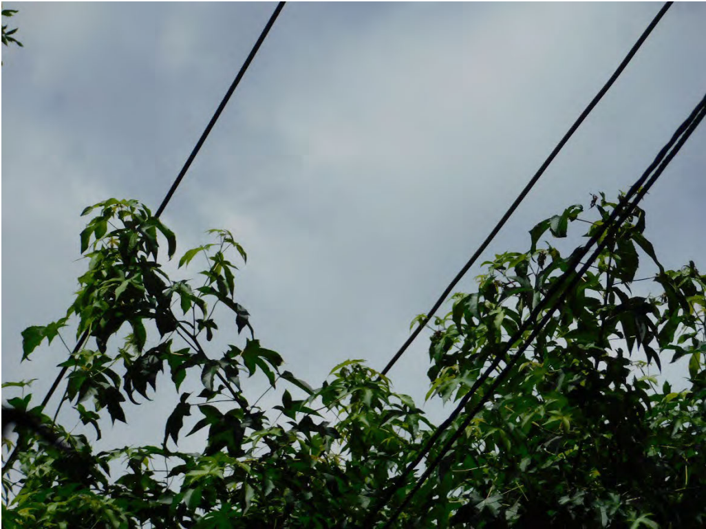
Probable violation B.126: Tree shows evidence of contacting primary conductors at the intersection of Woodside Circle and Deerbrush Avenue, Lake Oswego (45.3962, -122.7218)
