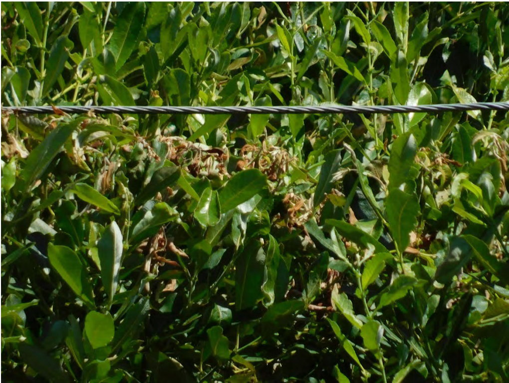
Probable violation B.84: Tree shows evidence of contacting primary conductors at the intersection of NW Wind Ridge Drive and NW Skyline Blvd., Portland. (45.5570, -122.7796)
