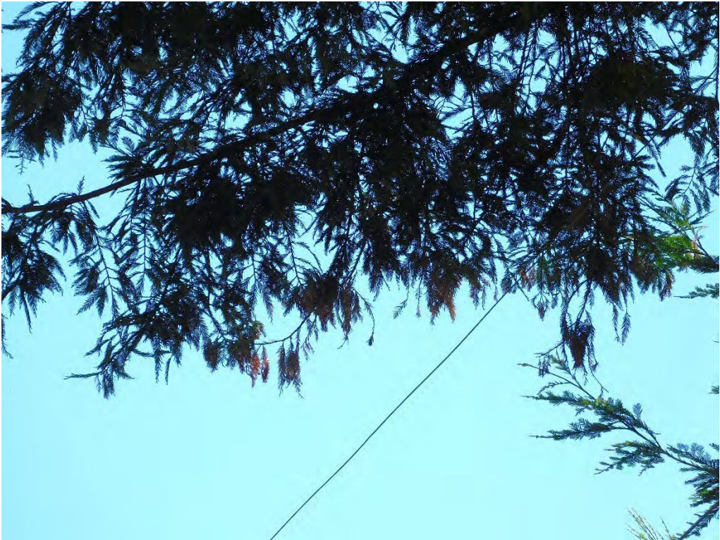
Probable violation B.351: Tree shows evidence of contacting primary conductors on SE Victory Road, Troutdale. (45.4938, -122.3364)
