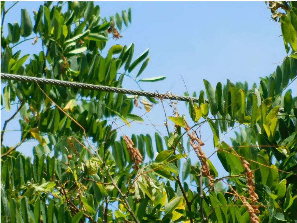
Probable violation B.108: Multiple trees show evidence of contacting the primary conductor at 4875 SW Schatz Road, Tualatin. (45.3574, -122.7265)
