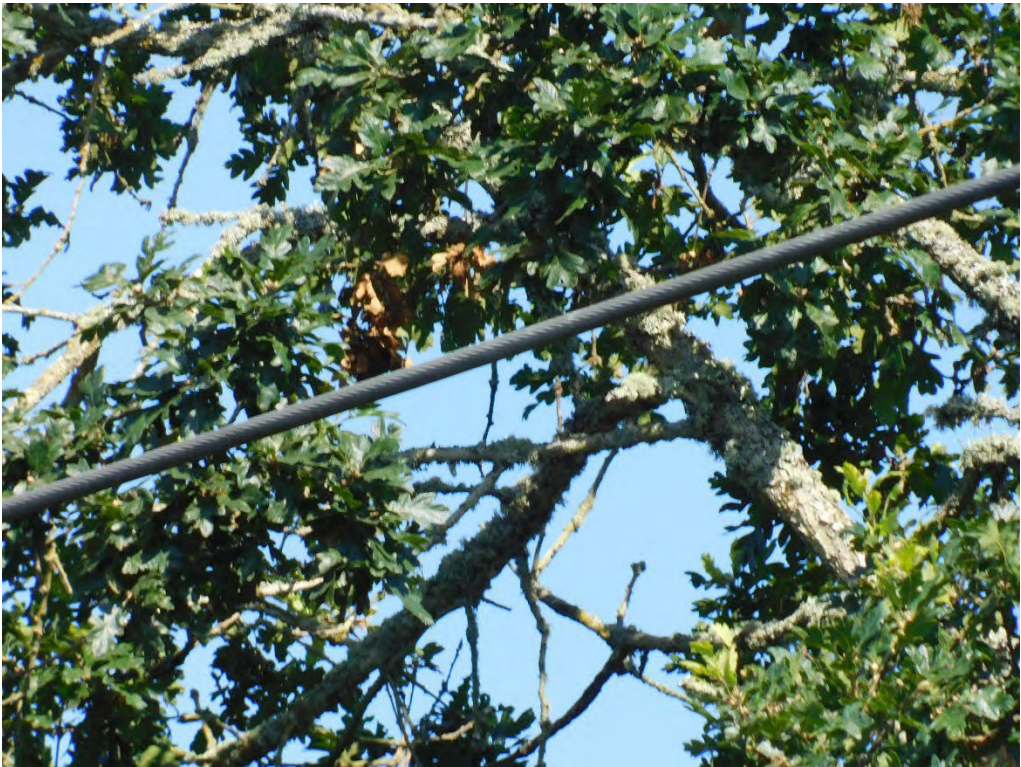
Probable violation B.250: Tree shows evidence of contacting primary conductors at 5335 Chicago Street SE, Turner. (44.8427, -122.9507)
