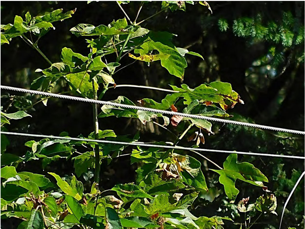
Probable violation B.3: Tree shows evidence of contacting primary conductors at 5045 River Road South, Salem. (44.8824, -123.1369)
