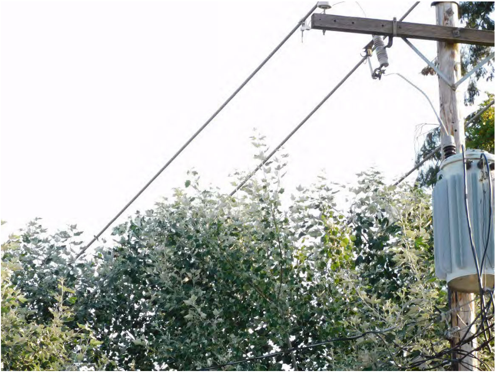
Probable violation A.3: Hazard: Readily climbable tree shows evidence of contacting the primary conductor at 540 SW Dennis Avenue, Hillsboro. (45.5167, -122.9958)
