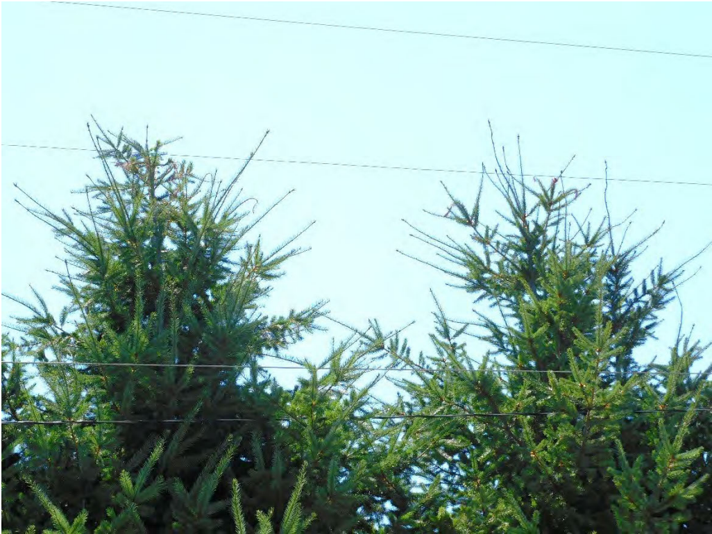
Probable violation B.352: Multiple trees show evidence of contacting primary conductors on SE Lusted Road, Gresham. (45.4759, -122.3323)
