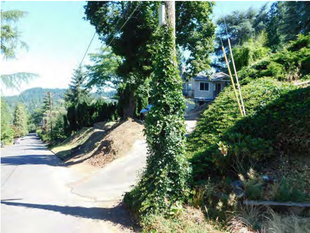
Probable violation C.21: Vines engulfing pole are creating a climbing hazard at 6510 SW 32 nd Avenue, Portland. (45.4775, -122.7095)
