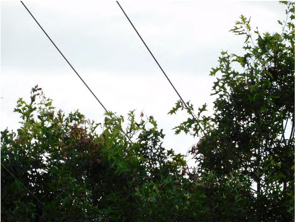
Probable violation A.17: Hazard: Readily climbable tree shows evidence of contacting the primary conductor on South Haines Road, Canby. (45.2723, -122.6610)
