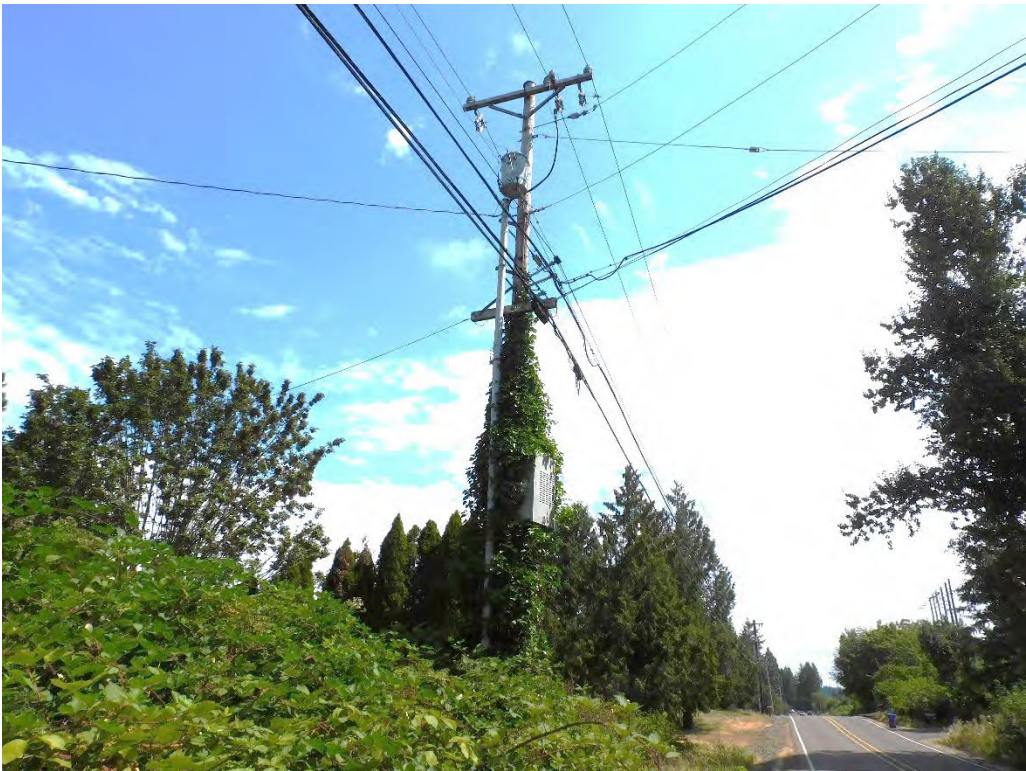
Probable violation C.16: Vines engulfing pole are creating a climbing hazard at 14831 South Maplelane Road, Oregon City. (45.3371, -122.5614)
