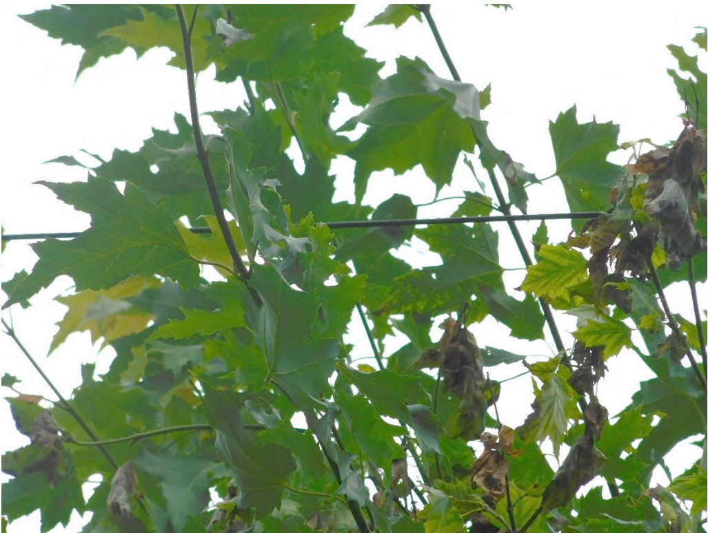
Probable violation B.95: Two trees show evidence of contacting the primary conductor at 5741 SW Pasadena Drive, Portland. (45.4457, -122.7359)
