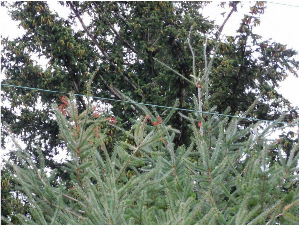
Probable violation B.371: Two trees show evidence of contacting primary conductors at 9615 SE Eastview Drive, Happy Valley. (45.4536, -122.5482)
