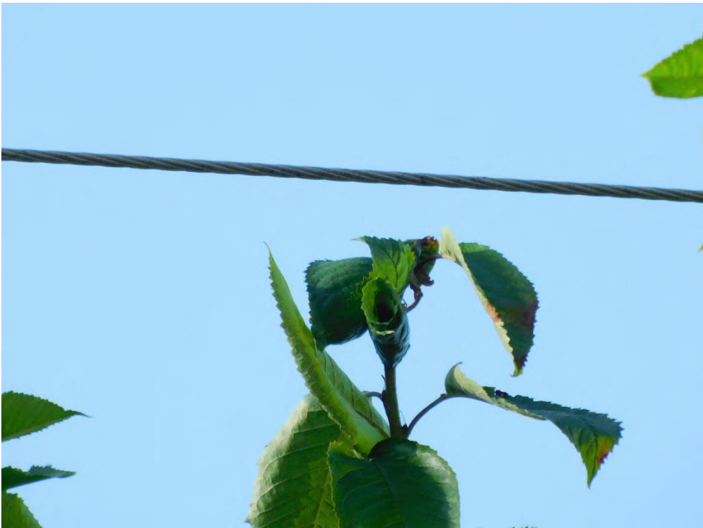
Probable violation B.2: Tree shows evidence of contacting primary conductors on Kuebler Blvd. South, Salem. (44.8832, -123.0803)
