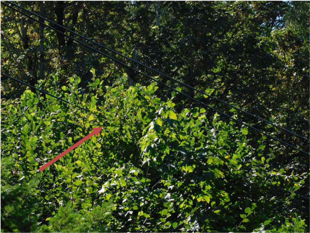
Probable violation B.347: Tree shows evidence of contacting primary conductors on SE Littlepage Road, Corbett. (45.5083, -122.2857)
