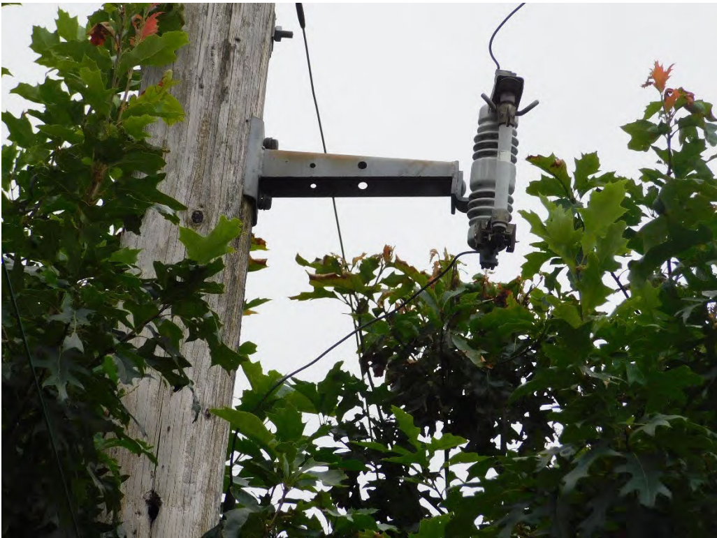
Probable violation B.184: Tree shows evidence of contacting primary conductors at 10920 SE 72 nd Avenue, Portland. (45.4438, -122.5893)
