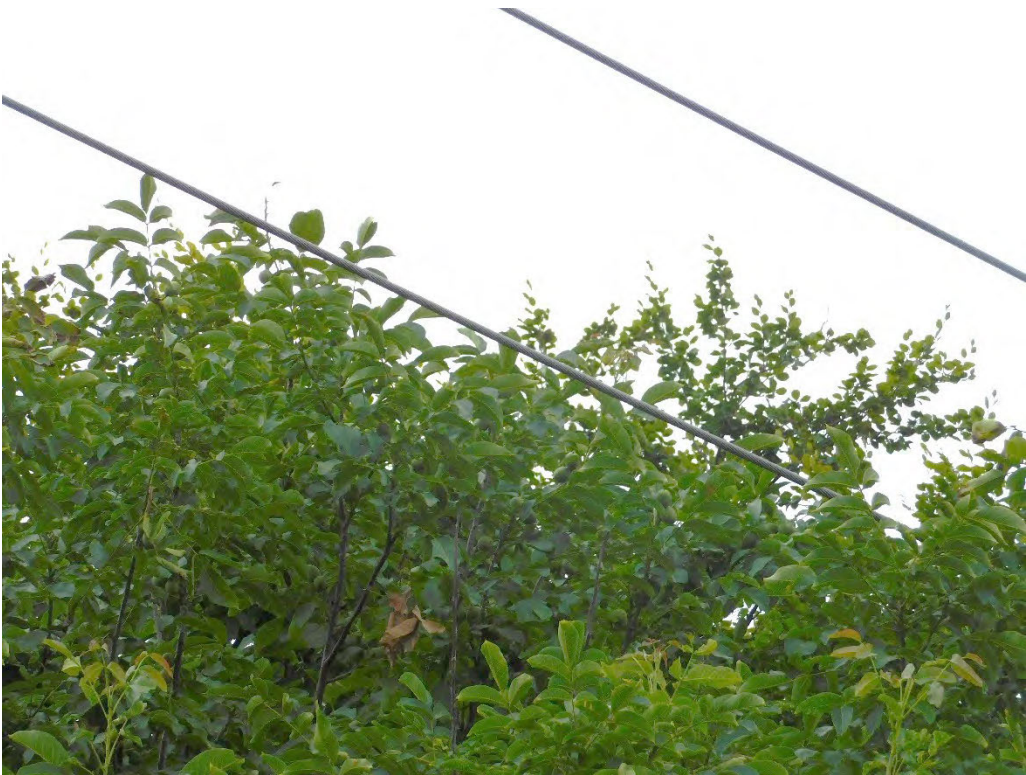
Probable violation B.178: Tree shows evidence of contacting primary conductors at 7816 SE Stephanie Court, Portland. (45.4379, -122.5838)
