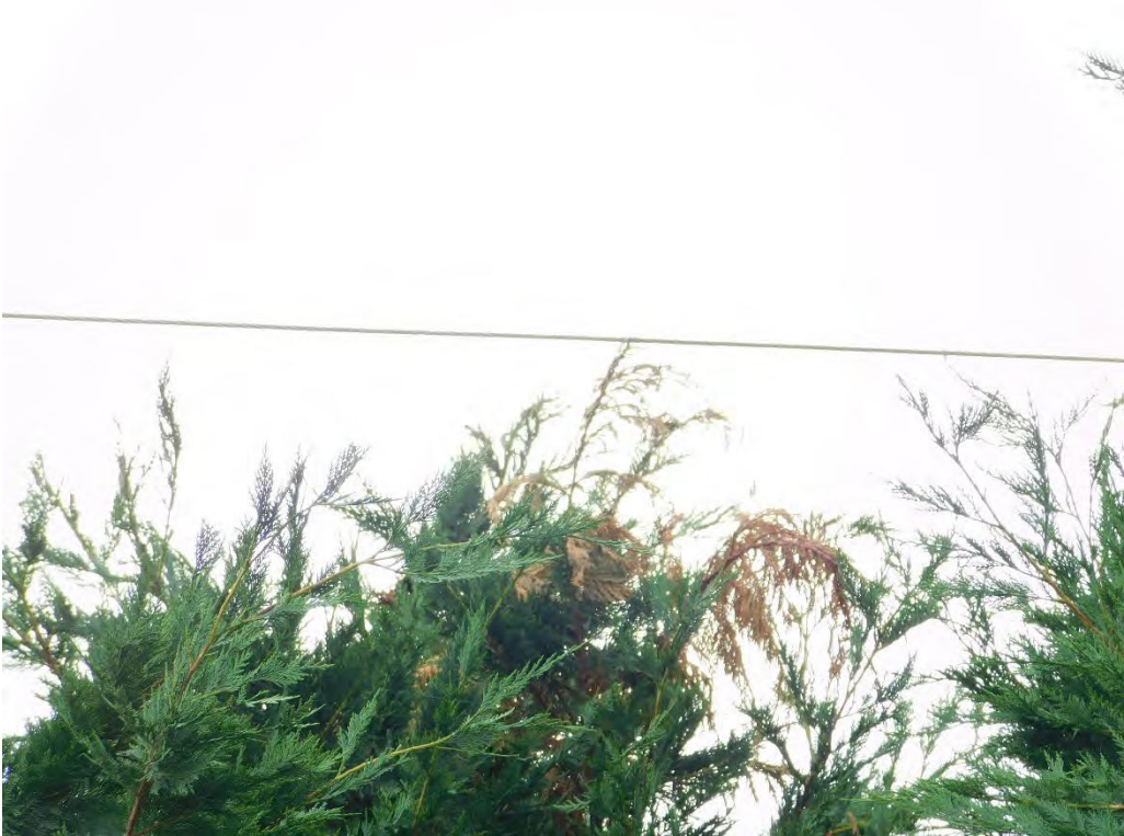
Probable violation B.242: Tree shows evidence of contacting primary conductors on Dollar Street, West Linn. (45.3451, -122.6603)
