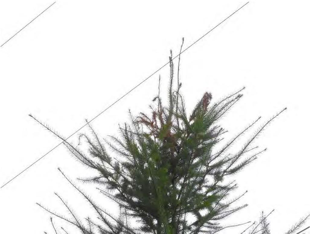
Probable violation B.37: Tree shows evidence of contacting primary conductors on NW Hahn Road, Banks. (45.6282, -123.0729)
