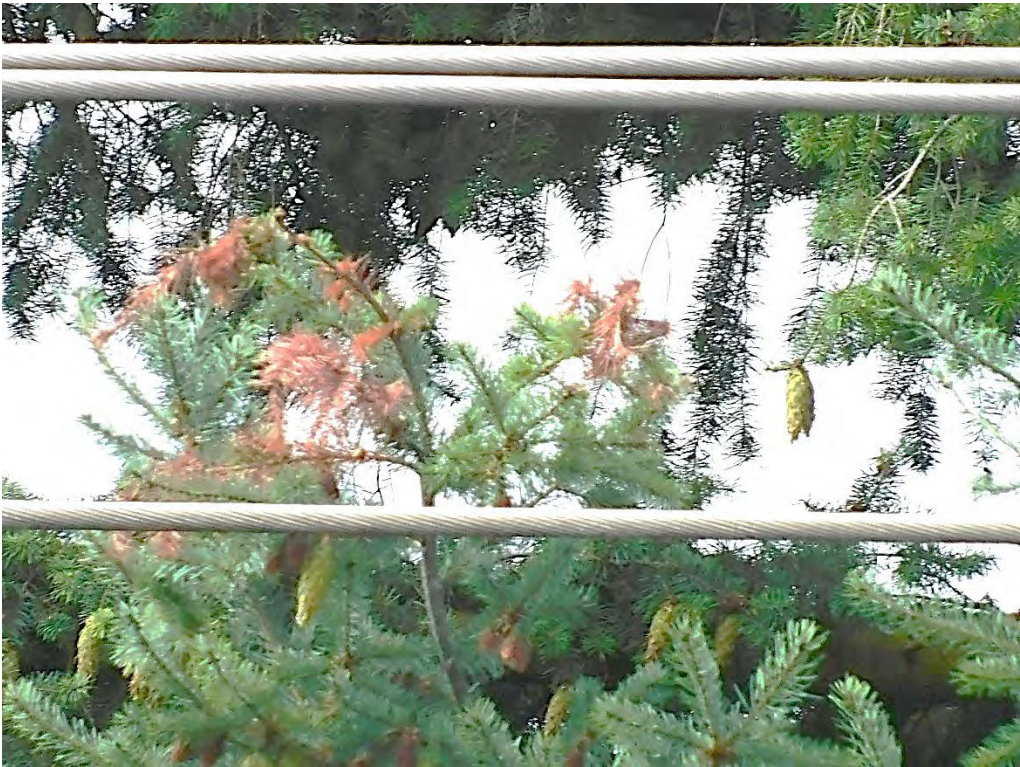
Probable violation B.147: Tree shows evidence of contacting primary conductors at 16417 SE McLoughlin Blvd., Portland. (45.4039, -122.6229)
