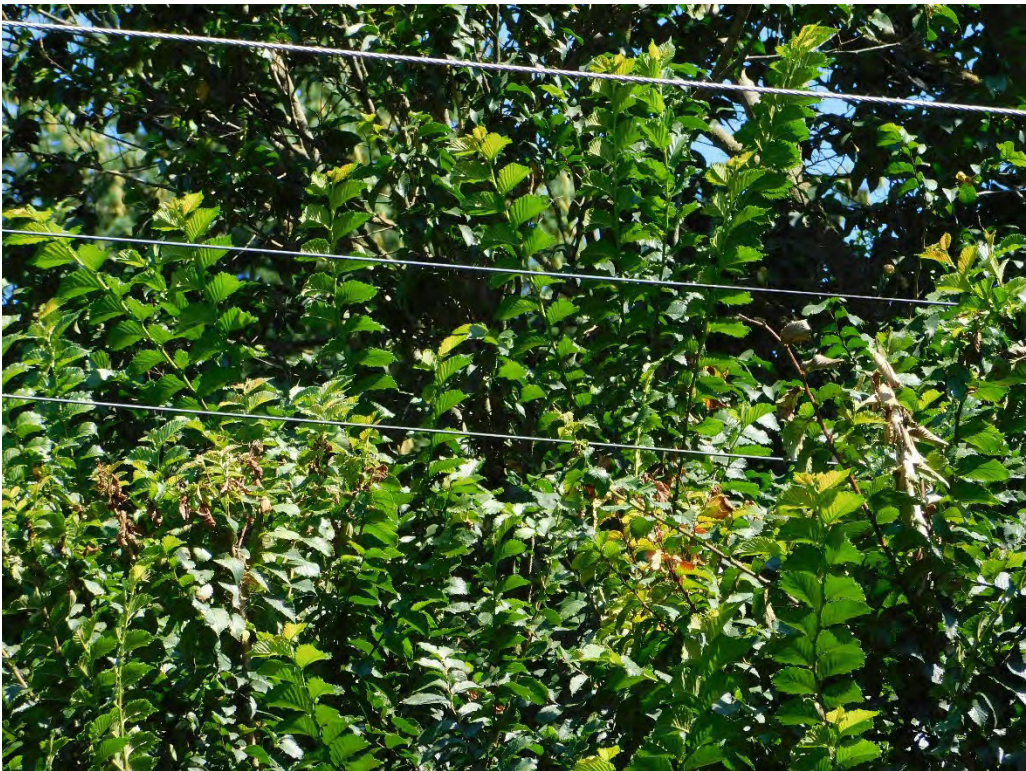
Probable violation B.6: Two trees show evidence of contacting the primary conductor at 4335 River Road South, Salem. (44.8931, -123.1304)
