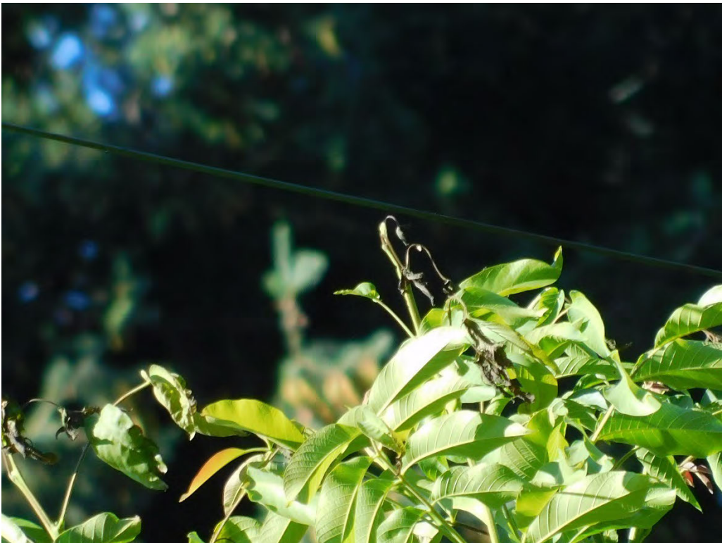
Probable violation B.111: Tree shows evidence of contacting primary conductors at 4342 SW Kanan Drive, Portland. (45.4821, -122.7220)
