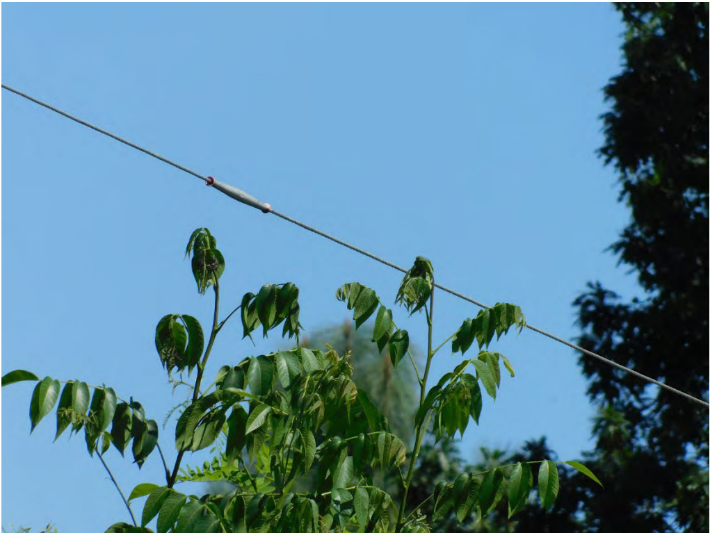
Probable violation B.306: Tree shows evidence of contacting primary conductors at 1050 South Pacific Highway, Woodburn. (45.1235, -122.8557)
