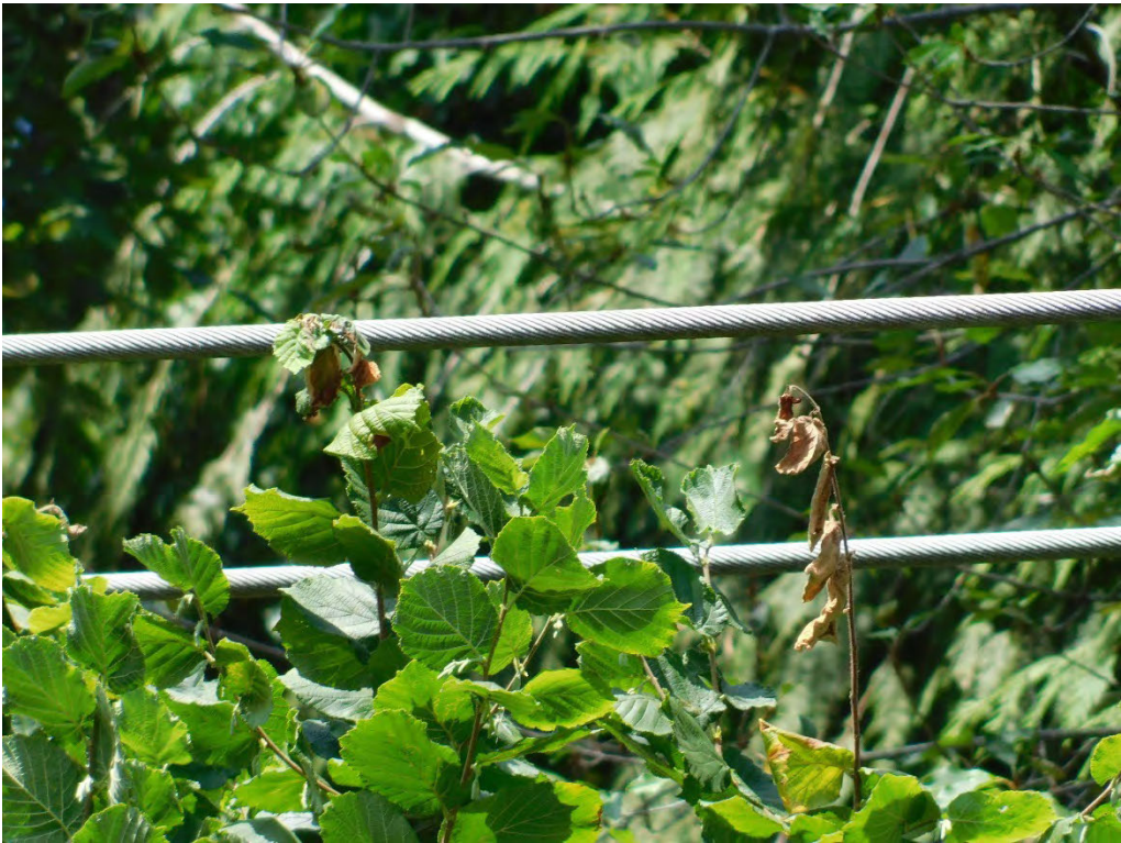
Probable violation B.235: Tree shows evidence of contacting primary conductors at 797 SW Borland Road, West Linn. (45.3556, -122.6847)
