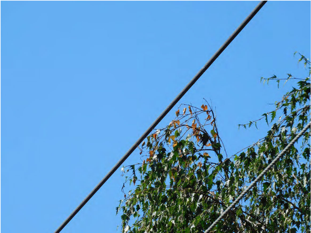
Probable violation B.48: Tree shows evidence of contacting primary conductors at 1299 NE 17th Avenue, Hillsboro. (45.5345, -122.9646)
