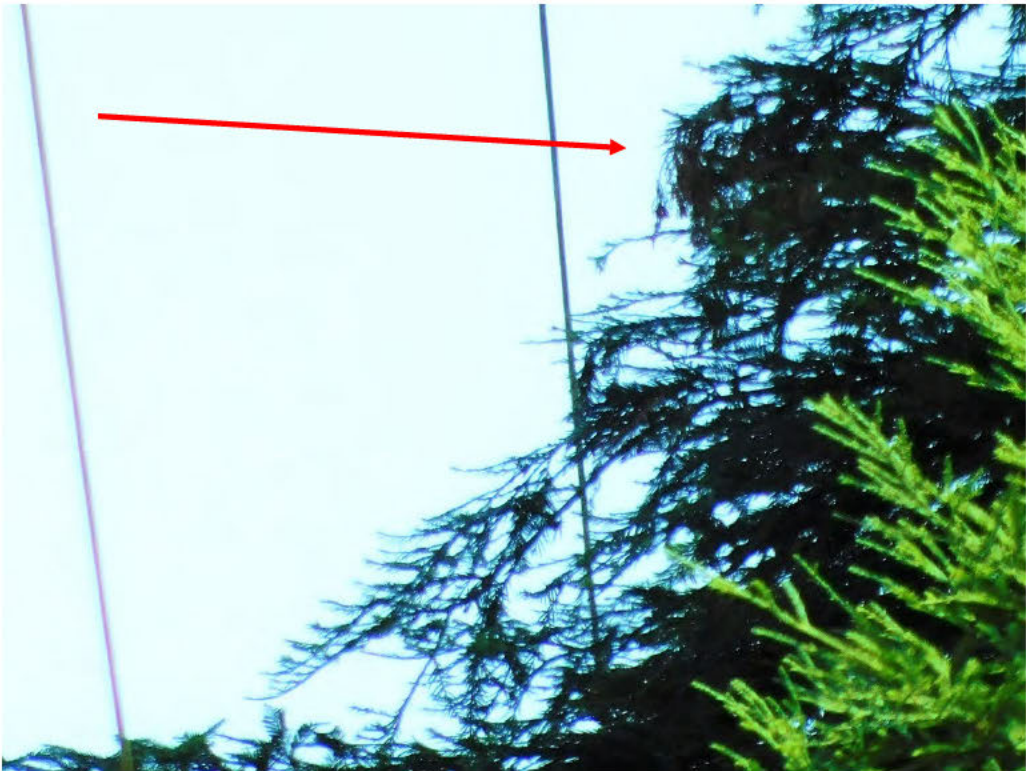
Probable violation B.271: Tree shows evidence of contacting primary conductors at 7373 Conifer Road NE, Salem. 44.9458, -122.9103)
