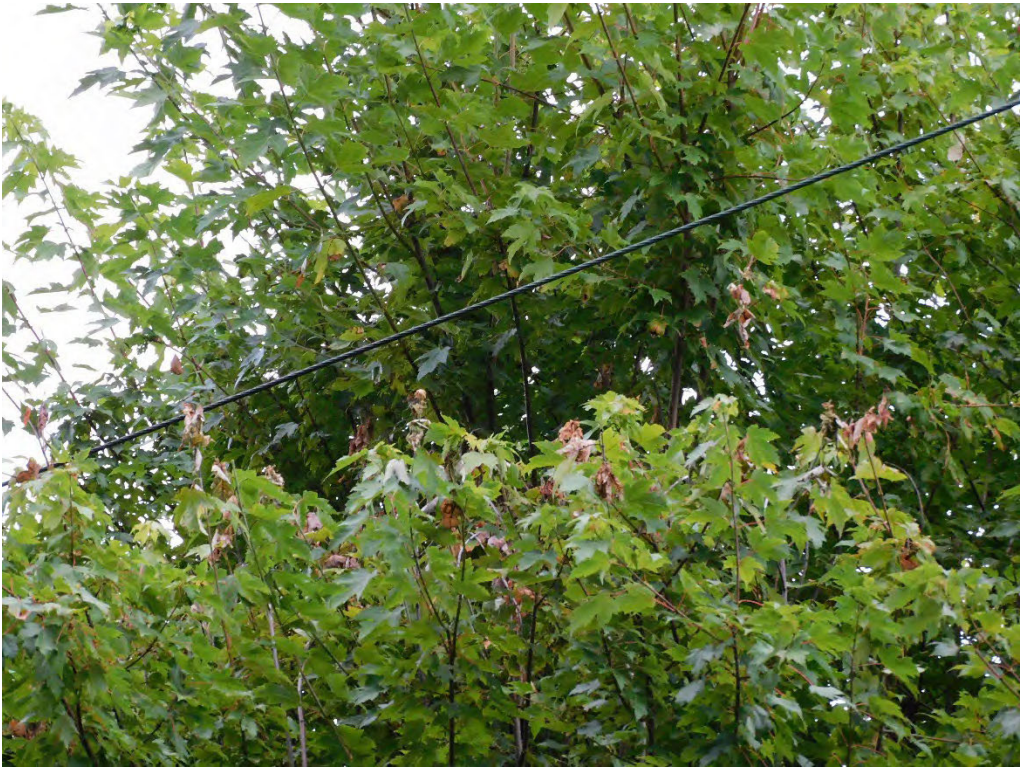
Probable violation B.361: Multiple trees show evidence of contacting primary conductors at 33685 SE Compton Road, Boring. (45.4327, -122.3272)
