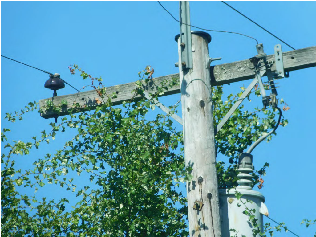
Probable violation C.4: Vines engulfing pole and approaching primary conductor are creating a hazard at 17731 SE River Road, Portland. (45.3945, -122.6236)
