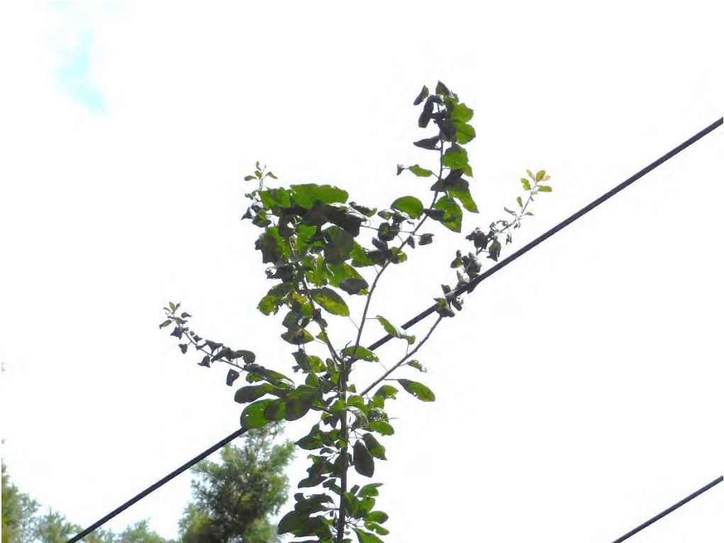
Probable violation B.121: Tree shows evidence of contacting primary conductors at 3188 Glenmorrie Drive, Lake Oswego. (45.4066, -122.6553)
