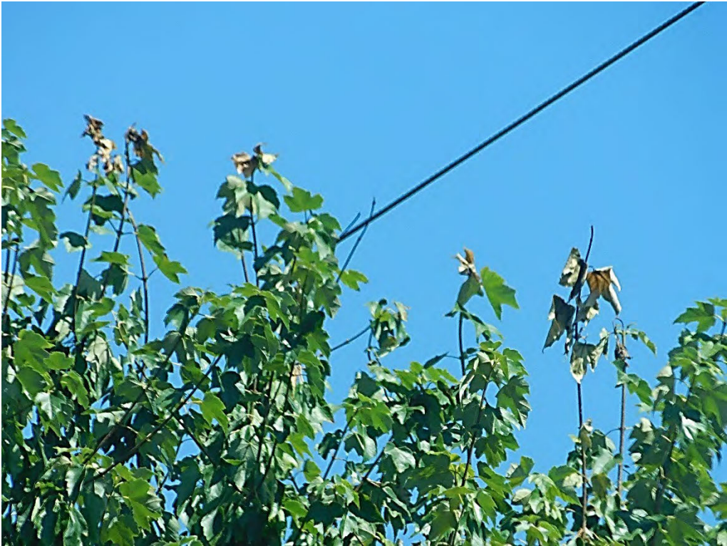
Probable violation B.219: Tree shows evidence of contacting primary conductors at 6232 SE 47 th Avenue, Portland. (45.4771, -122.6143)
