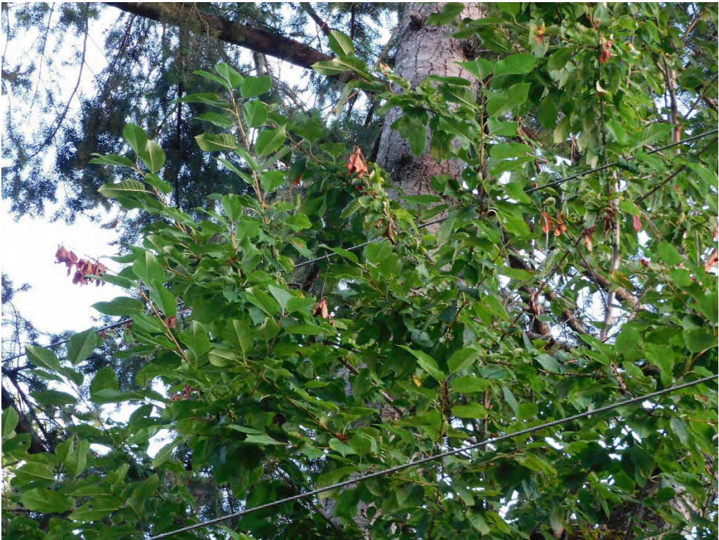
Probable violation B.337: Tree shows evidence of contacting primary conductors on South Lower Highland Road, Beaver Creek. (45.2621, -122.5014)
