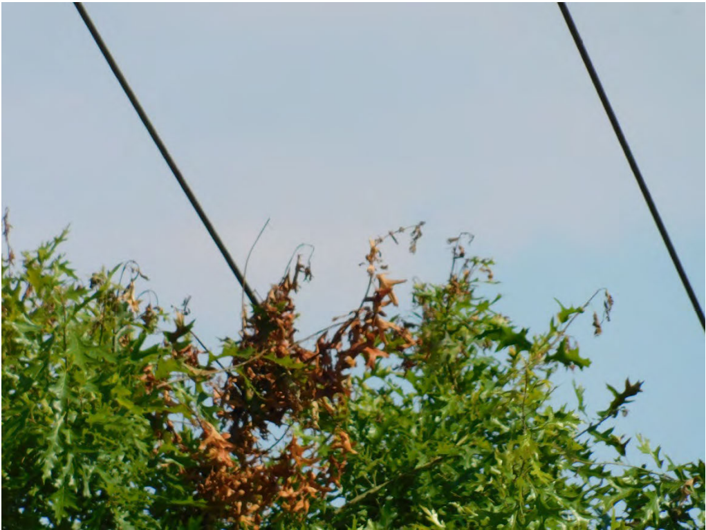
Probable violation B.264: Tree shows evidence of contacting primary conductors at the intersection of 45th Avenue NE and Herrin Road NE, Salem. (44.9771, -122.9731)
