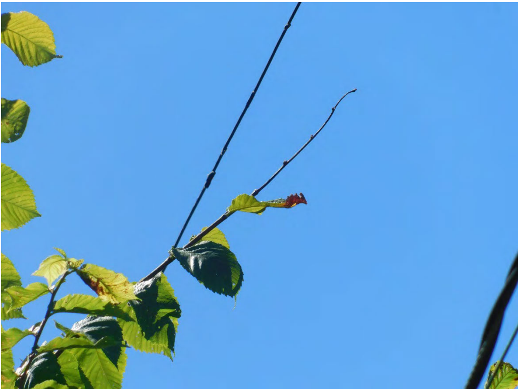
Probable violation B.63: Tree shows evidence of contacting primary conductors at 2486 NW Kearny Street, Portland. (45.5290, -122.7025)
