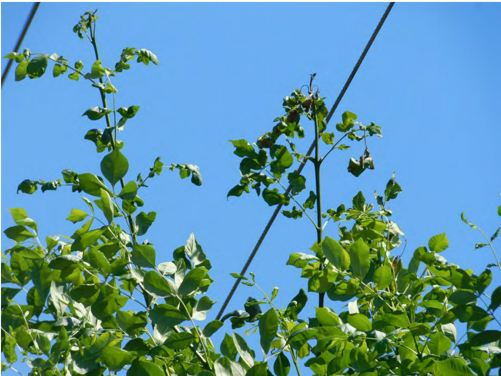
Probable violation B.321: Tree shows evidence of contacting primary conductors on Woodburn/Estacada Highway, Colton. (45.1700, -122.4598)
