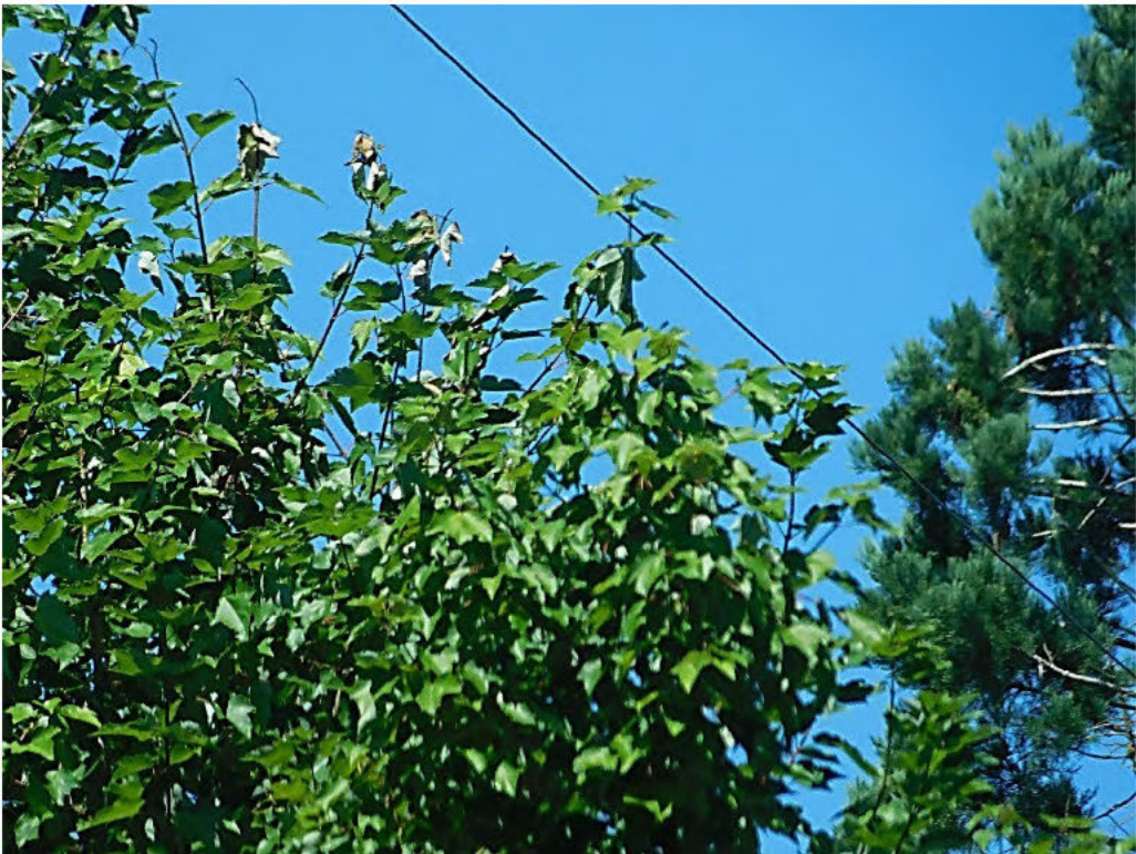
Probable violation B.142: Tree shows evidence of contacting primary conductors at 2420 SE Mulberry Drive, Portland. (45.4008, -122.6380)
