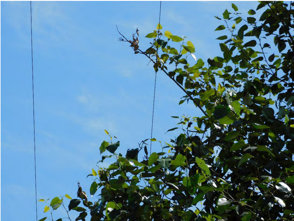
Probable violation B.357: Multiple trees show evidence of contacting primary conductors at 30830 SE Bluff, Gresham. (45.4652, -122.3451)
