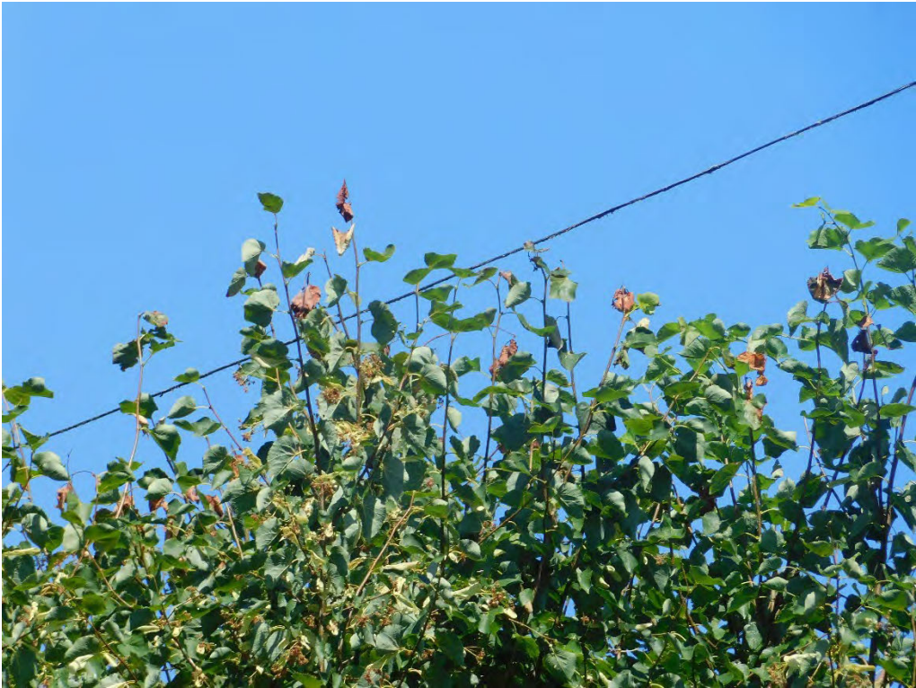
Probable violation B.211: Multiple trees show evidence of contacting the primary conductor across from 8230 SE Liebe Steet, Portland. (45.4870, -122.5782)
