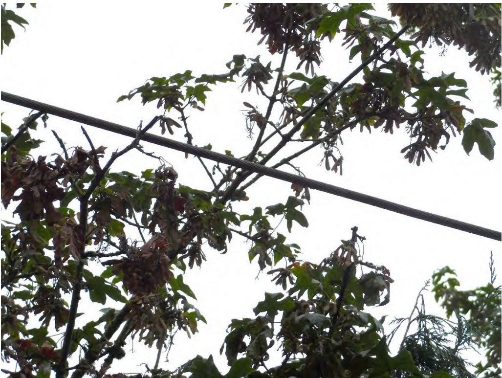
Probable violation B.116: Tree shows evidence of contacting primary conductors at 2249 SW Borland Road, Tualatin. (45.3721, -122.6997)
