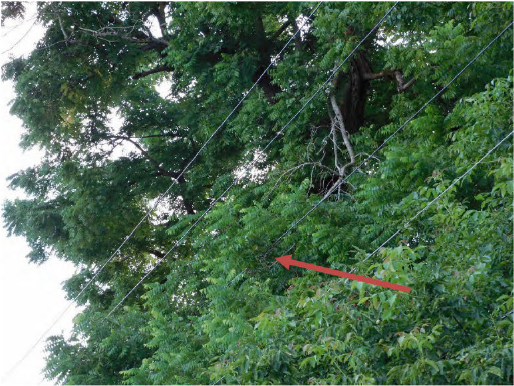
Probable violation B.329: Multiple trees show evidence of contacting primary conductors at 23300 South Blount Road, Canby. (45.2693, -122.6557)
