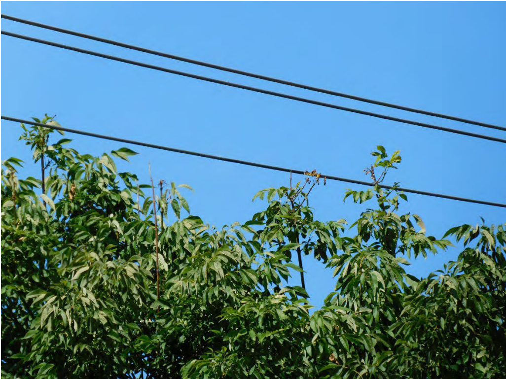
Probable violation A.18: Hazard: Readily climbable tree shows evidence of contacting the primary conductor across from 7142 SE 302nd Avenue, Gresham. (45.4712, -122.3525)
