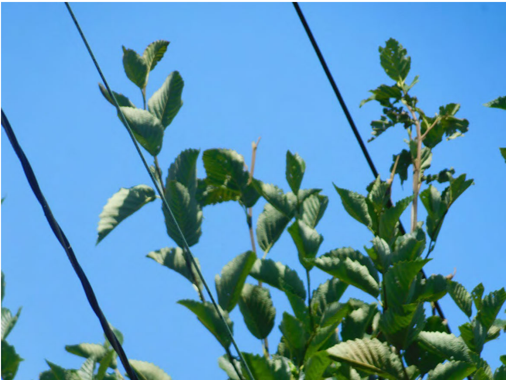
Probable violation B.81: Two trees show evidence of contacting the primary conductor at 8221 NW Cresap Lane, Portland. (45.5450, -122.7612) HFRZ
