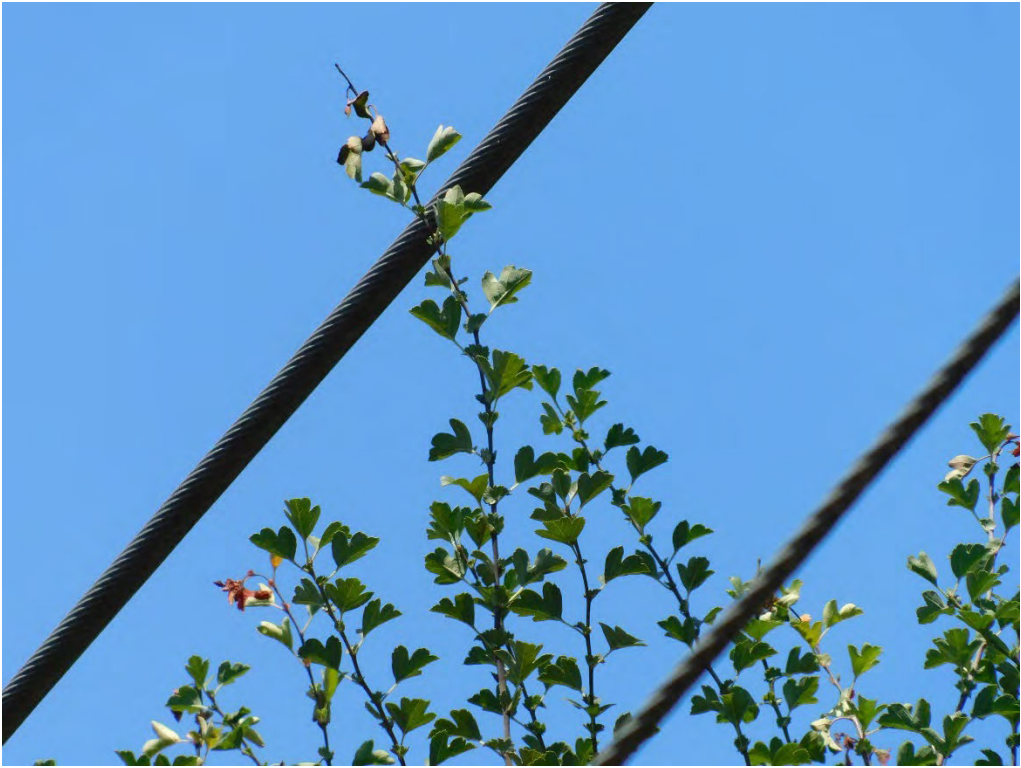
Probable violation B.173: Tree shows evidence of contacting primary conductors at 14928 SE Oatfield Road, Portland. (45.4146, -122.6248)
