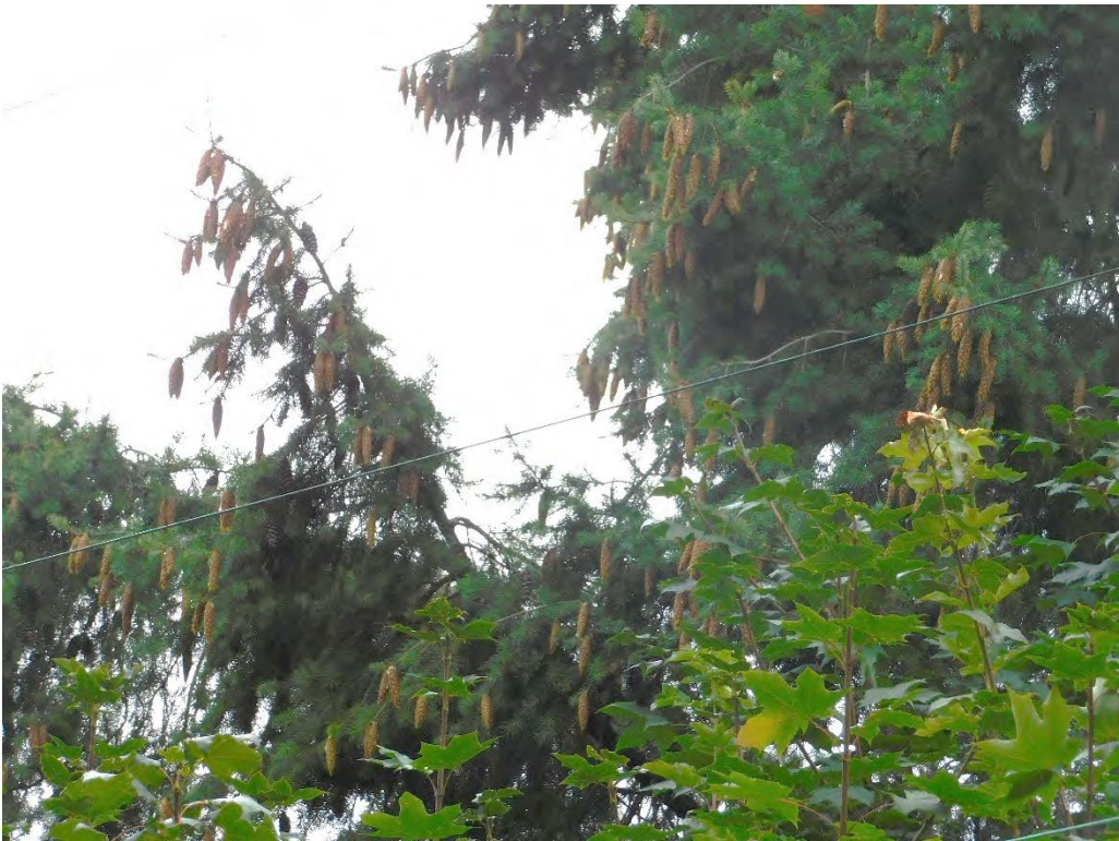
Probable violation B.176: Tree shows evidence of contacting primary conductors at 7506 SE Sunnyside Drive, Portland. (45.4333, -122.5865)
