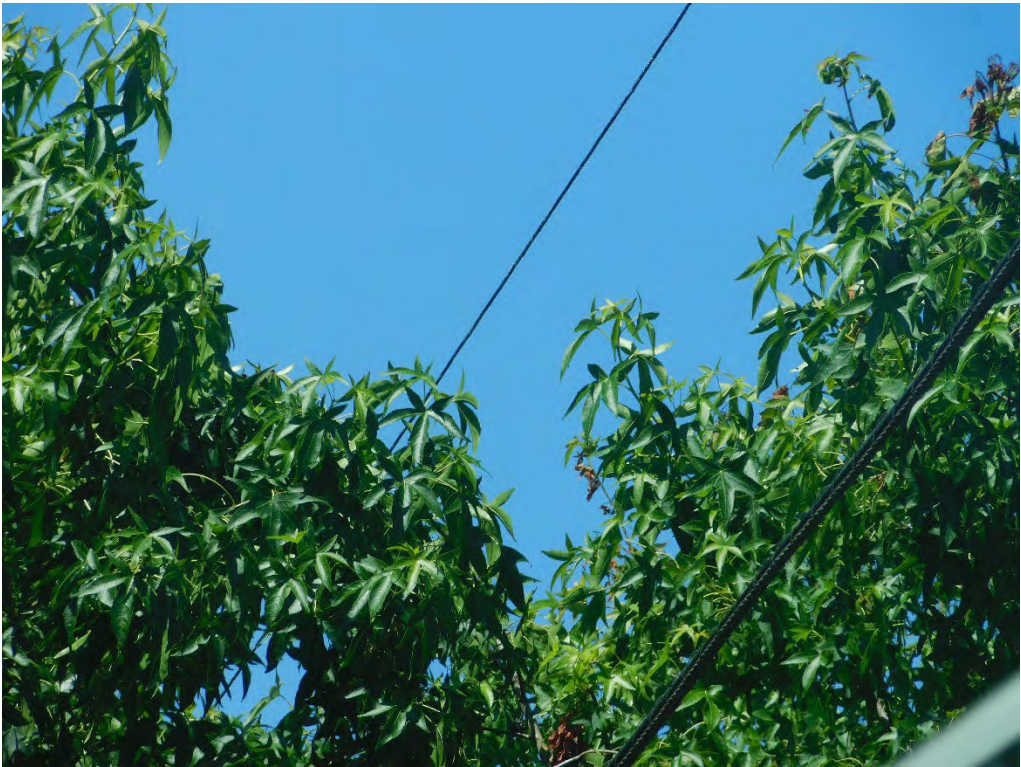
Probable violation B.217: Tree shows evidence of contacting primary conductors at 5519 SE Insley Street, Portland. (45.4839, -122.6061)
