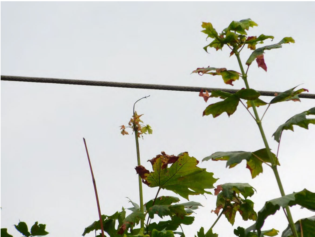
Probable violation B.109: Multiple trees show evidence of contacting the primary conductor at 22720 SW Stafford Road, Tualatin. (45.3555, -122.7268)
