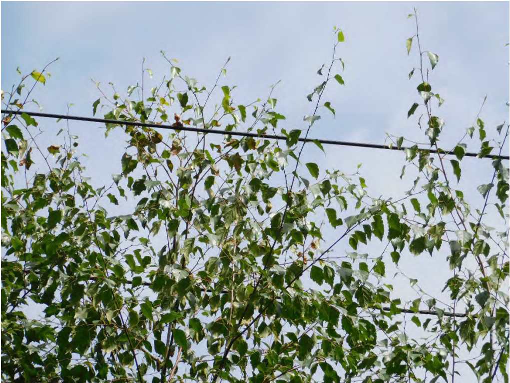
Probable violation B.123: Multiple trees show evidence of contacting the primary conductor at 2445 Glenmorrie Drive, Lake Oswego. (45.4031, -122.6571)
