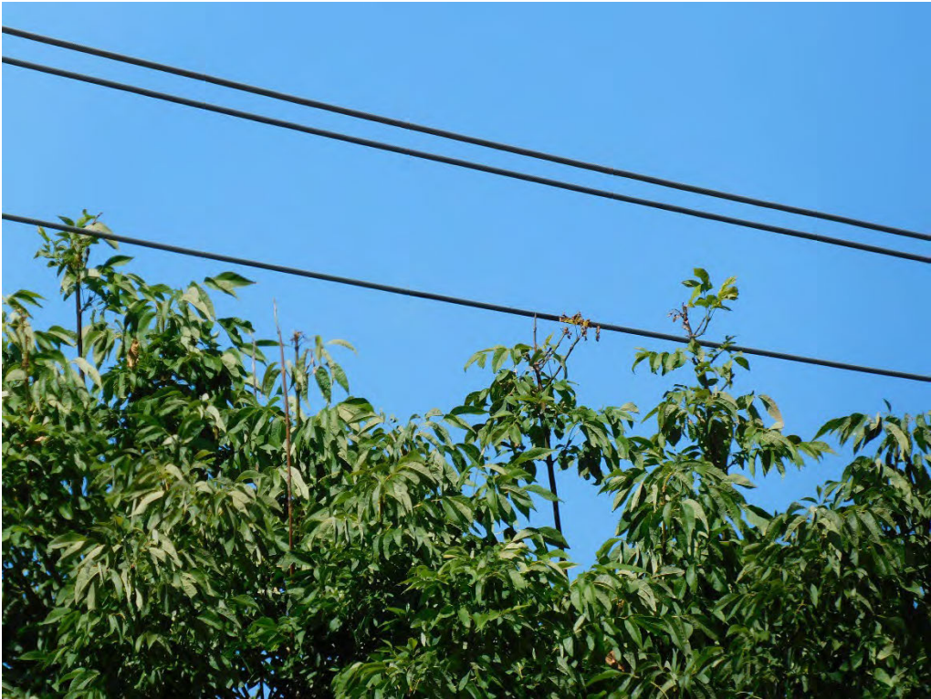
Probable violation A.7: Hazard: Readily climbable tree shows evidence of contacting the primary conductor across from 7142 SE 302 nd Avenue, Gresham. (45.4712, -122.3525)
