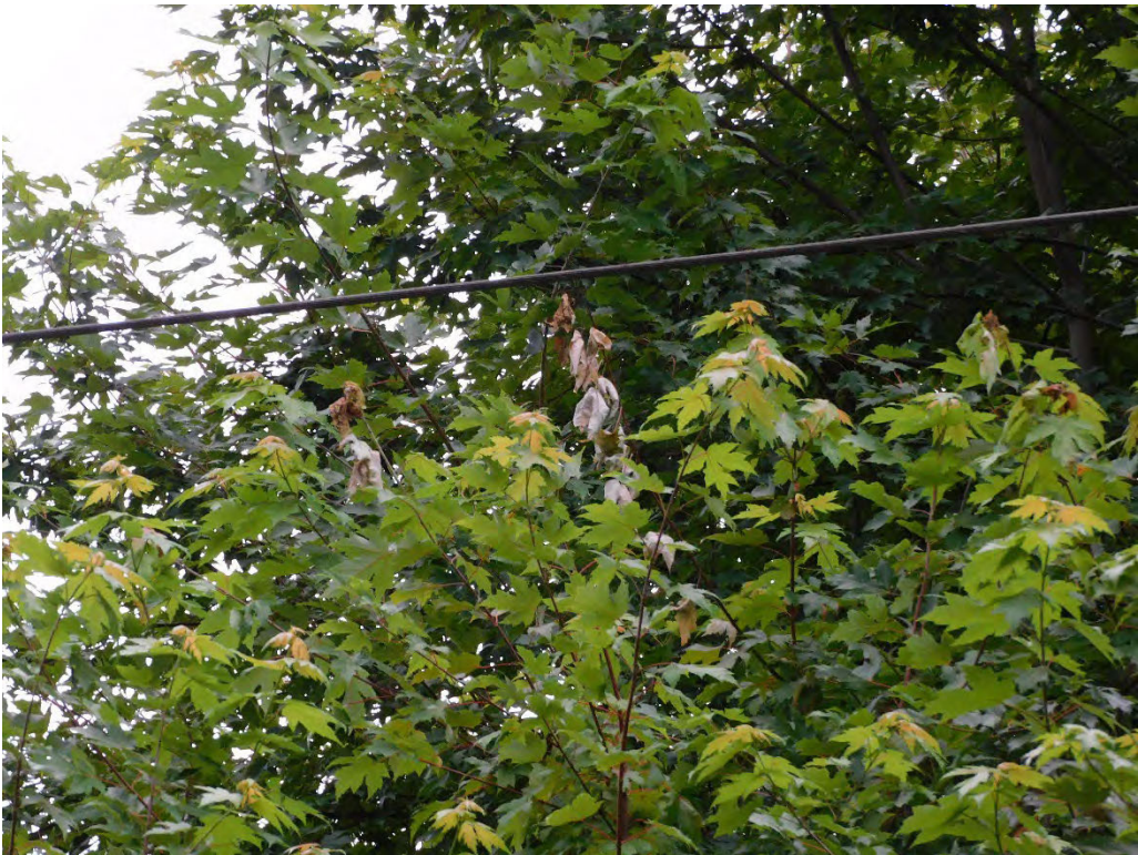
Probable violation B.366: Tree shows evidence of contacting primary conductors at 1265 SE Roberts Avenue, Gresham. (45.4872, -122.4203)
