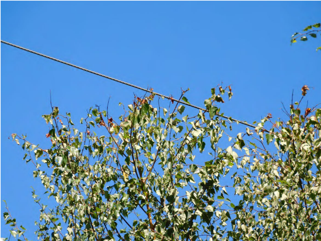
Probable violation B.356: Multiple trees show evidence of contacting primary conductors at 30945 SE Jackson Road, Gresham. (45.4739, -122.3451)
