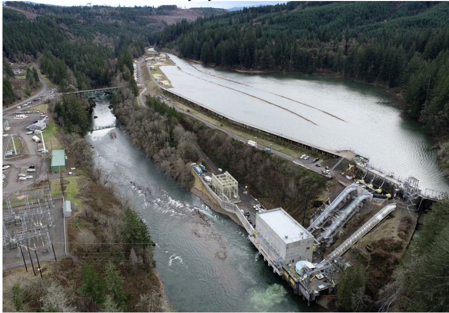
Figure 6 Faraday Hydroelectric Plant
