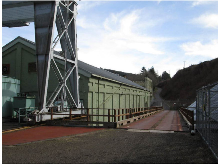
Figure 3 Faraday Units 1-5 and 6 Powerhouse
