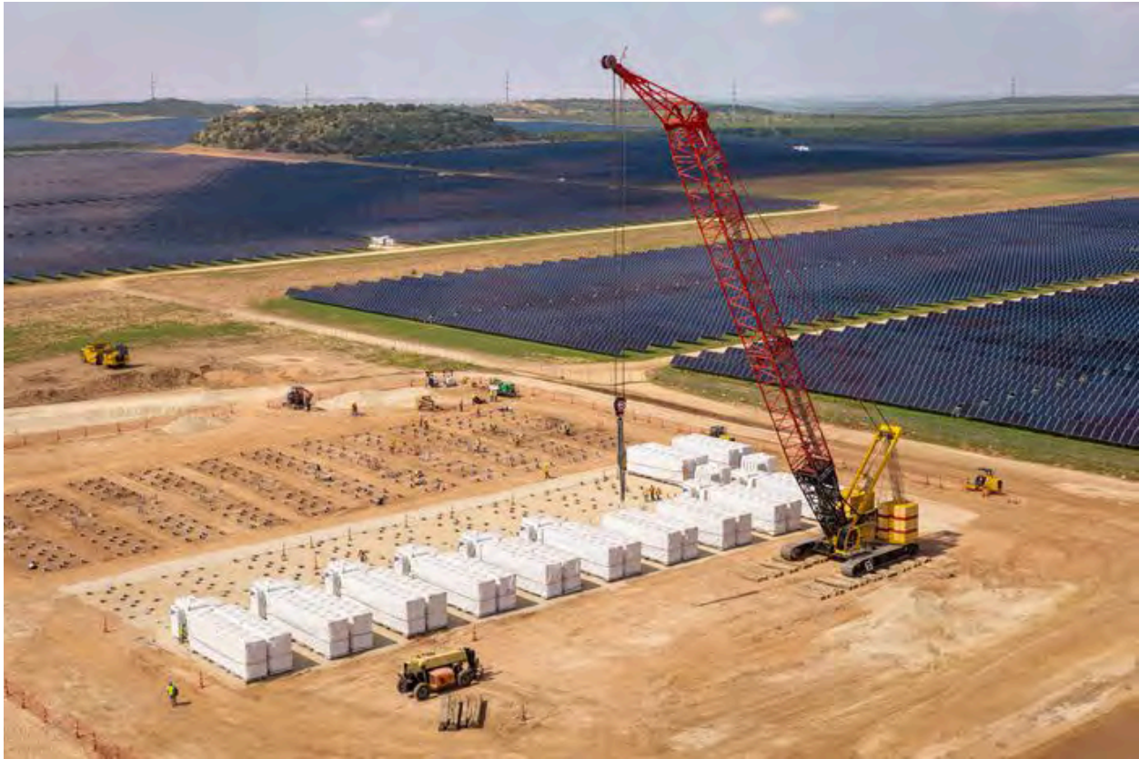
Intersect Power is installing Tesla Megapack batteries to store and dispatch electricity in Scurry County, TX.
