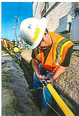
Aldyl A Natural Gas Pipe Replacement
