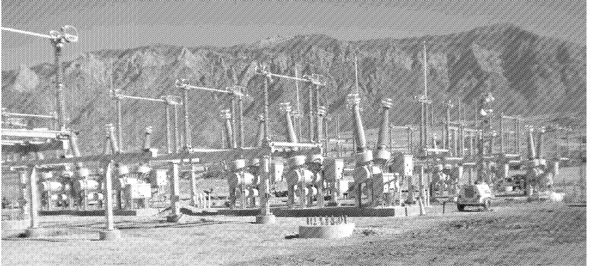
Populus substation— 345kV circuit breakers
