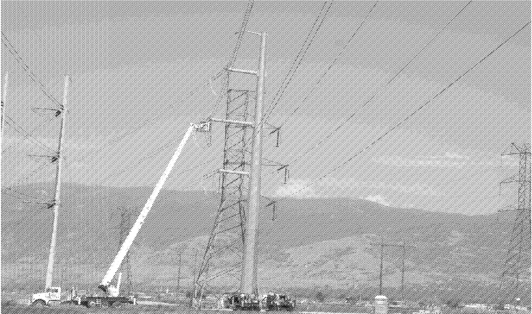
Angle Structure Installation
