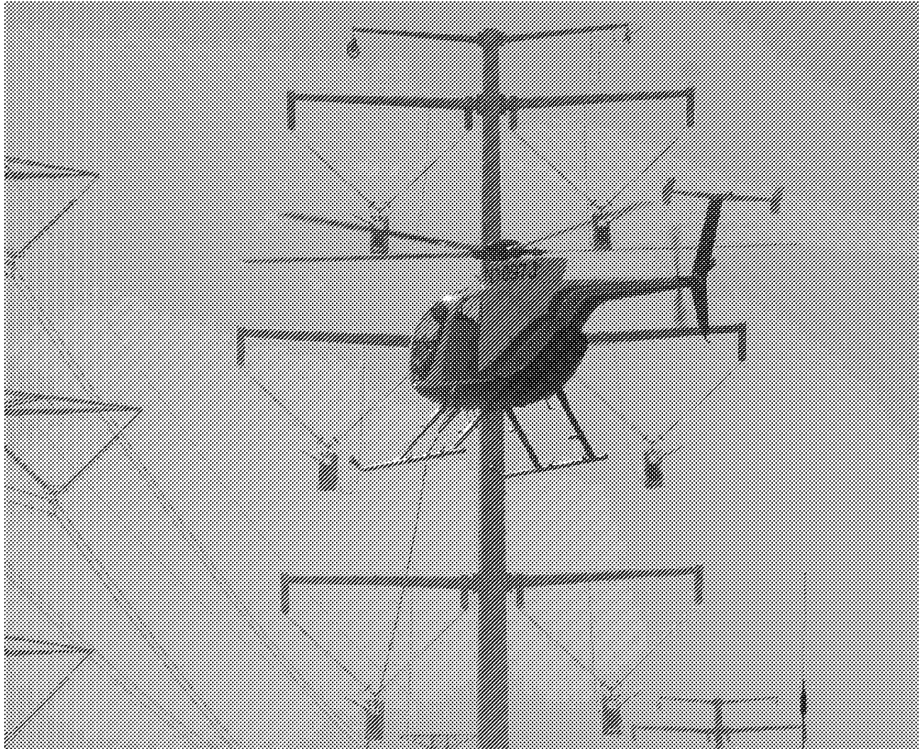
Stringing Optical Ground Wire
